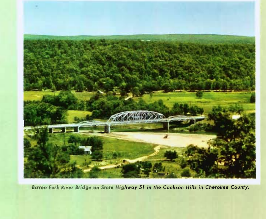
Barron Fork River Bridge on State Highway 51 in the Cookson Hills in Cherokee County.
