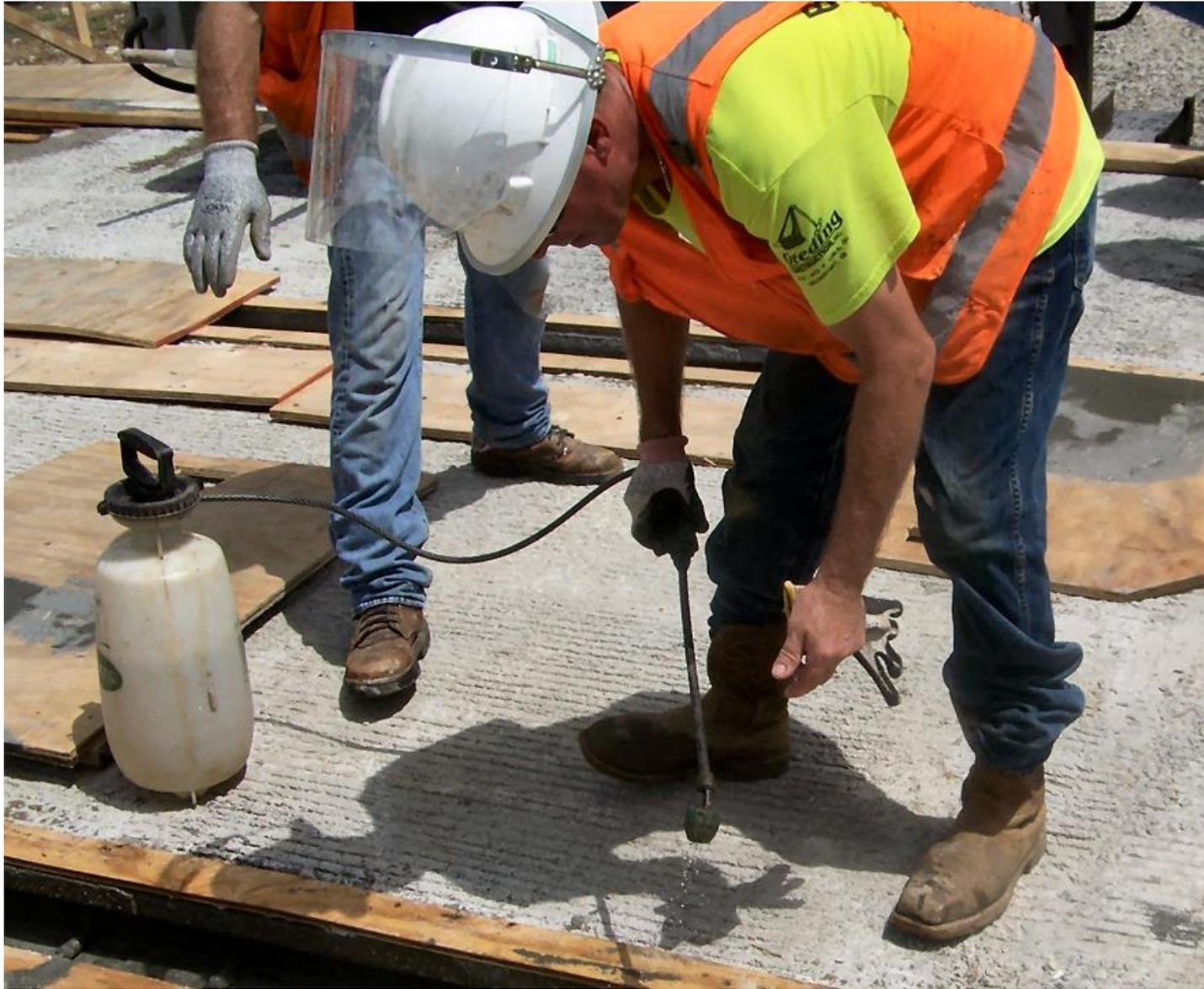
**Hand pump sprayer was identified as a better alternative to the water hose sprayer to keep surfaces SSD.**
