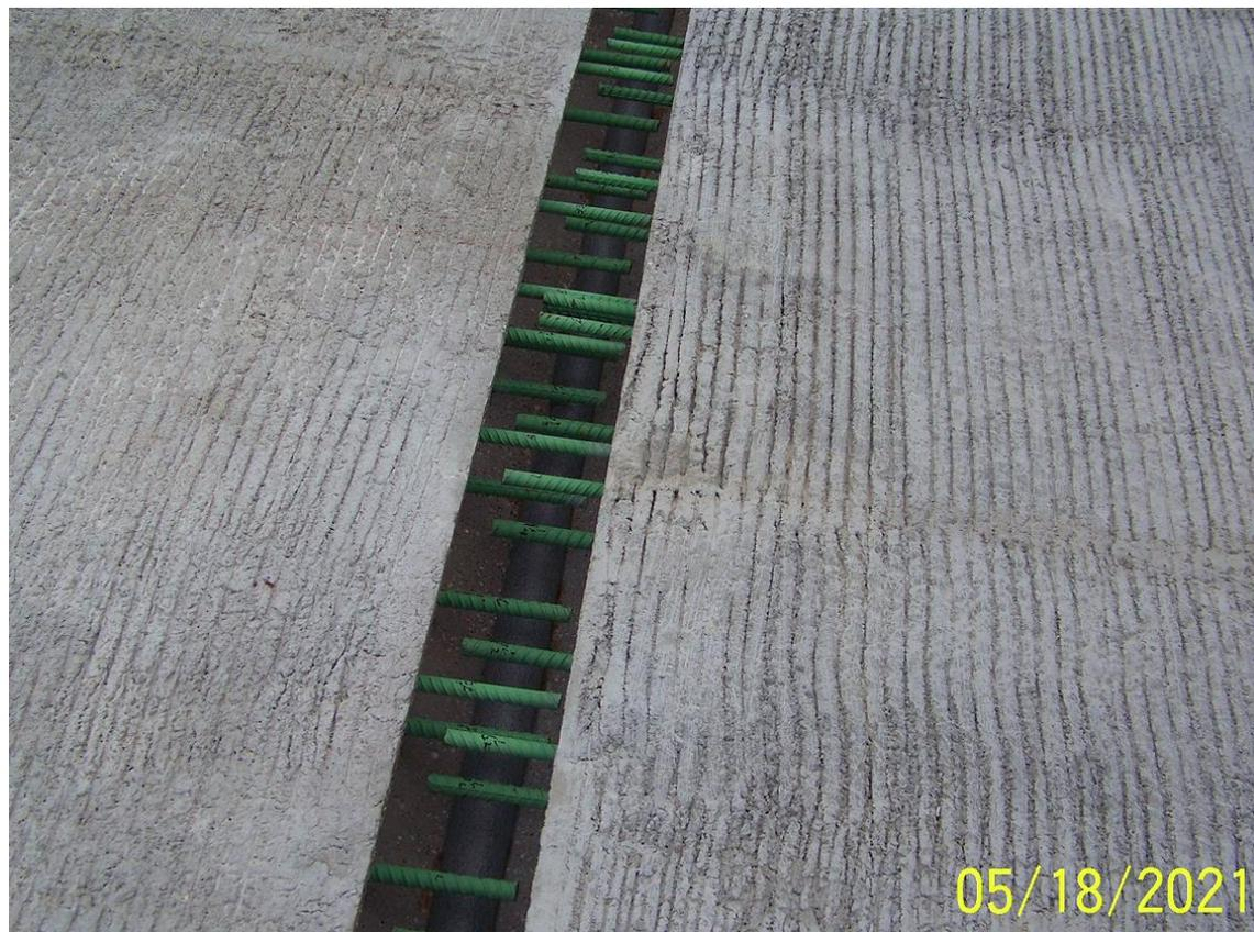
**Joint Opening prior to placing the UHPC – note the non-contact splice bars.**
