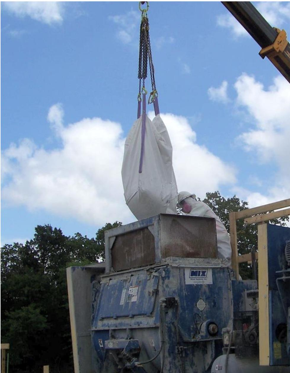
**Ductal® JS1000 - sacks premixed in pre-weighed supersacks of 2400 lbs. Steel fibers 2% by volume, and a high range water reducing admixture (HRWR). +/-25% of the required mixing water was added as ice since the ambient temperature that day was in excess of 80 °F.**
