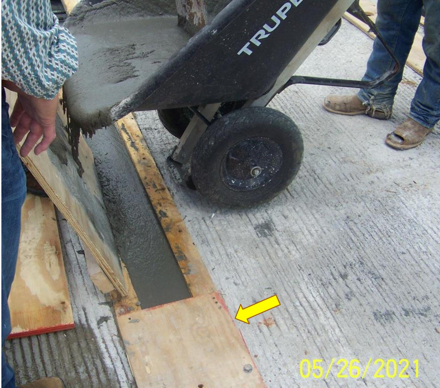
**UHPC must be top formed to prevent it from running out on the bridge deck.**
