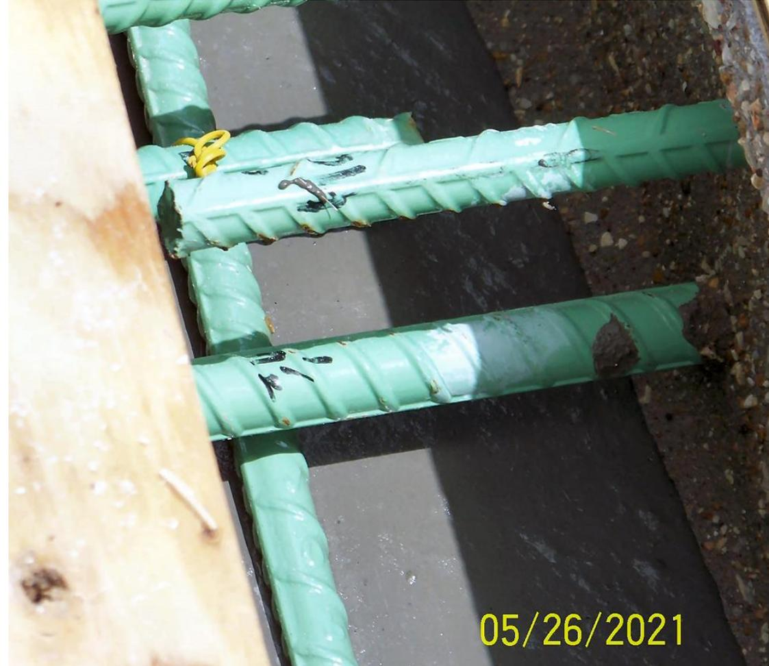
Note prior to placement of UHPC, surfaces must be “Surface Saturated Dry”. This can be a challenge on a hot windy day.
