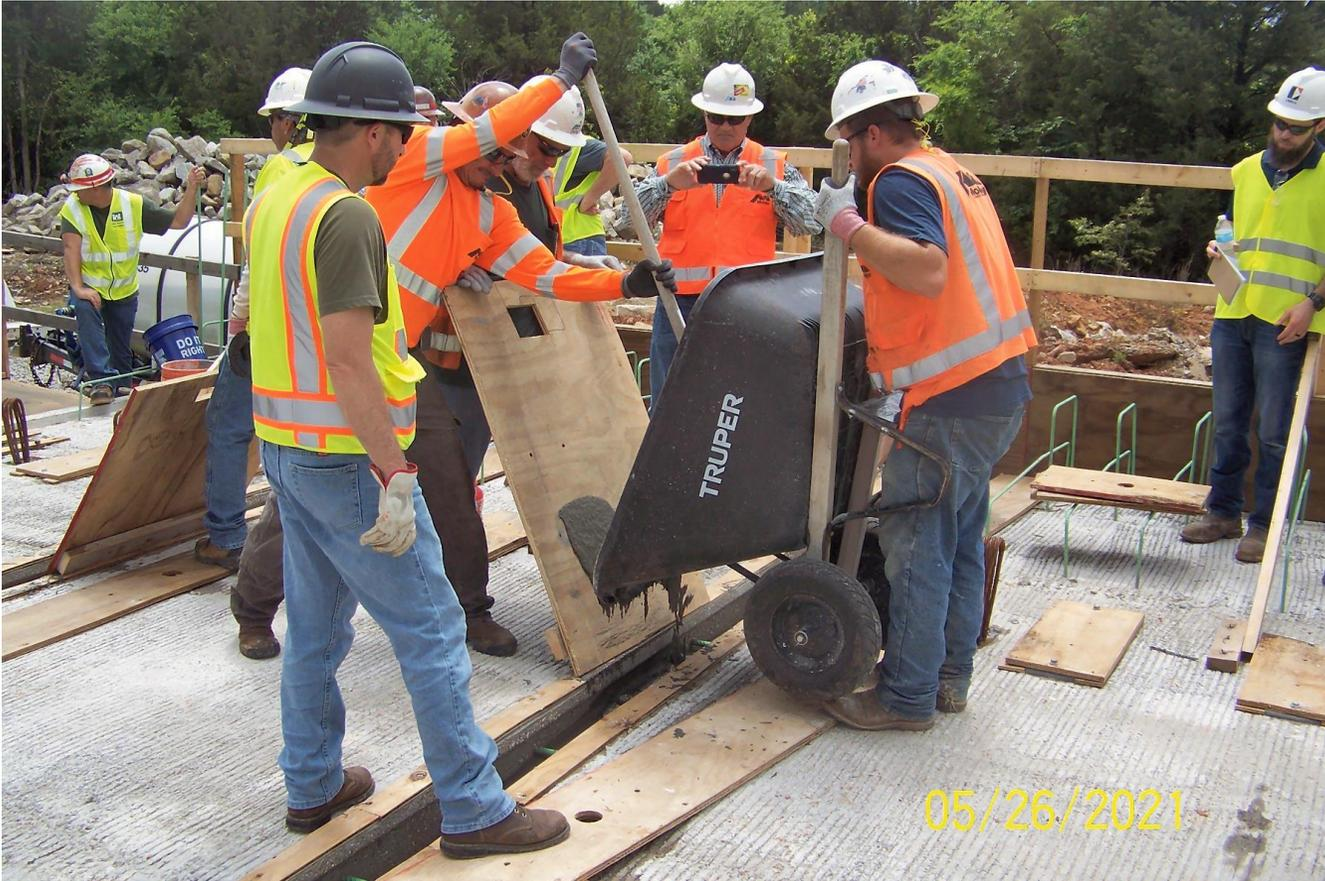
**Placing UHPC to connect precast panels.**
