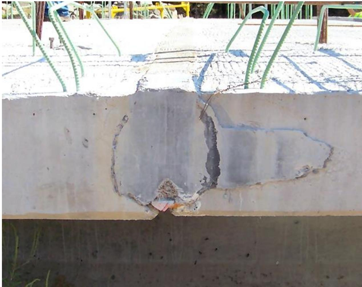
**UHPC Joint after Form Removal. Cores taken from the mock-up joints indicated excellent bond between the UHPC and the deck panel concrete.**
