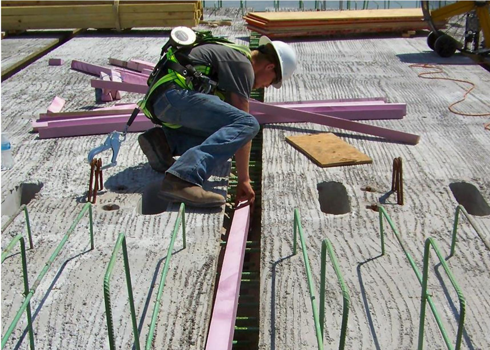
**Foam placement to seal joints form UHPC placement. Joints formwork was tested for watertightness by filling joints with water in advance of the UHPC placement.**
