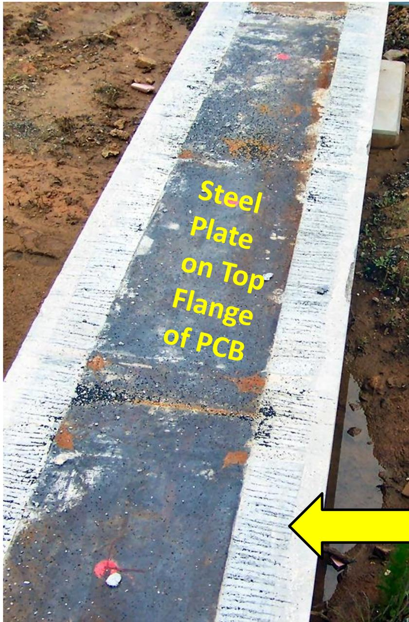
Looking down on the prestress beam note steel plate on the top of the beam. Studs will be welded to the steel plate.
