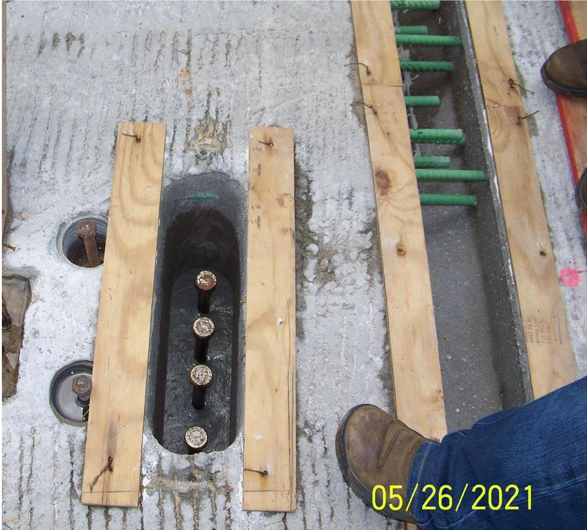
UHPC Flowing under panel and into openings for studs.
