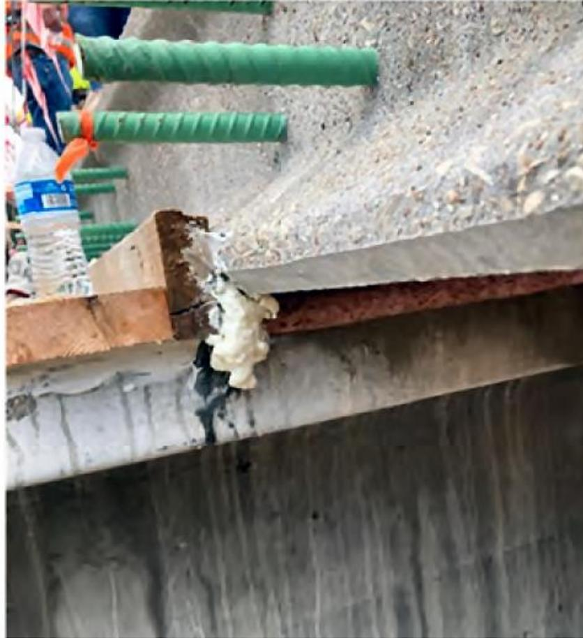
**The leak issues were resolved by the contractor applying additional spray foam and formwork bracing**
