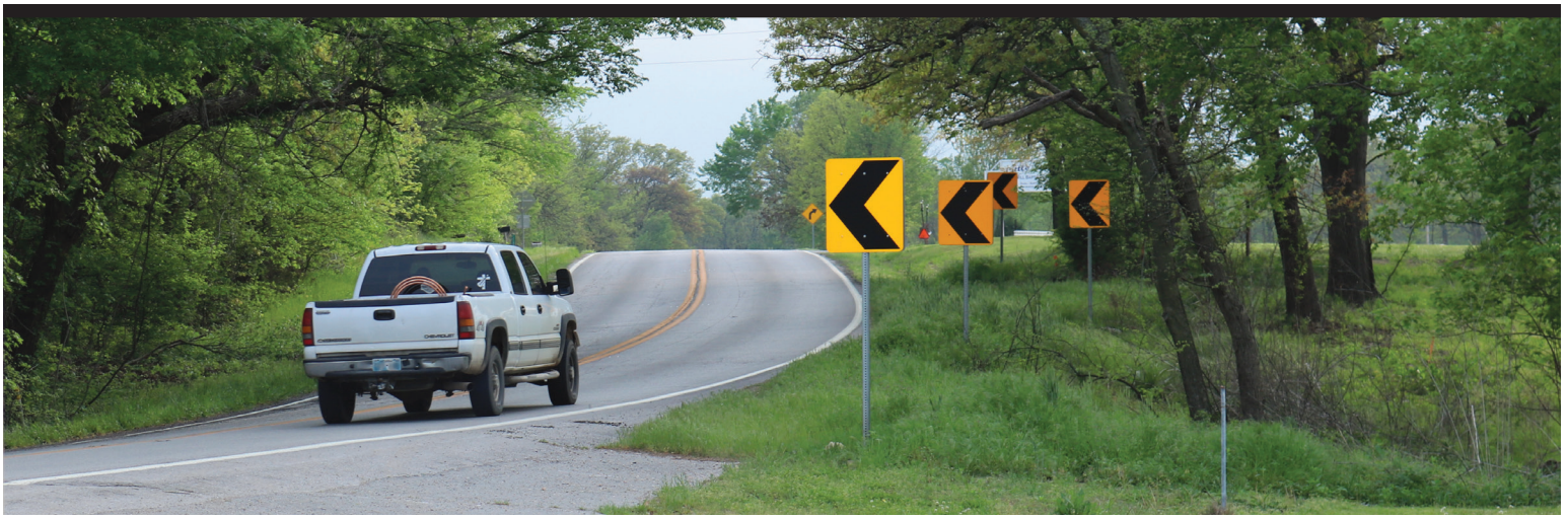
Above: A Fall 2018 application of HFST on SH-20 near Locust Grove, will reduce crashes, injuries and fatalities on this stretch of road in Mayes County. HFST will also be applied in Rogers, Sequoyah, LeFlore, Lincoln and Tulsa counties.
