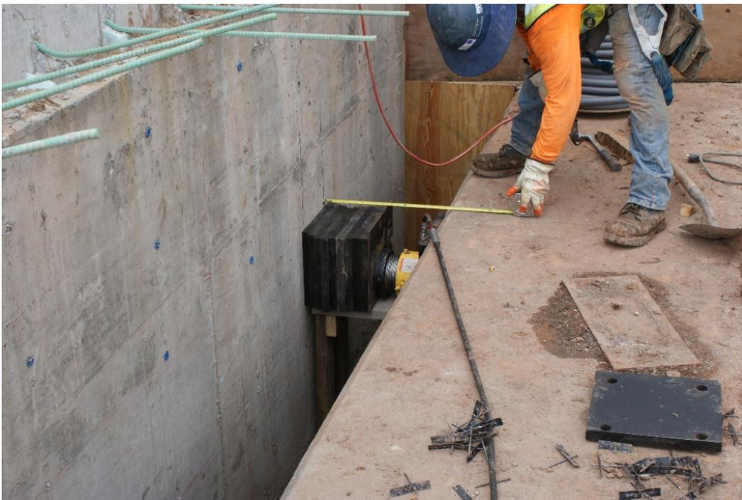
Figure 18. Photo. Air-operated jack placed between abutment and deck slab to provide adjustment between sections.
