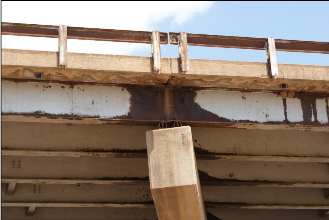
Figure 3. Photo. Deteriorated steel and support mechanisms on existing bridge.
