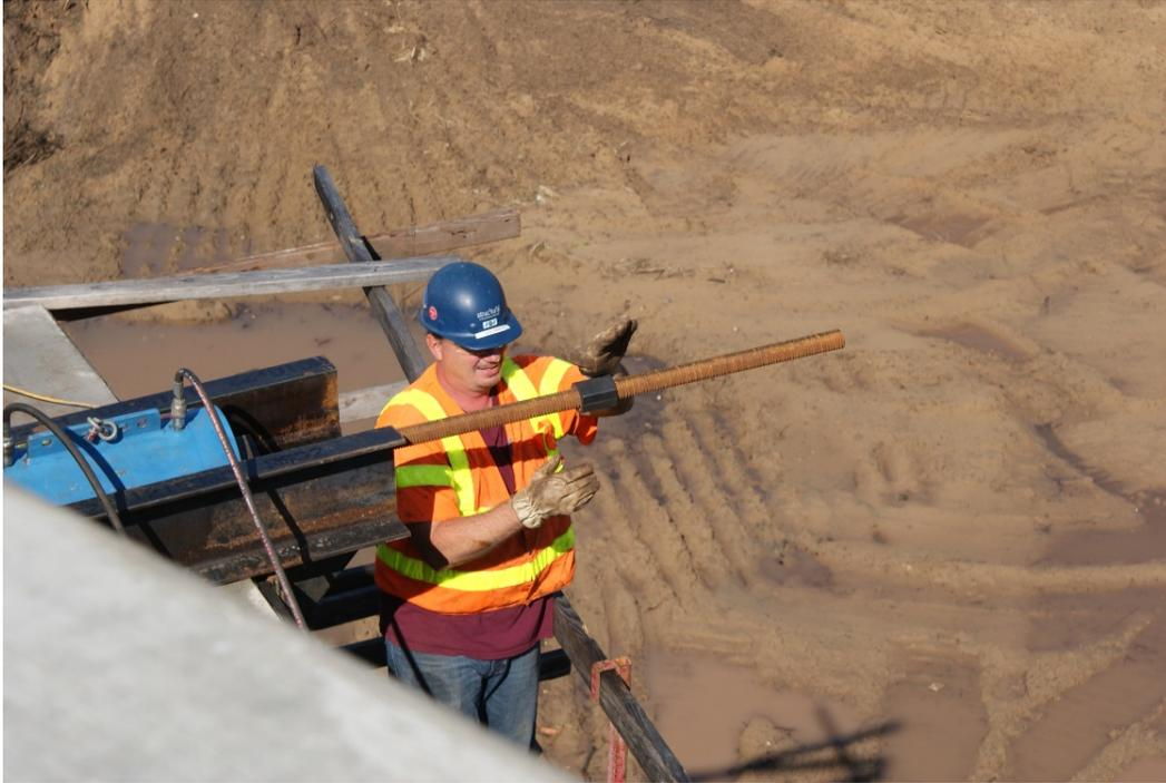
Figure 17. Photo. Threaded nut used to lock rod to ram prior to pull.
