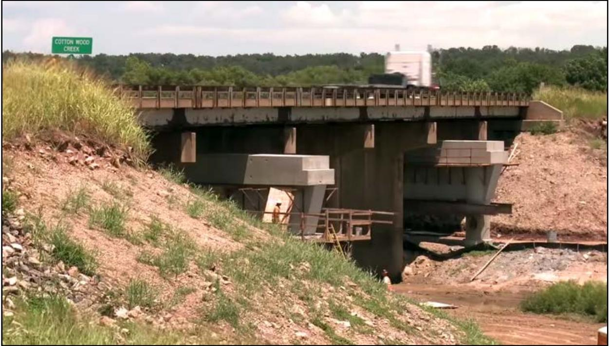
Figure 5. Photo. New piers and caps in place below and between existing piers.
