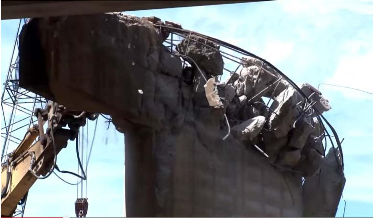
Figure 11. Photo. Removal of existing piers (courtesy: ODOT).
