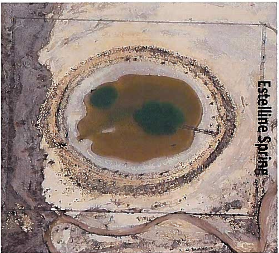
Aerial view of Estelline Springs project showing earthen ring dike surrounding the salt spring
