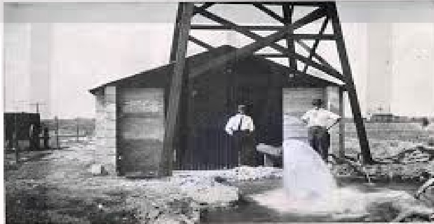
McDonald Irrigation Well, 1000 Gallons per Minute, Hereford, Texas.
