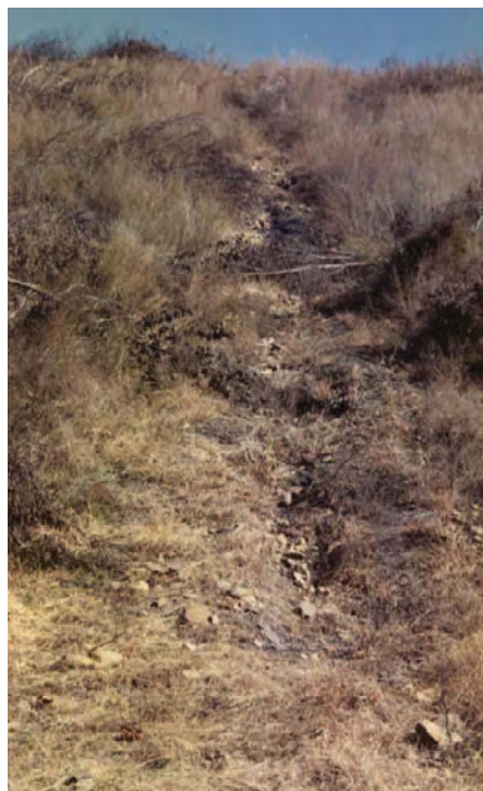
Erosion of dam embankment
