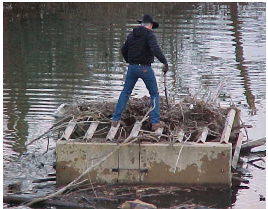
Trash Rack With Debris
