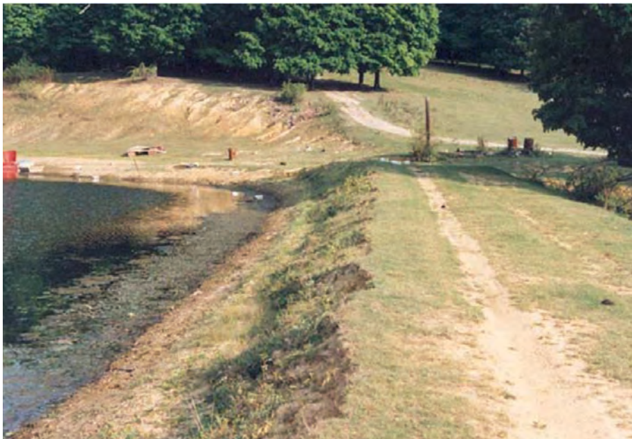
Wave erosion on upstream slope of dam.
