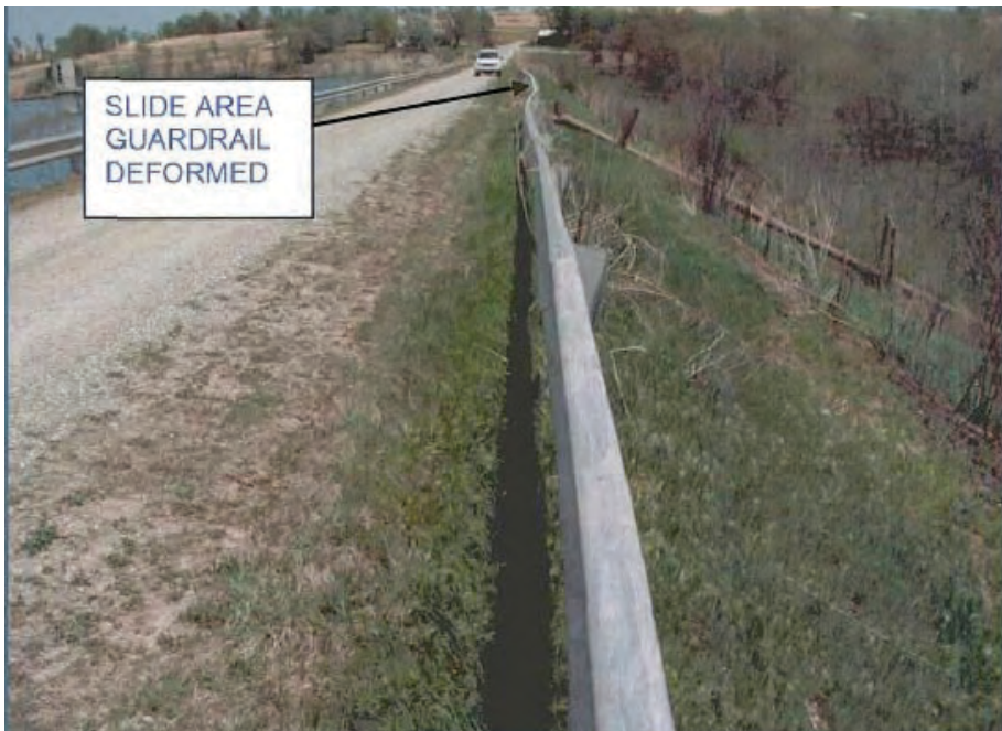
Embankment slide moves guardrail
