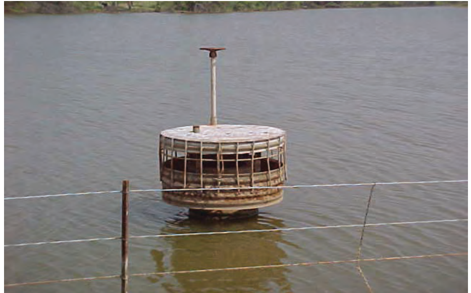
Trash Rack Over Inlet Pipe
