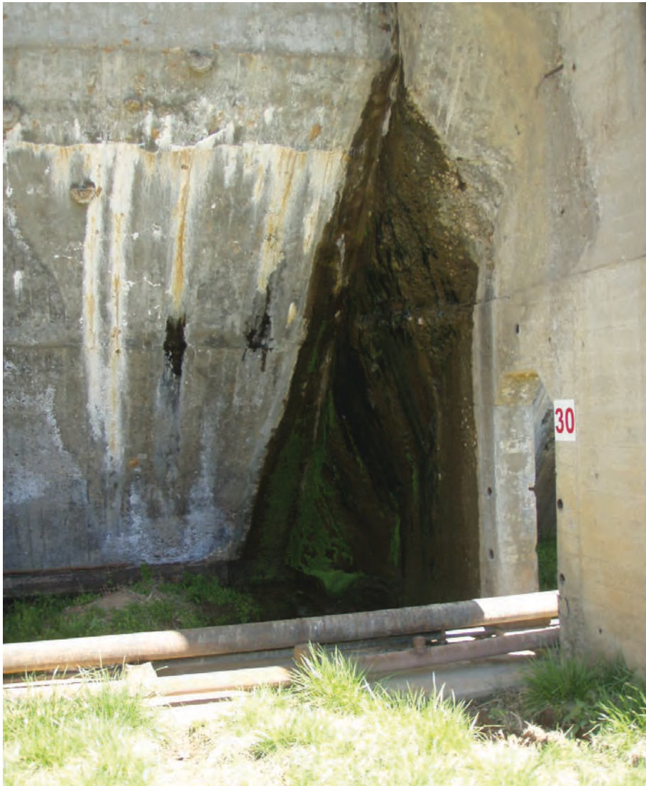
Vertical crack in dam allowing seepage
