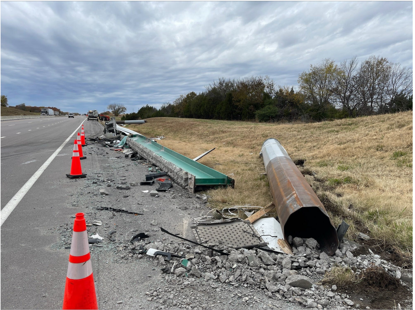
The damaged bridge beam is shown Nov. 9 lying on the shoulder of westbound I-44/Turner Turnpike at Stroud next to other debris from the bridge as well as large pipes knocked loose from the top of the illegal, over-height semi-tractor trailer load after it hit the bridge about 11 p.m. Nov. 8.
