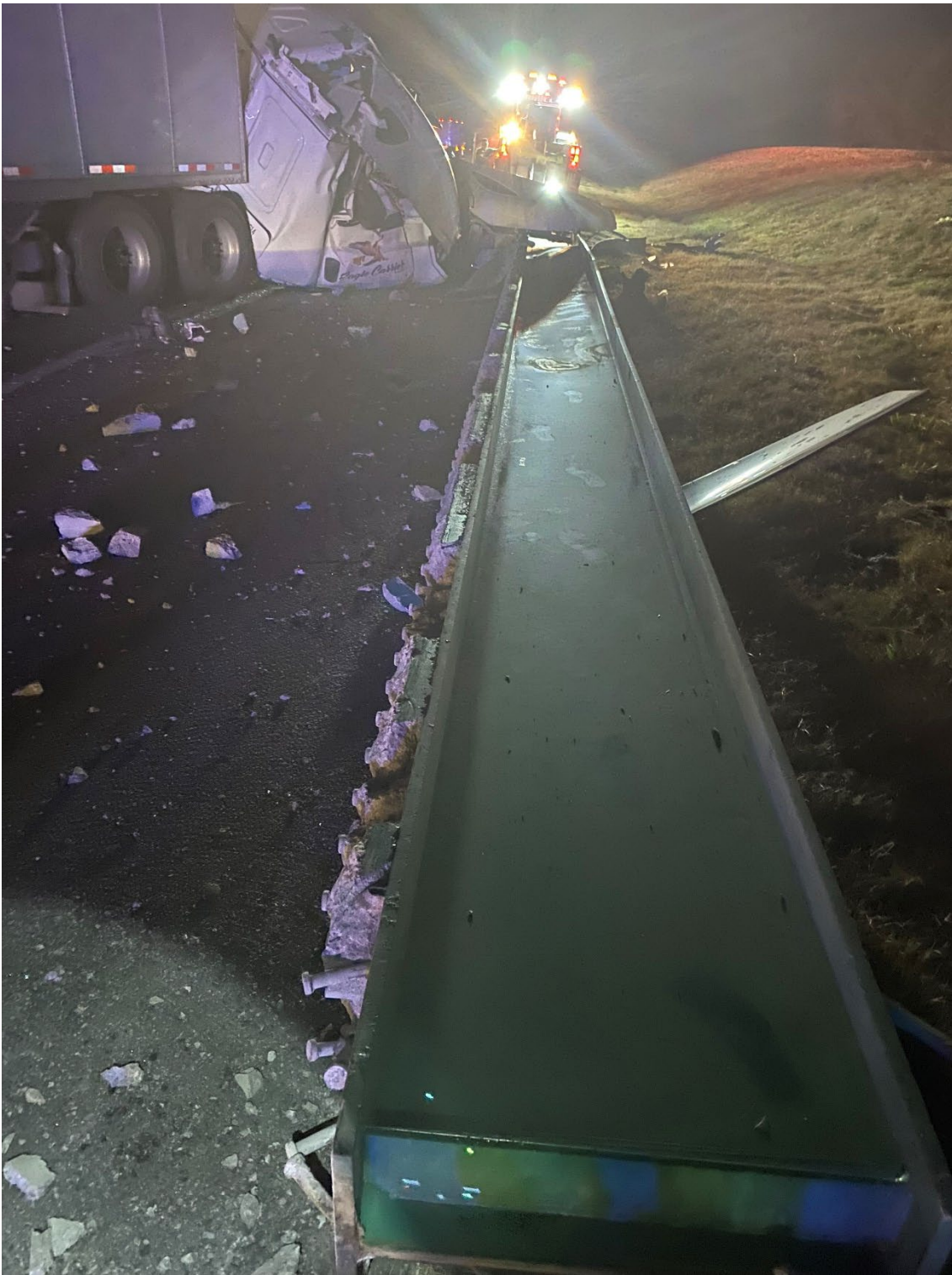
Taken shortly after the crash Wednesday night on westbound I-44/Turner Turnpike at Stroud, this shows the second vehicle that was impacted by the falling bridge beam after an illegal, over-height semi-truck traveling just ahead of this vehicle hit the bridge, causing extensive damage.
