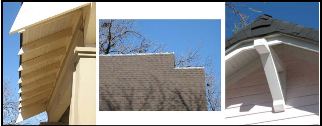
FIGURE 36: PRESERVE ORIGINAL ROOF FEATURES, SUCH AS EXPOSED RAFTER TAILS, RIDGE TILES AND SUPPORT BRACKETS.
