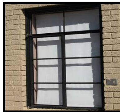
FIGURE 32: STEEL CASEMENT WINDOWS MAY BE REPLACED IN-KIND, IF NECESSARY.
