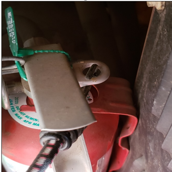
Trash Can Bungee Attached to Fire Extinguisher
