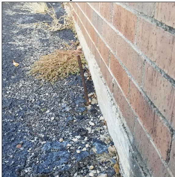
Exposed Rebar
