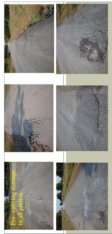
Not eligible - Damage attributed poor condition of road prior to the event as evidenced by potholes, edge deterioration, cracking, alligator cracks, and numerous patches in the chip and seal surface.
