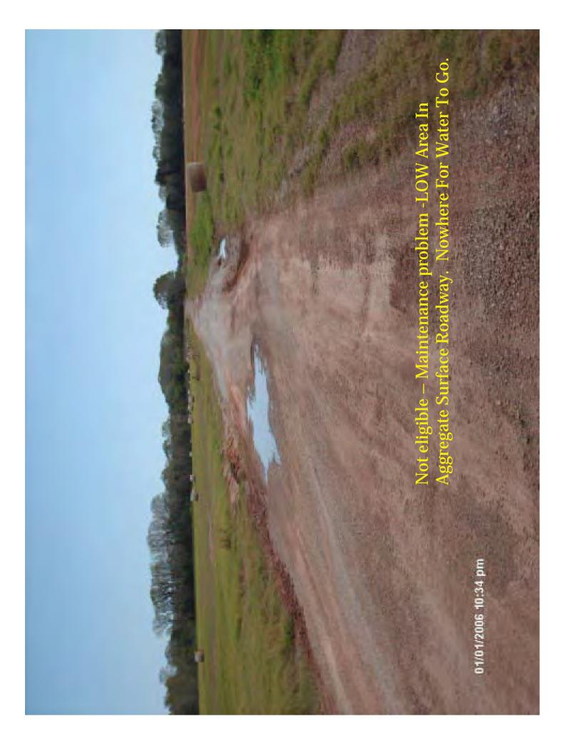
Sub-G ade. Replace Destroyed Aggregate Surface. No More Than 3", Looks Like Applicant Lost No More Than 2" Thickness **Gligible – Haul to Embankment And Build** Aggregate.
