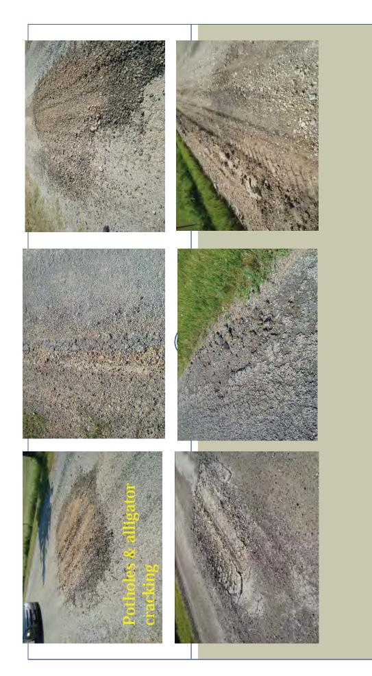
Not eligible - Chip and seal roadway surface has considerable alligator cracking and potholes. The roads have considerable alligator cracking well beyond the damaged locations.
