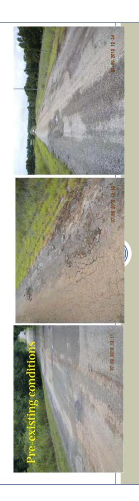
Ineligible. Normal deterioration such as "alligator cracking" are not eligible as it is pre disaster damage.
