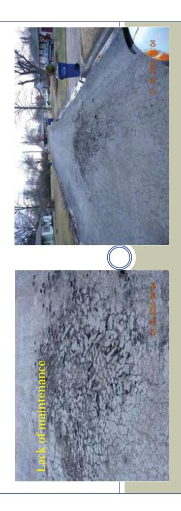
Not eligible - Damages ineligible per FEMA 322 page 33, based on the lack of maintenance at the sites, pre-existing damage: potholes alligator cracking.
