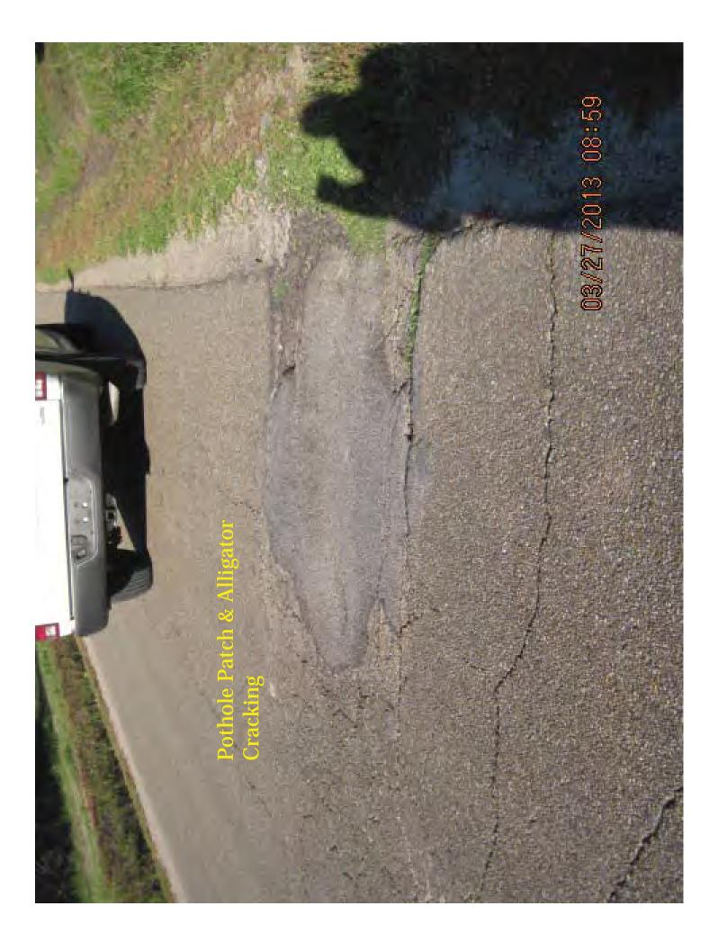
Not eligible - Base & Sub-Grade Failure. Usually Caused by Not Enough Depth Of Base.
