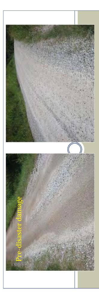
patches and alligator cracking along the road leading to the damage site indicating deferred maintenance. Not eligible - Damage not storm related due to numerous
