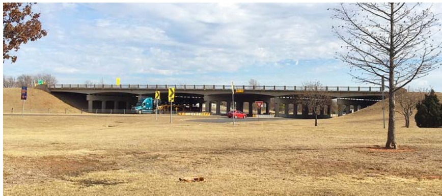
Photo 7: View facing eastward towards Douglas Blvd Bridge.
