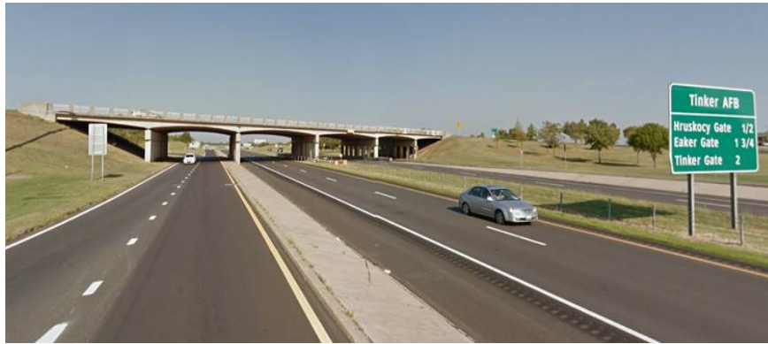
Photo 5: View from I-40 facing westward towards Douglas Blvd Bridge.
