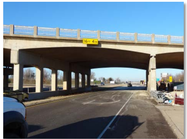
Figure 2: Substandard Truck Clearance under I-40 on Anderson Road
