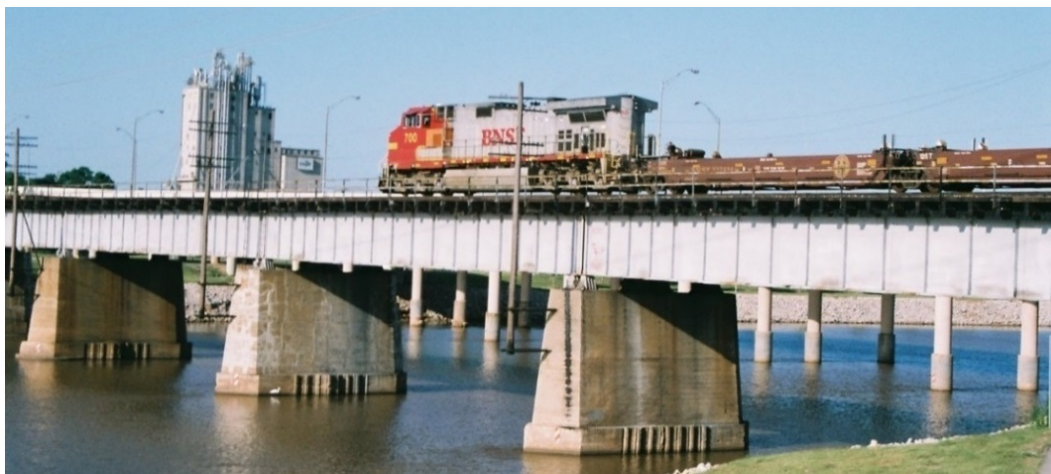
BNSF bridge over the Oklahoma River, south of downtown Oklahoma City
