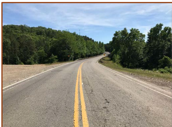
Figure 10. U.S. 259 North of Stevens Gap Road
