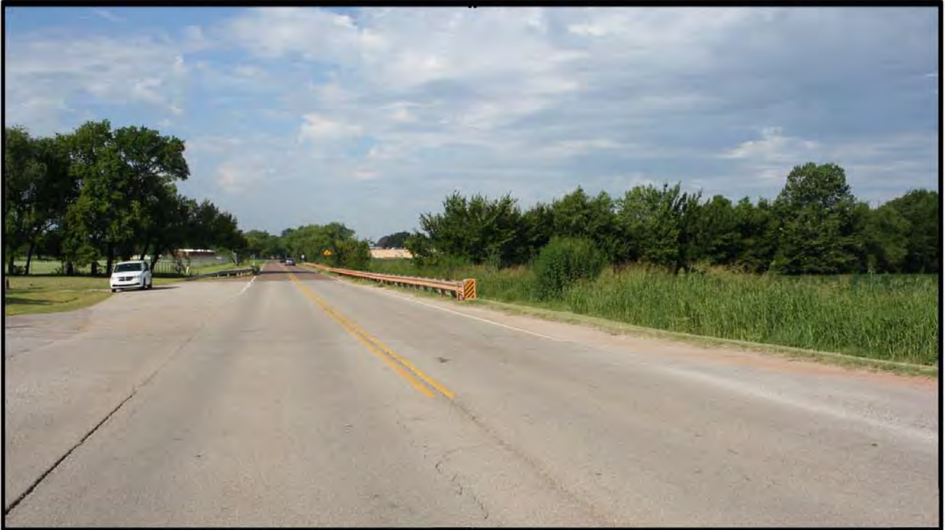
State Highway 66 Roadbed in Arcadia and vicinity Oklahoma County, Arcadia, Oklahoma Intersection of State Highway 66 and Anderson Rd. Anna Eddings--ODOT Cultural Resources Program
