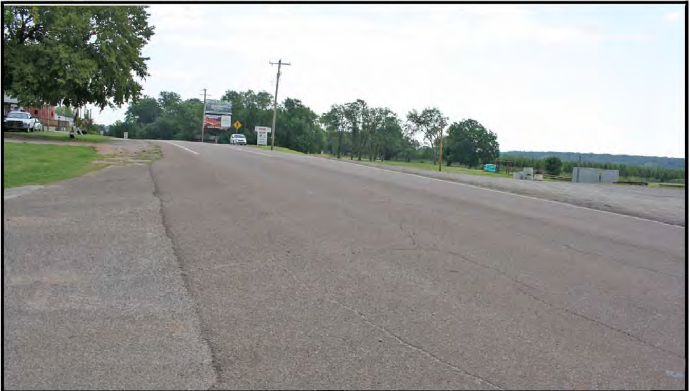
State Highway 66 Roadbed in Arcadia and vicinity Oklahoma County, Arcadia, Oklahoma Intersection of State Highway 66 and Division St. Anna Eddings--ODOT Cultural Resources Program
