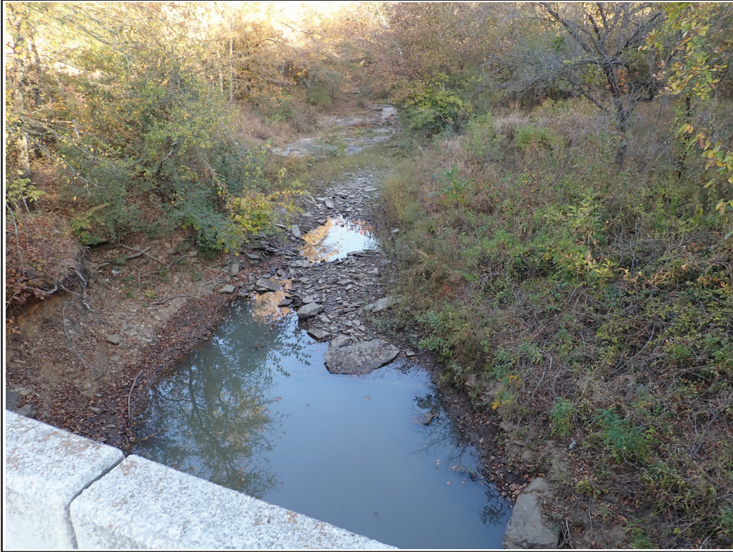
Photo 3 - On bridge looking north, upstream
