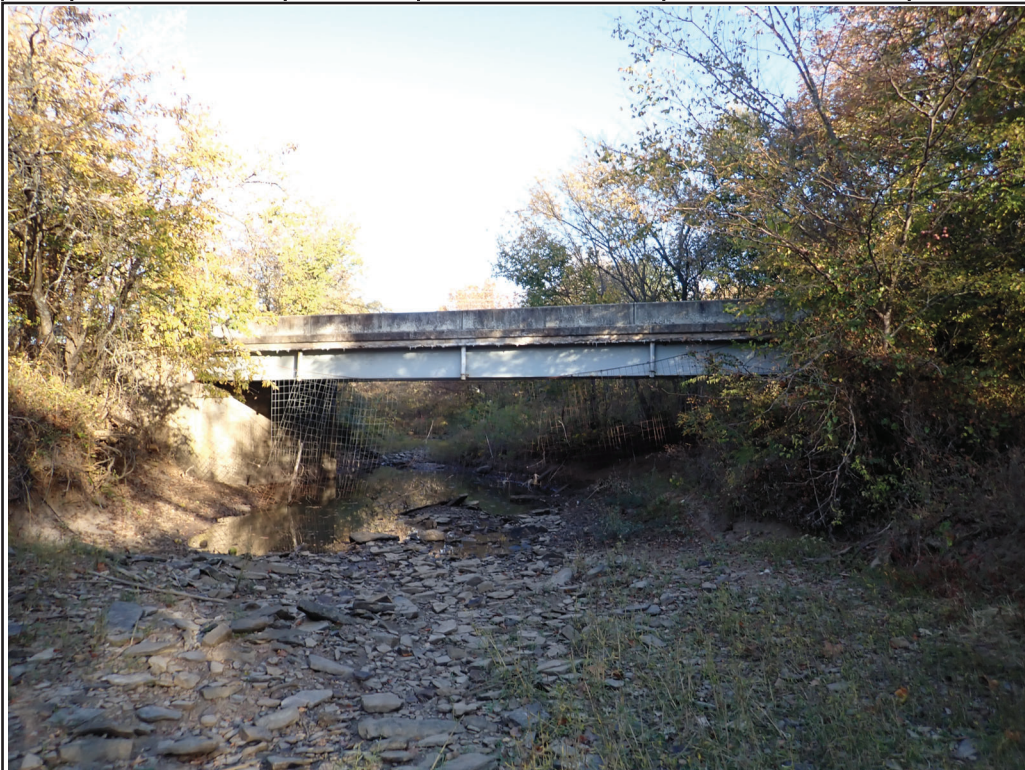
Photo 2 - South elevation, looking upstream
