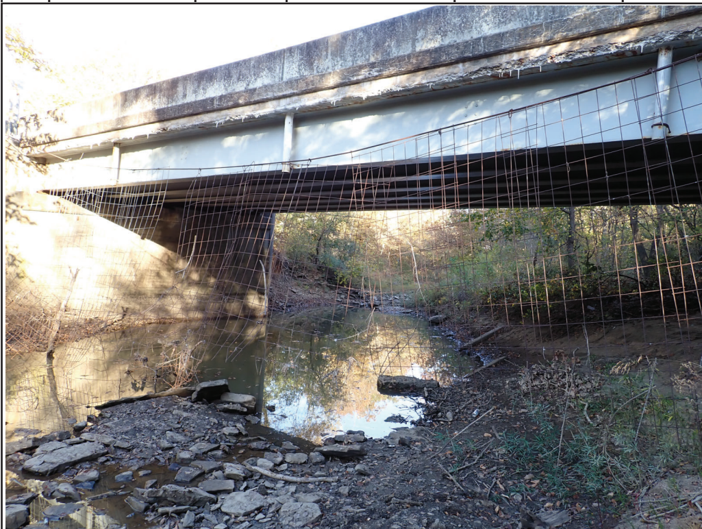
Photo 10 - South channel; cattle fence installed
