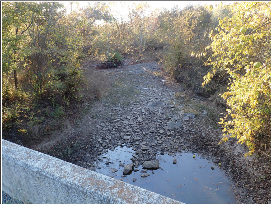
Photo 4 - On bridge looking south, downstream
