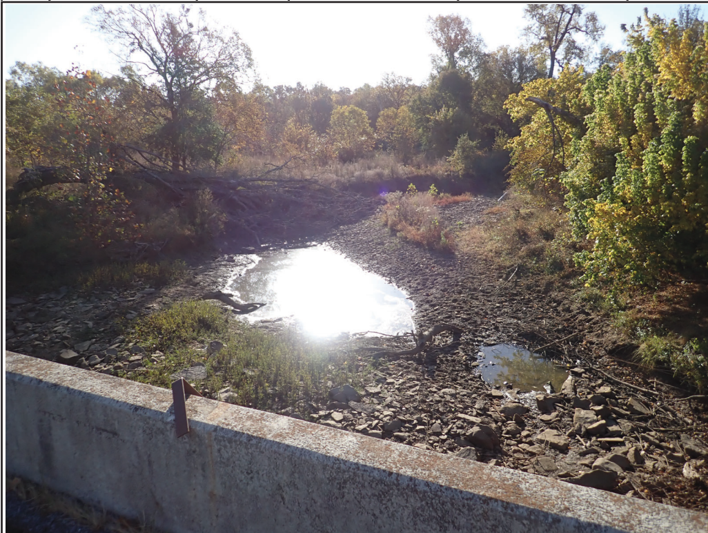
Photo 4 - On culvert looking south, downstream
