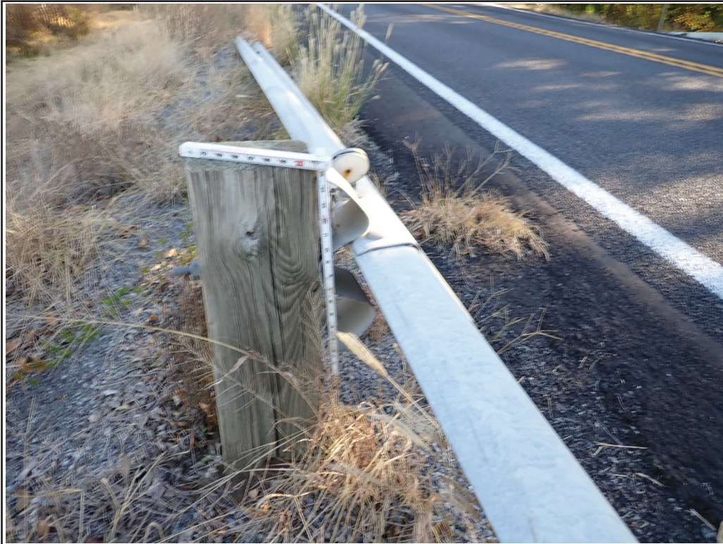
Photo 5 - Northeast approach guardrail; detached from posts
