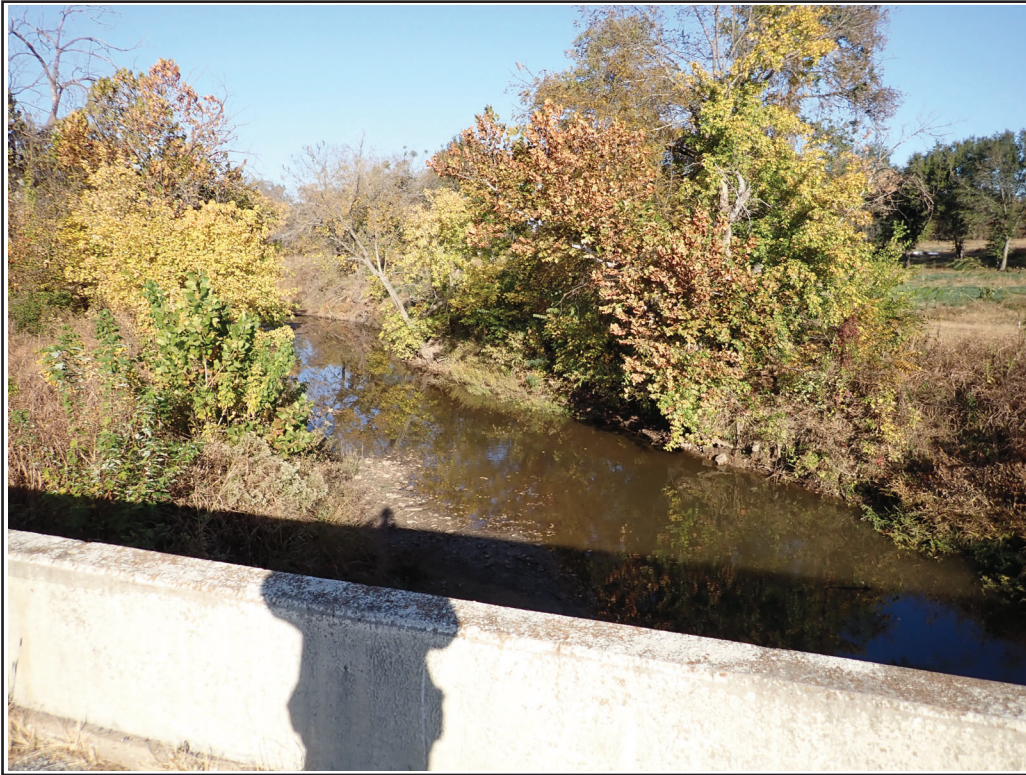
Photo 3 - On culvert looking north, upstream
