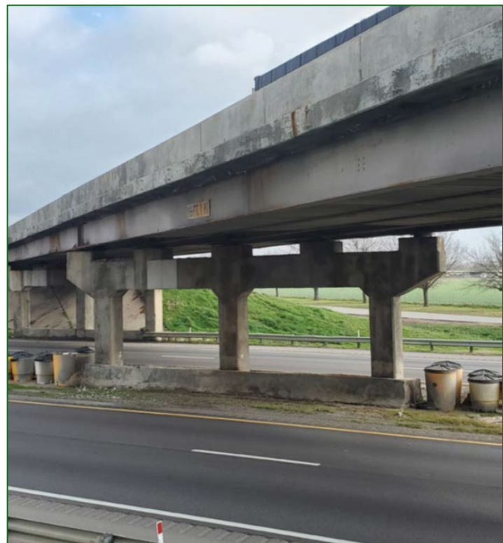
Figure 2. SH-74 Bridge over I-35
