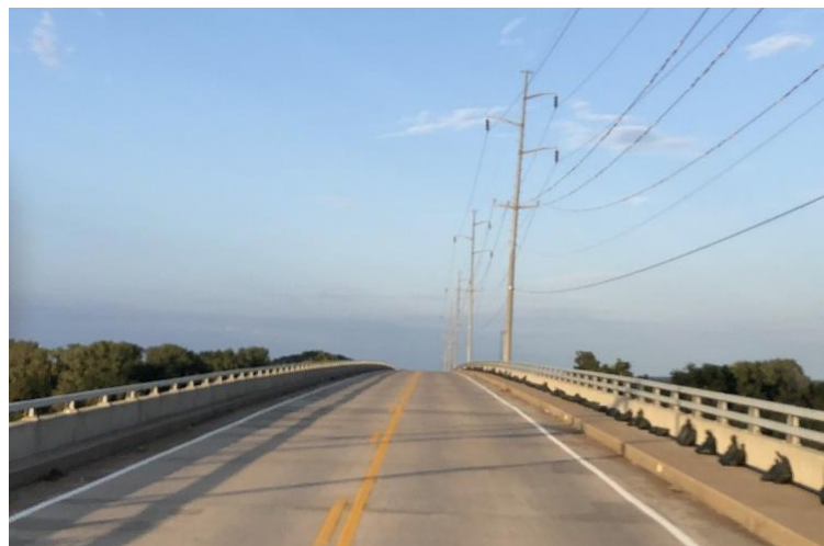
Figure 7: Existing bridge, facing west
