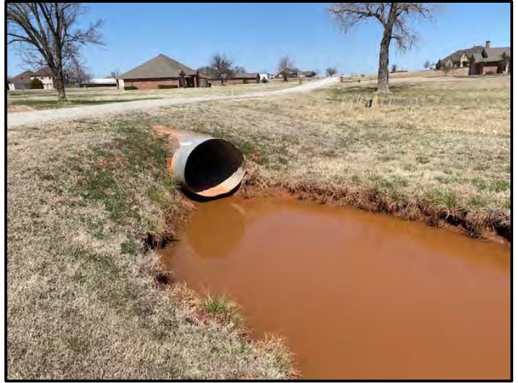
Photograph 19: Structure 5 at R4SBC-04, no migratory bird nests present.
