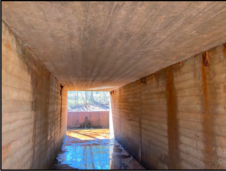
Photograph 12: Beneath Structure 2, barn swallow nest.
