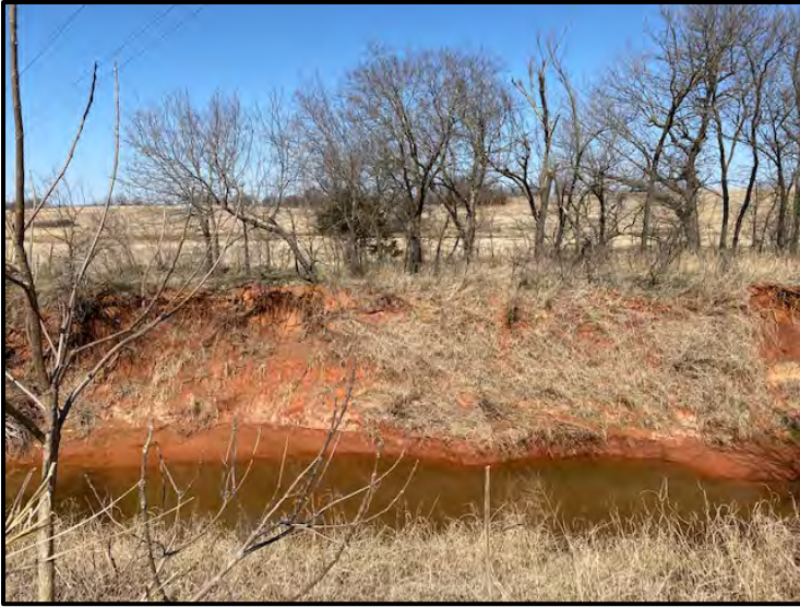
Photograph 6: Steeply sloped bank of R2UBHx-01 (Captain Creek).
