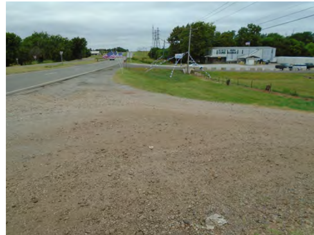
Image 8 (PS 4): looking NW from the northside of the SH-66 westbound lanes.
