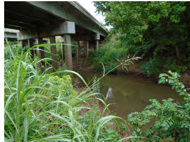
Image 12 (PS 7): looking N at Shell Creek.
