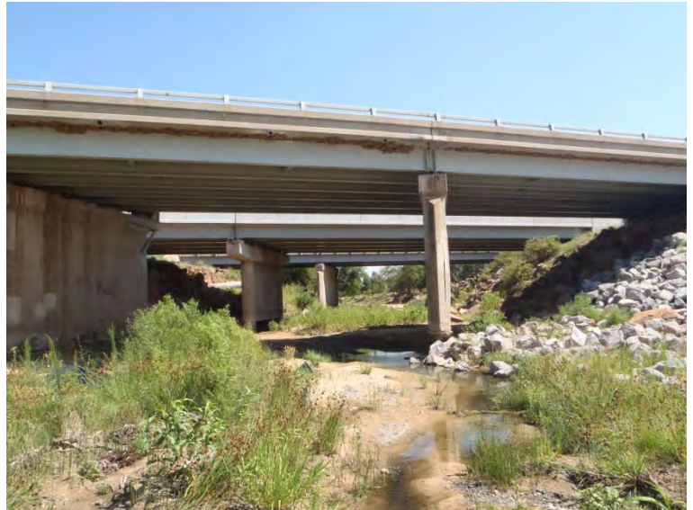
Photograph 4: Facing north along FS-1 toward east-bound I-40 bridge.
