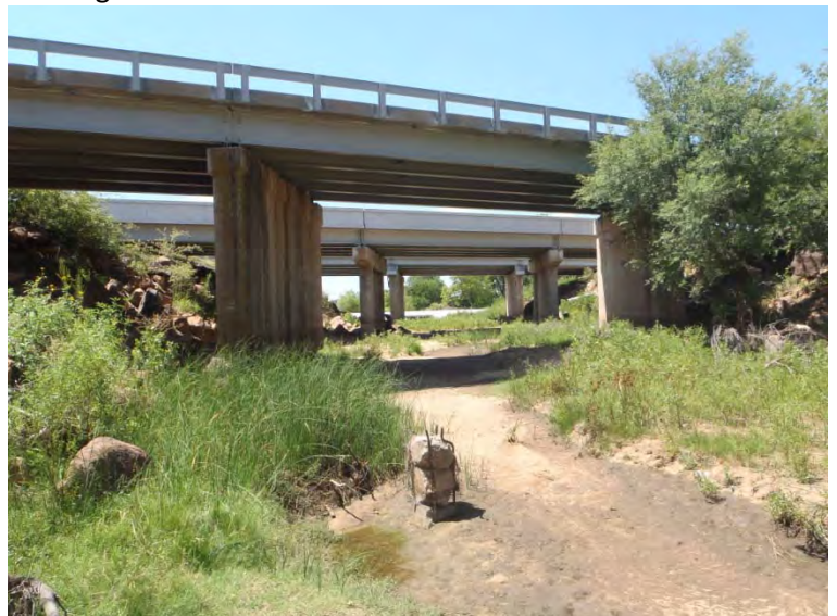
Photograph 6: Facing south along FS-1 toward north service road bride.
