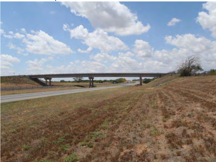
Photograph 11: Facing east along I-40 near eastern edge of Turkey Creek study area.
