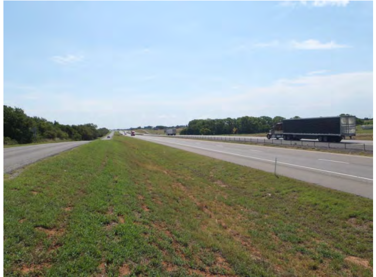
Photograph 8: Facing east along I-40 near western edge of Sand Creek study area.
