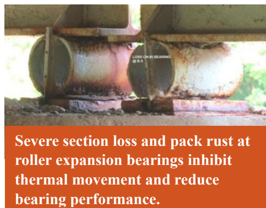
Figure 4: NBI #12629 Condition
