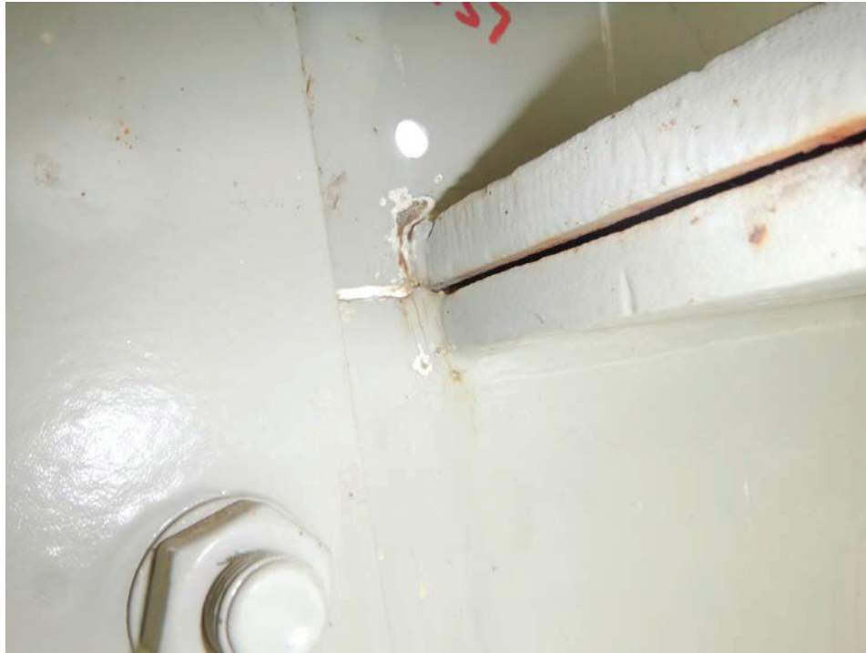
Photograph 9 - Looking southwest at girder 1, span 7 at the termination of the horizontal splice near floor beam 4. Note: paint cracks up to 1 inch long at the top plate and 1 1/8 inches long at the bottom plate. No change from 2017 inspection.
