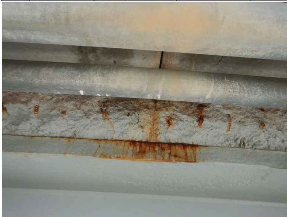
Photograph 4 - Looking north at the underside of the south overhang at floor beam 6, span 6. Note: spalling of the deck and corrosion of girder 1 due to deck drainage ponding on the sidewalk.
