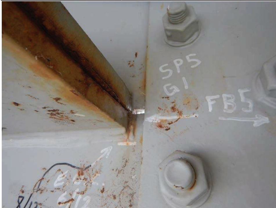
Photograph 6 - Looking southeast at girder 1, span 5 at the termination of the horizontal splice near floor beam 5. Note: no change to previously noted crack.
