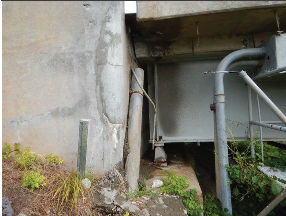
Photograph 23 - Looking north at the west abutment. Note: backwall has rotated east 1 1/8 inches over 4 feet.
