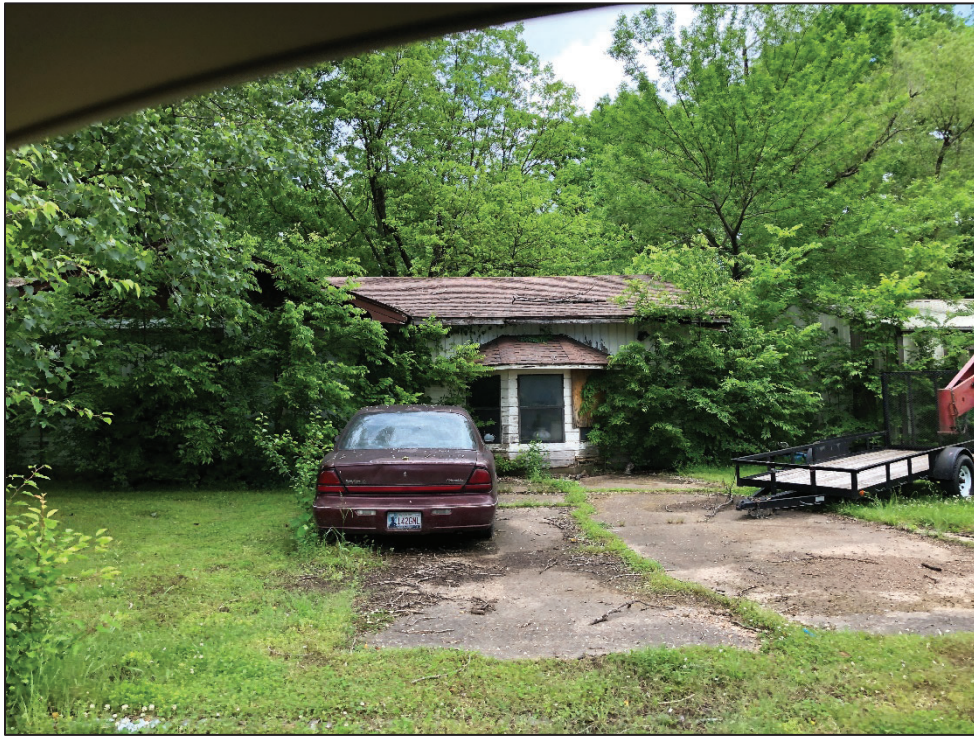
Photo 33: Home in disrepair in the study area.
