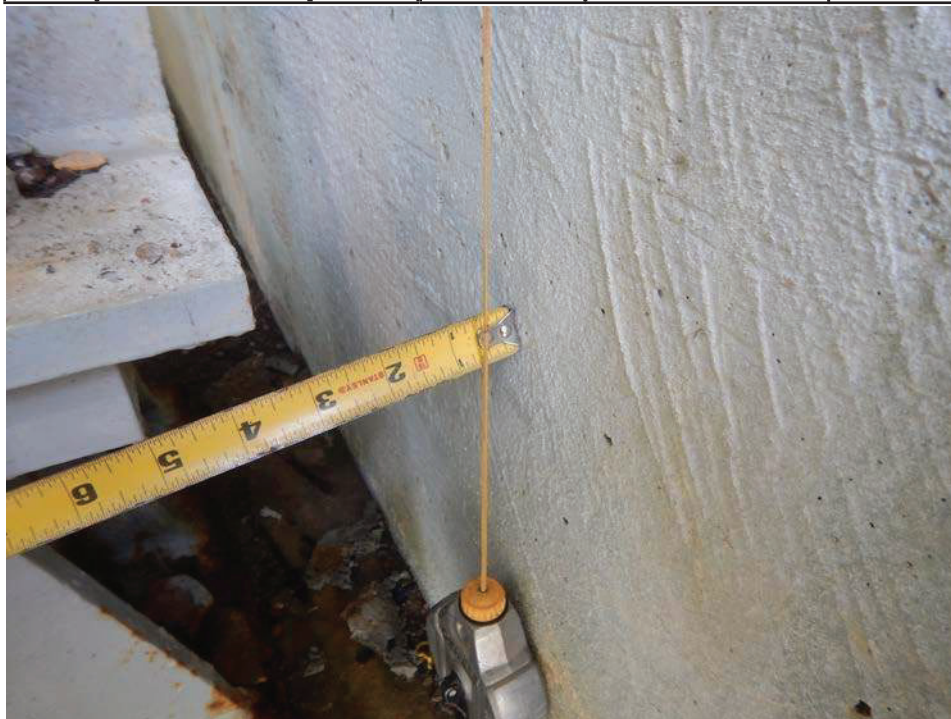
Photograph 24 - Looking north at the east abutment backwall at girder 1. Note: backwall is leaning 11/16 inch over 4 feet.
