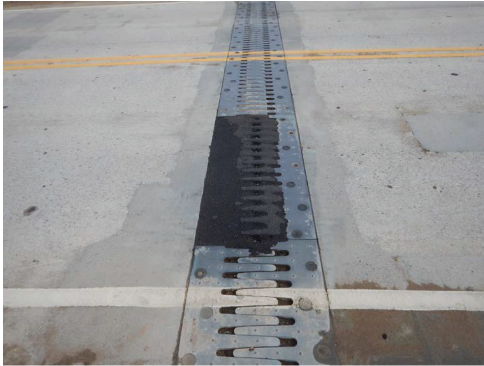
Photograph 5 - Looking north along the finger expansion joint at pier 4. Note: 5-foot section of the finger joint has been repaired with an asphalt patch.
