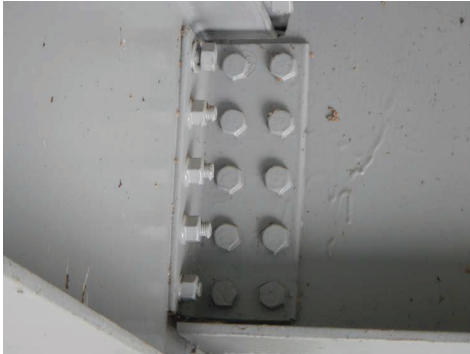
Photograph 17 - Looking north at the stringer 2 connection to floor beam 3 in span 6. Note: 1 loose bolt in connection to the floor beam.
