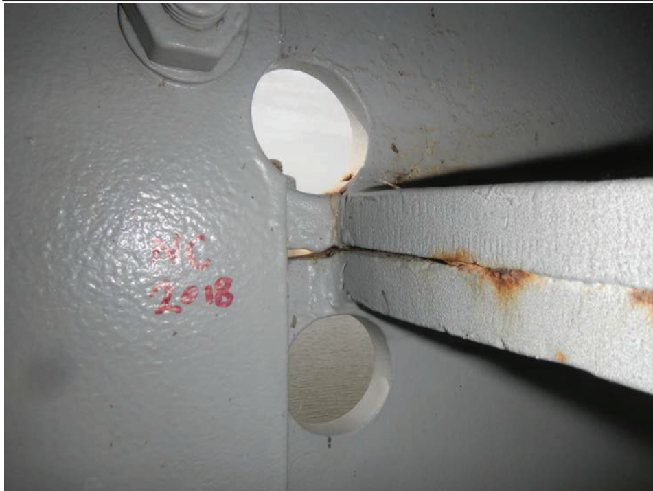
Photograph 8 - Looking southwest at girder 1, span 6 at the termination of the horizontal splice near floor beam 3. Note: 3/4-inch long crack arrested with drilled hole retrofits.
