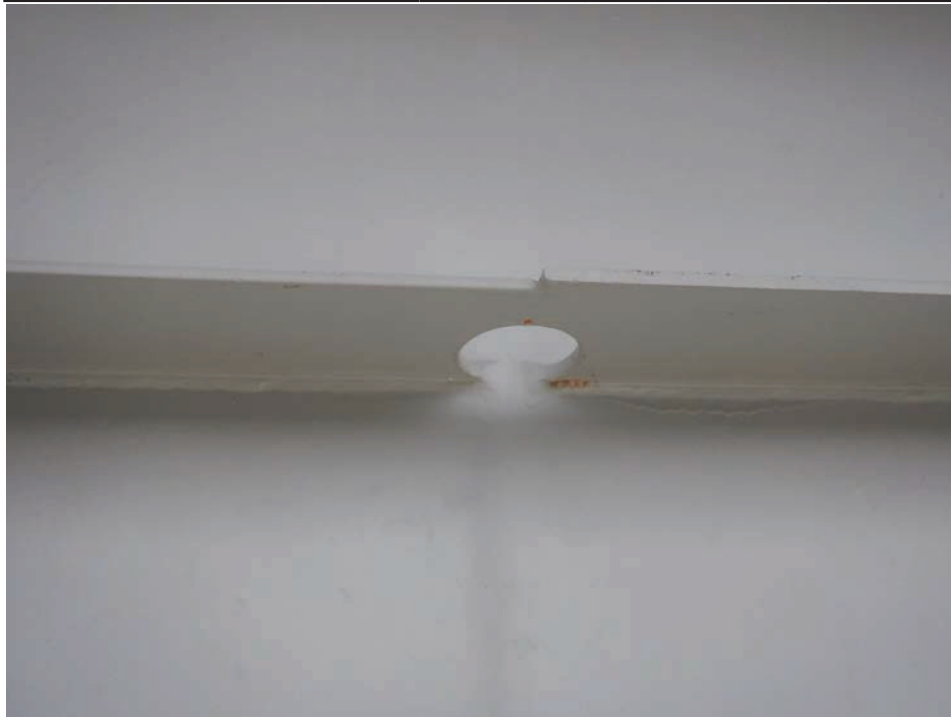
Photograph 14 - Looking north at girder 1, span 6 near floor beam 9. Note: drilled retrofit in upper horizontal stiffener.
