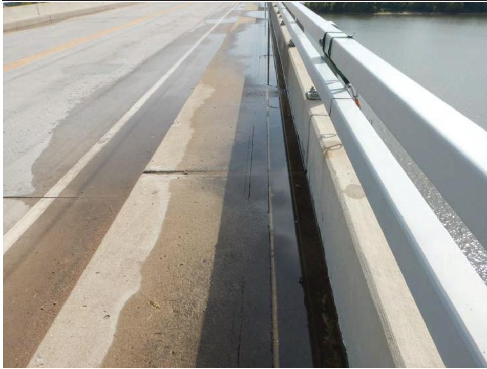
Photograph 3 - Looking east along the south bridge rail at floor beam 6, span 6. Note: ponding water on the sidewalk in span 6.
