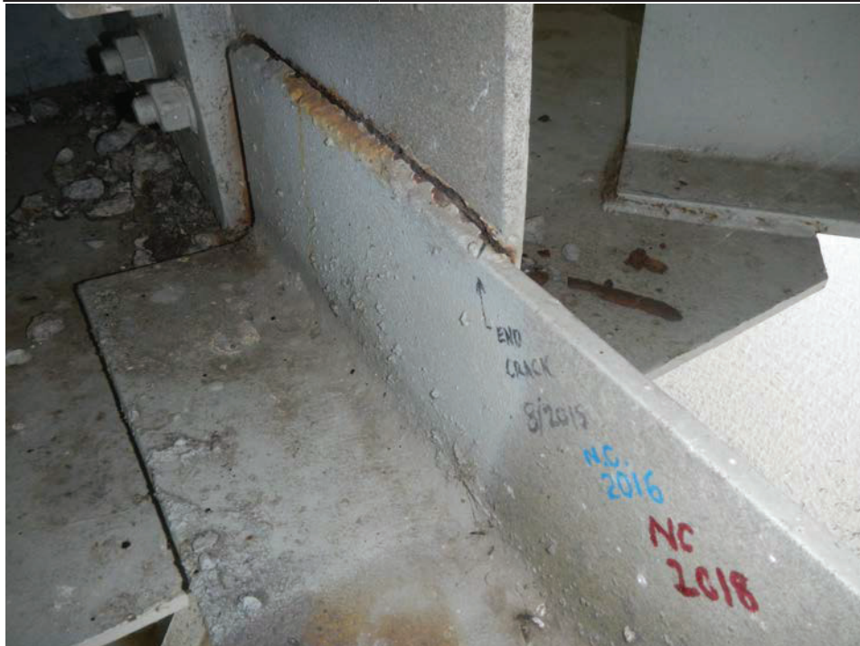
Photograph 20 - Looking northeast at the connection plate for floor beam 0, span 6 at the girder 2 bottom flange. Note: the horizontal weld has cracked full length.
