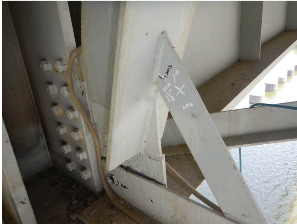
Photograph 21 - Looking northeast at the connection plate for floor beam 0, span 6 at girder 2 bottom flange. Note: 1/2-inch and 1 1/8-inch long cracks in welded repair plate.
