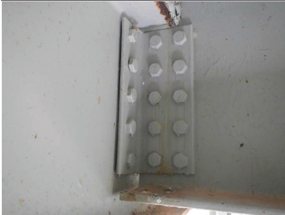
Photograph 18 - Looking northwest at the stringer 1 connection to floor beam 11 in span 6. Note: 5 loose bolts in connection angle to the floor beam web.
