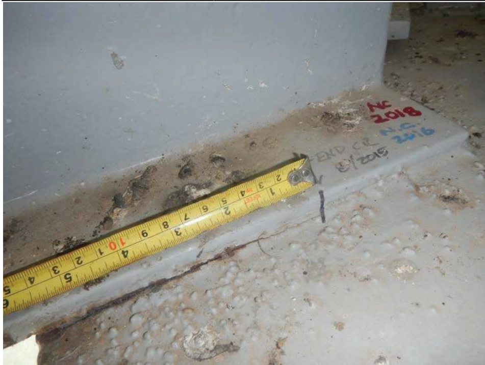
Photograph 22 - Looking west at the lower lateral bracing connection to the gusset plate at girder 2, east face of floor beam 12 in span 6. Note: 5 5/8-inch long crack in the weld between the bottom angle and the bracing gusset plate, no change since last inspection.
