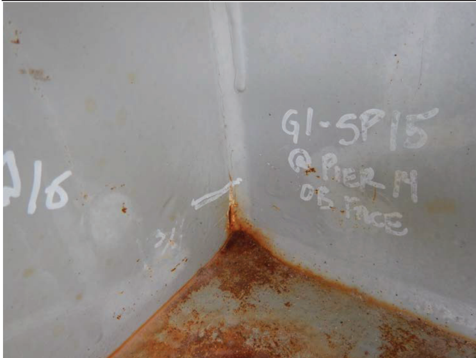
Photograph 16 - Looking south at beam 1 bearing stiffener for span 15 over pier 14. Note: 1 3/4-inch long vertical paint crack in the weld.
