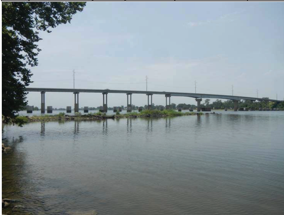
Photograph 2 - Looking southwest at the bridge elevation view.
