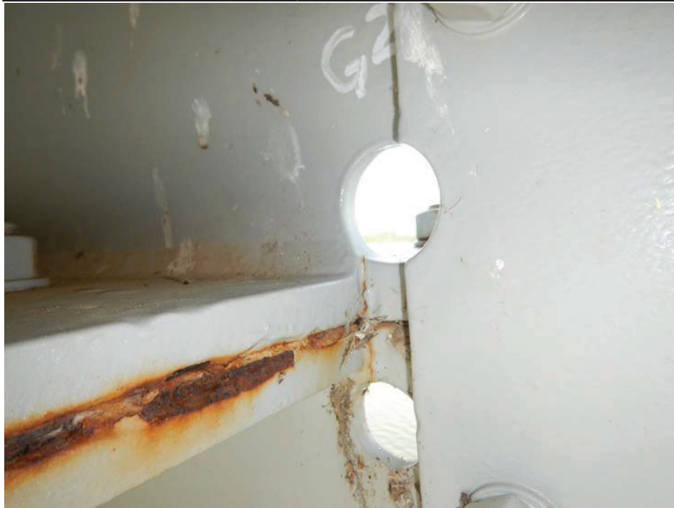
Photograph 10 - Looking northwest girder 2, span 7 at the termination of the horizontal stiffener near floor beam 4. Note: two vertical cracks arrested with drilled hole retrofits. No change from the 2017 inspection.
