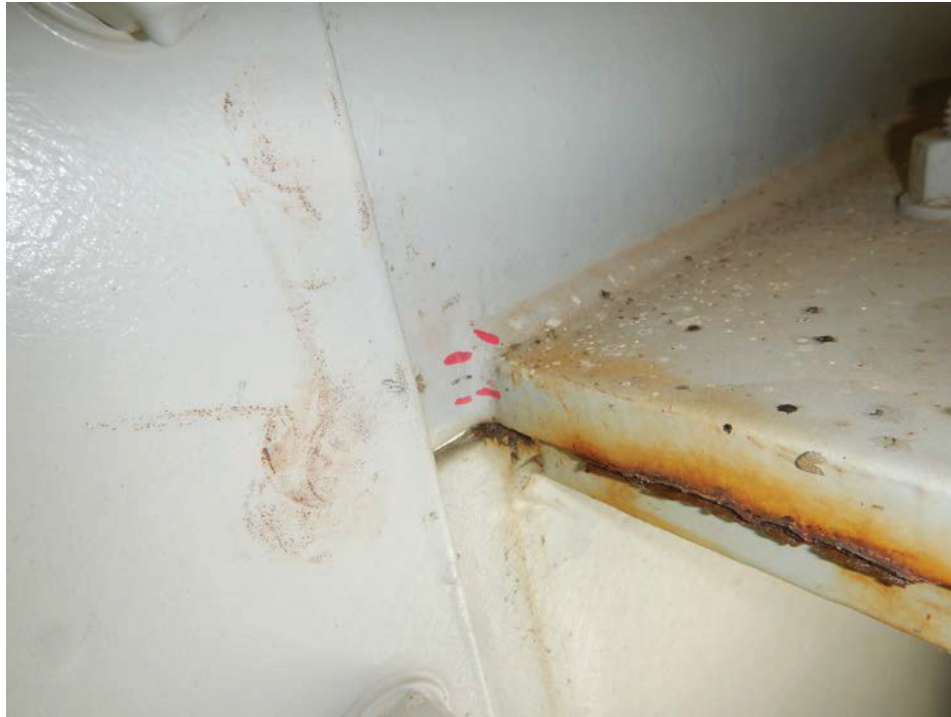
Photograph 7 - Looking northeast at girder 2, span 5 at the termination of the horizontal splice east of floor beam 5. Note: new 1/2-inch long paint crack adjacent to the previously noted 3/8-inch long paint crack.
