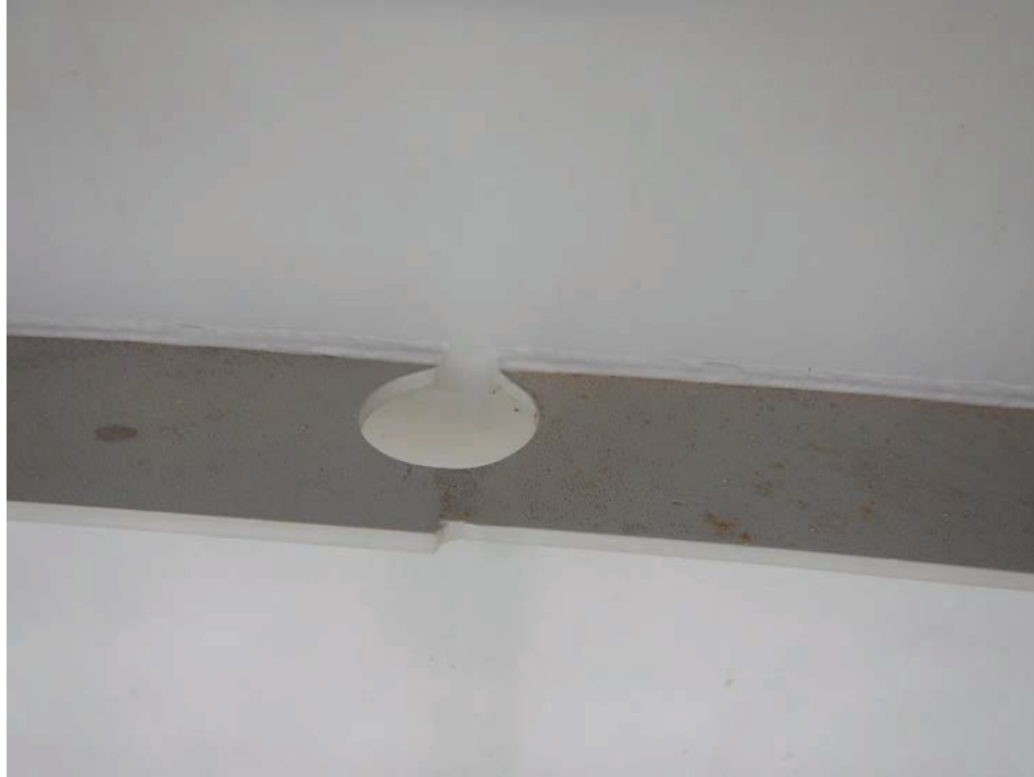
Photograph 15 - Looking south at girder 2, span 6 near floor beam 9. Note: drilled retrofit in upper horizontal stiffener.
