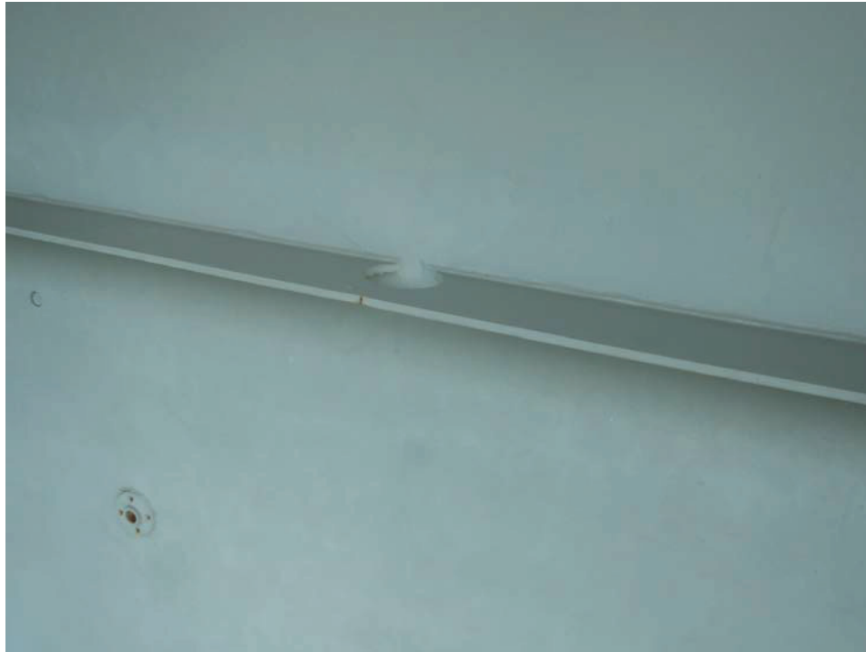
Photograph 13 - Looking north at girder 1, span 6 near floor beam 7. Note: drilled retrofit in upper horizontal stiffener.
