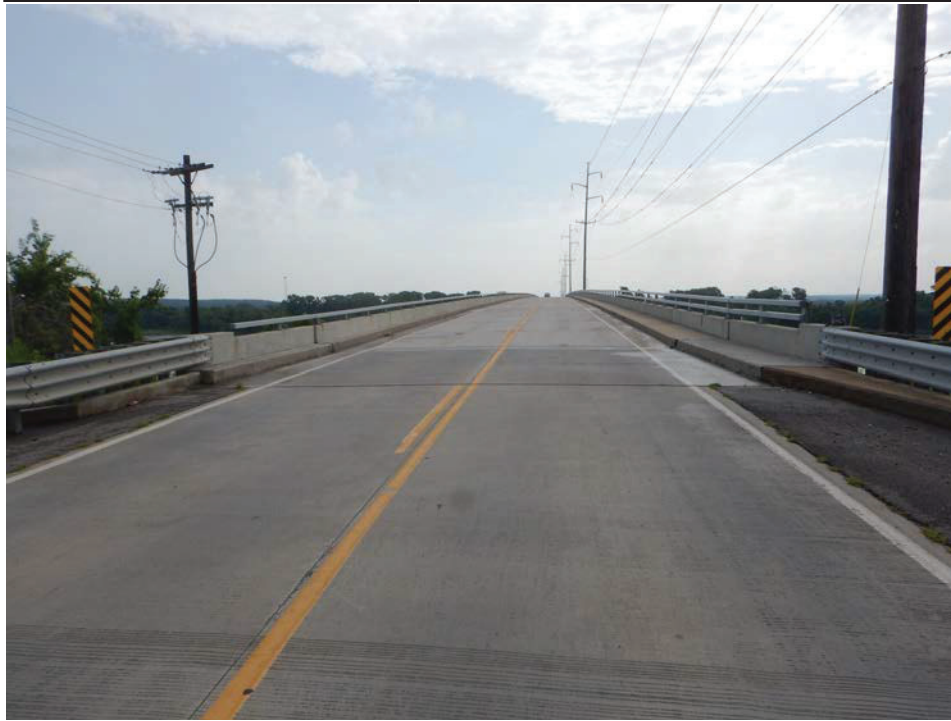
Photograph 1 - Looking east at the bridge end view.
