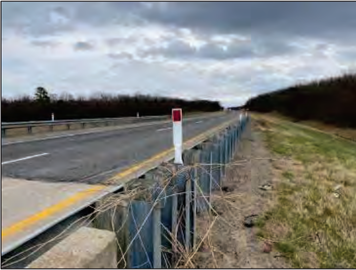
Photograph 38: Eastern edge of study area along I-40, south side facing west.
