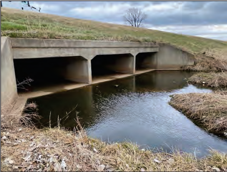
Photograph 8: NBI: 16907 (Structure 5), and site of DF2. 15 barn swallow nests present.
