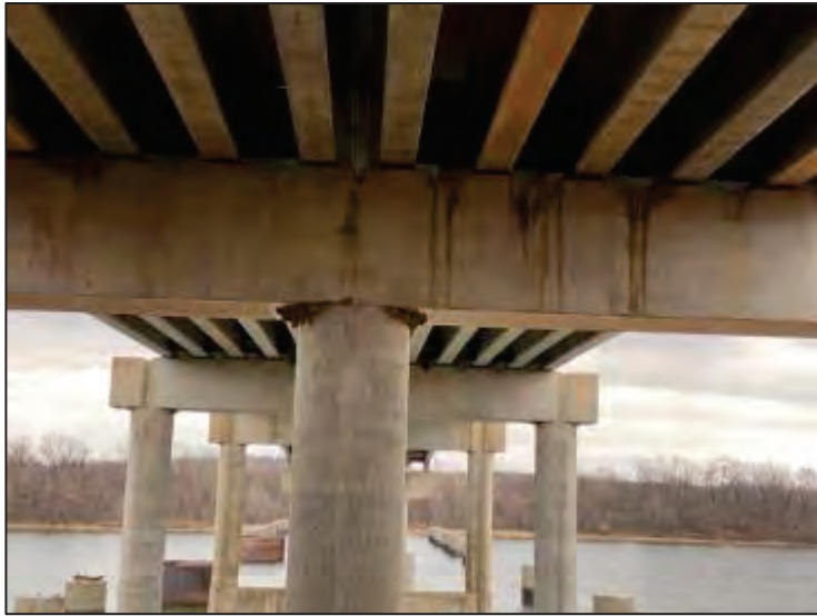
Photograph 19: Cliff swallow nests on bridge piers.
