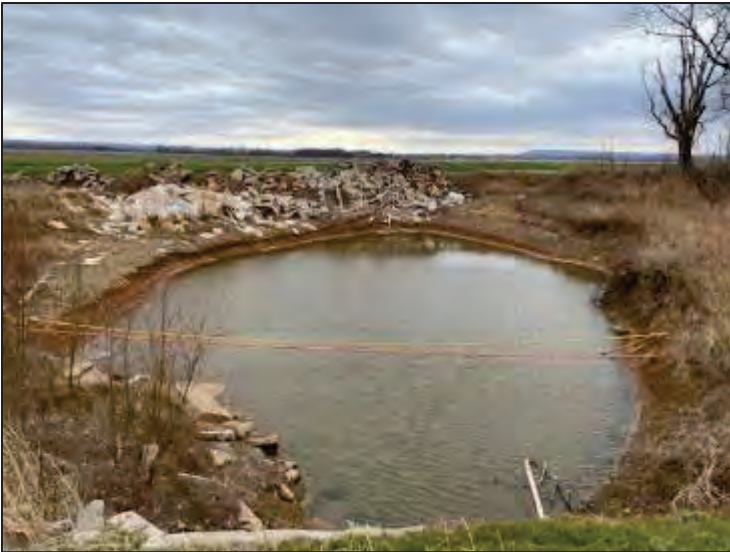
Photograph 12: Excavated hole south Structure 7. Exposed utilities and discarded debris.
