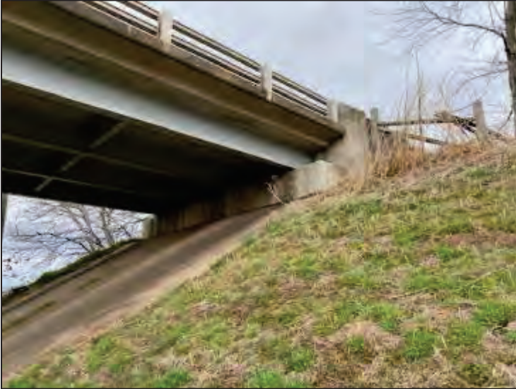
Photograph 2: NBI: 17013 (Structure 1) over I-40, no migratory bird nests present.
