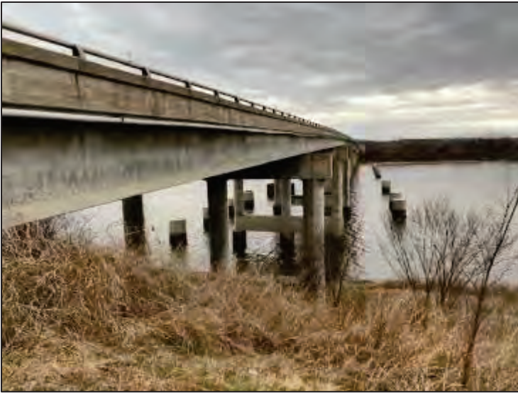
Photograph 18: NBI: 17051 (Structure 10) over Arkansas River.
