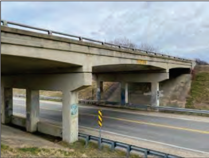
Photograph 30: NBI 16944 (Structure 13) over SH-10.
