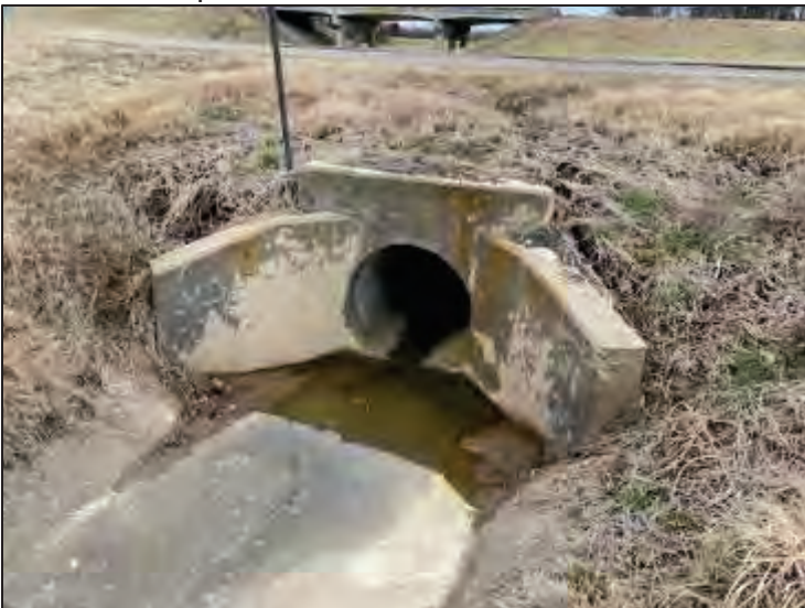
Photograph 34: Structure 16, no migratory bird nest or water feature present.
