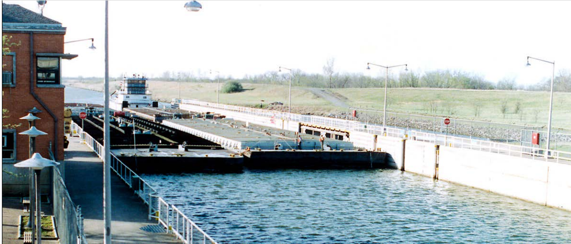
Figure 5.2-3: Typical Tanker Barge Tow in Lock Chamber (Tow Entering the Choteau Lock (USACE))
