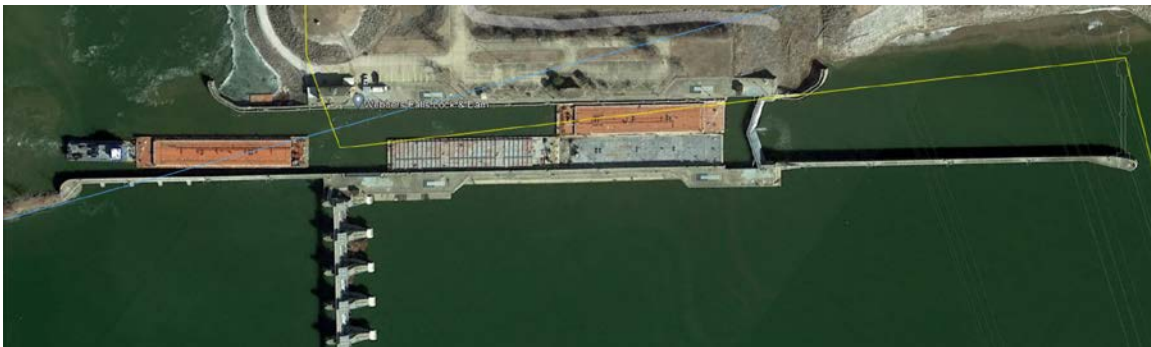
Figure 5.2-6: Tanker Barge Tow at Webbers Falls Lock and Dam 16
