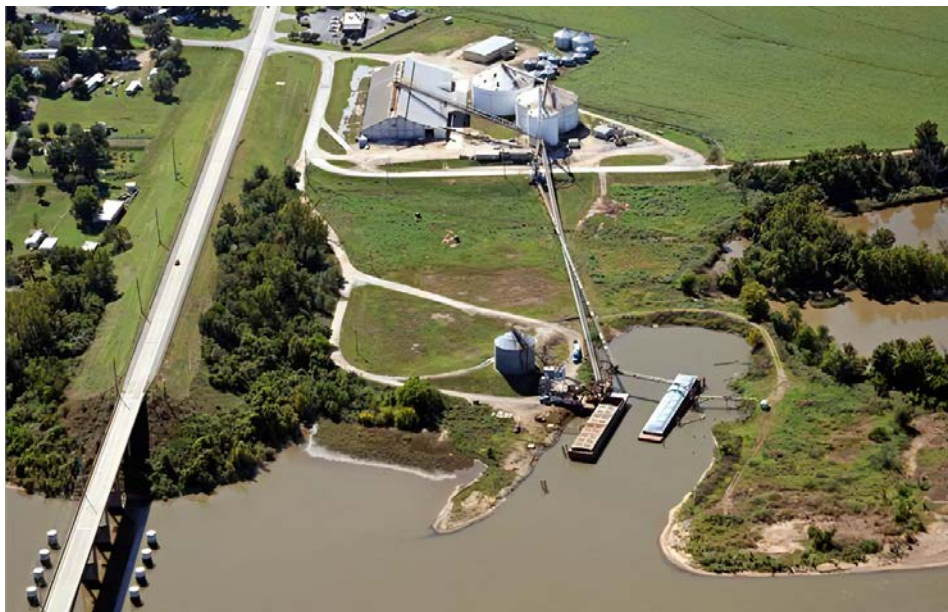
Figure 6.2-4: View of the Consolidated Grain and Barge Co Webbers Falls Dock
