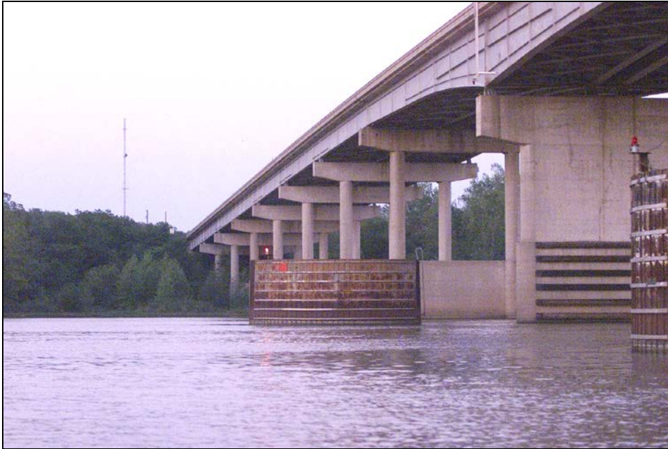
Figure 2.4-1: Sheet Pile Dolphins Upstream of Piers 4 and 5
