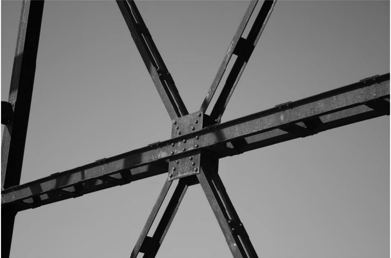
15. DETAIL VIEW OF GUSSET PLATE ON TRUSS, LOOKING NORTH
