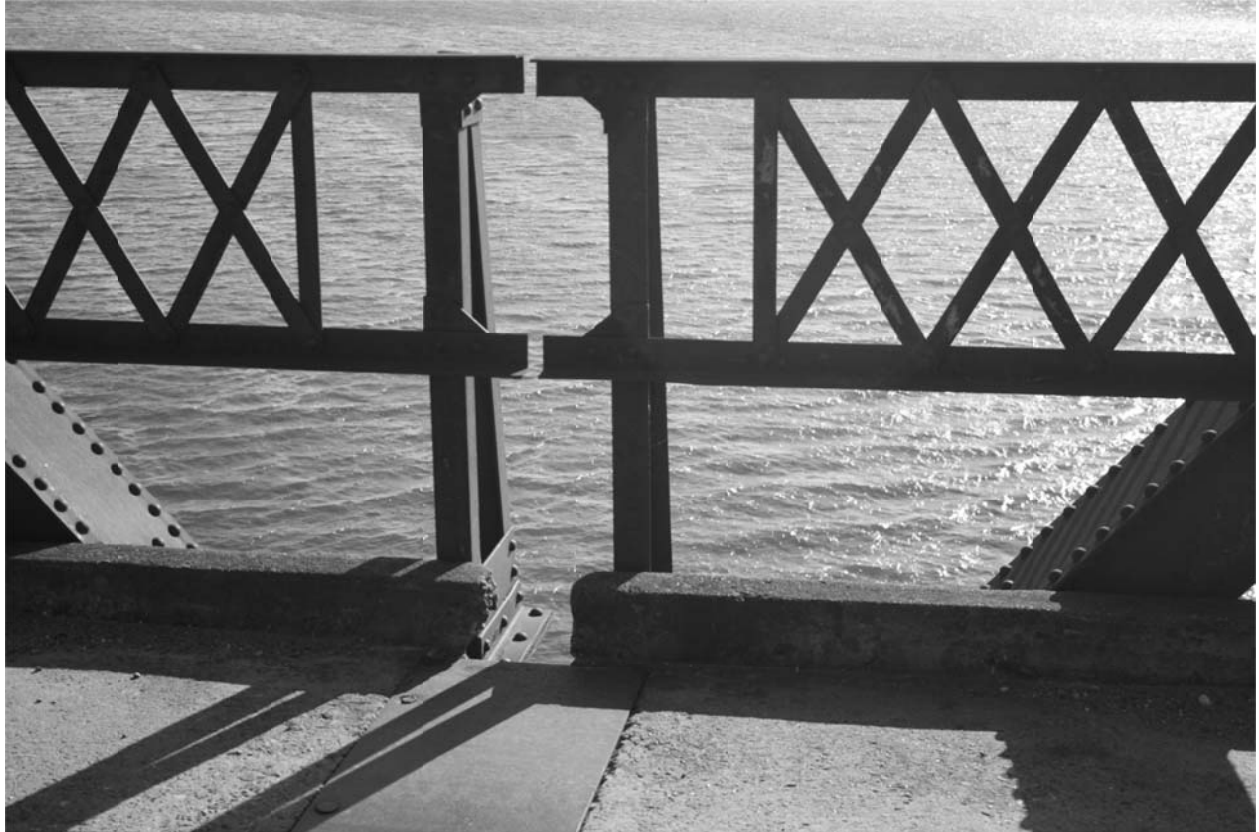
18. DETAIL VIEW OF SPAN CONNECTION, LOOKING SOUTH
