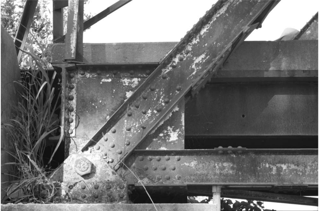
9. ABUTMENT GUSSET PLATE DETAIL, LOOKING NORTH
