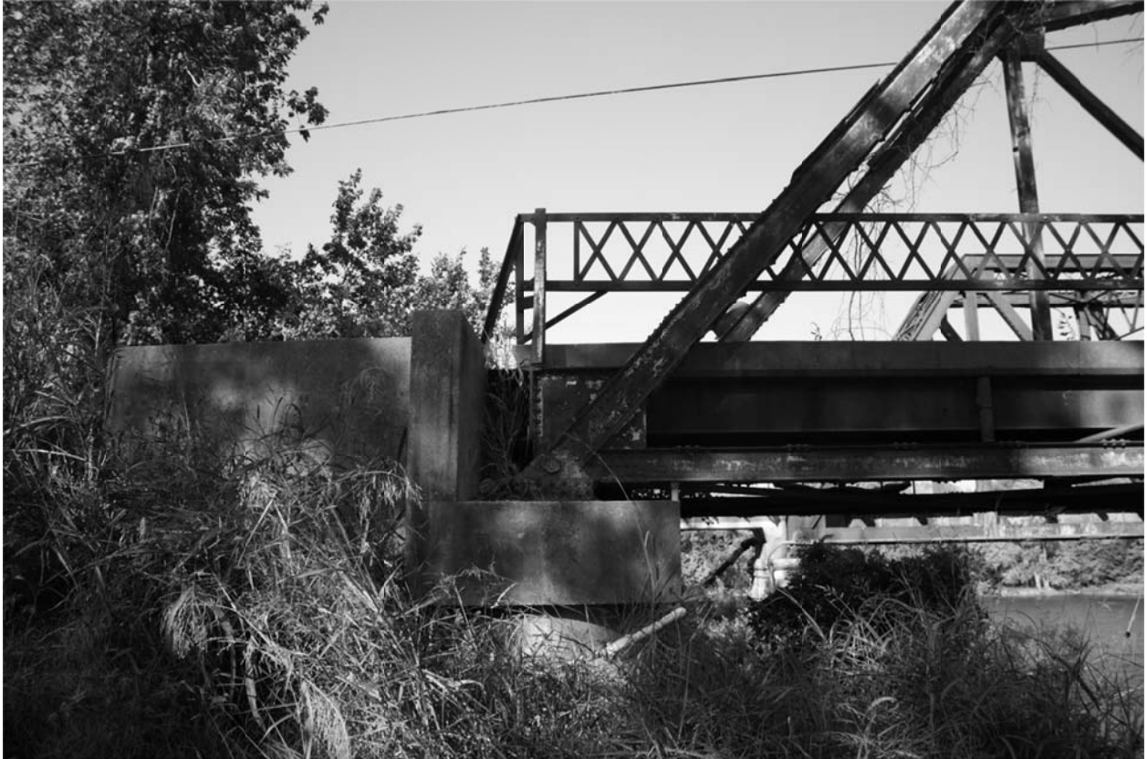
8. ABUTMENT AND DECK UNDERSIDE, LOOKING NORTH
