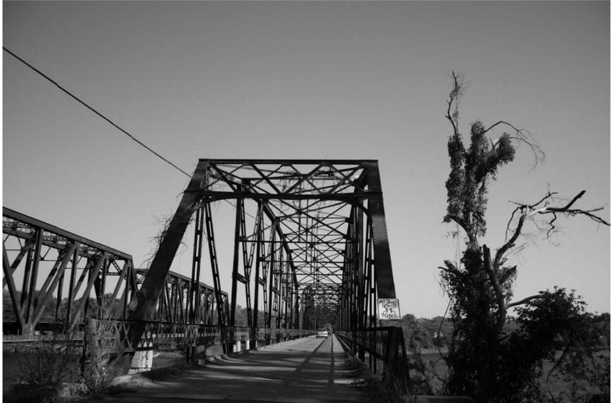
1. BRIDGE DECK AND TRUSS VIEW, LOOKING SOUTHEAST
