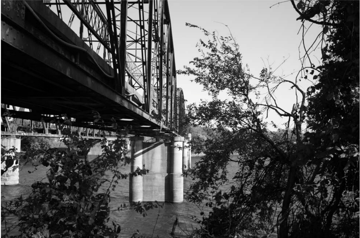
6. PIERS, LOOKING SOUTHEAST
