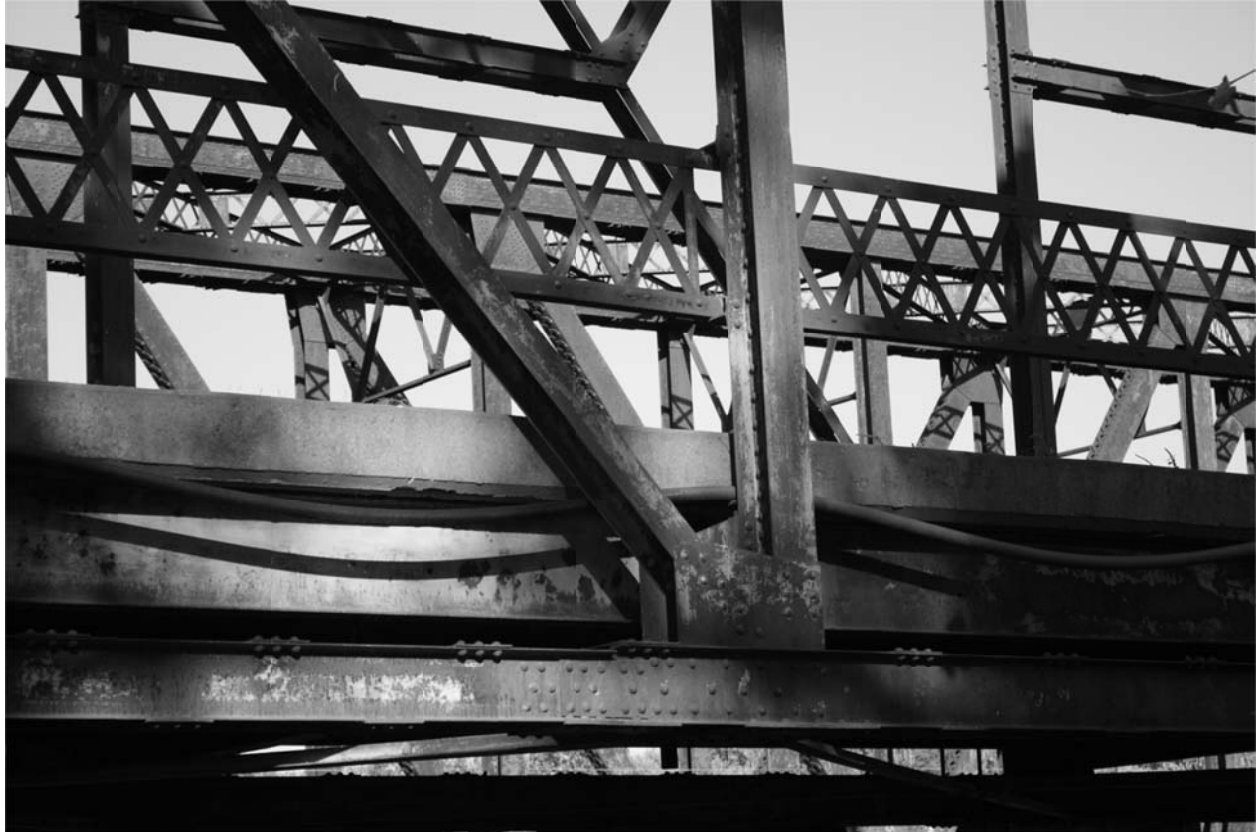
10. DETAIL VIEW OF GUSSET PLATE AT DECK, LOOKING NORTH
