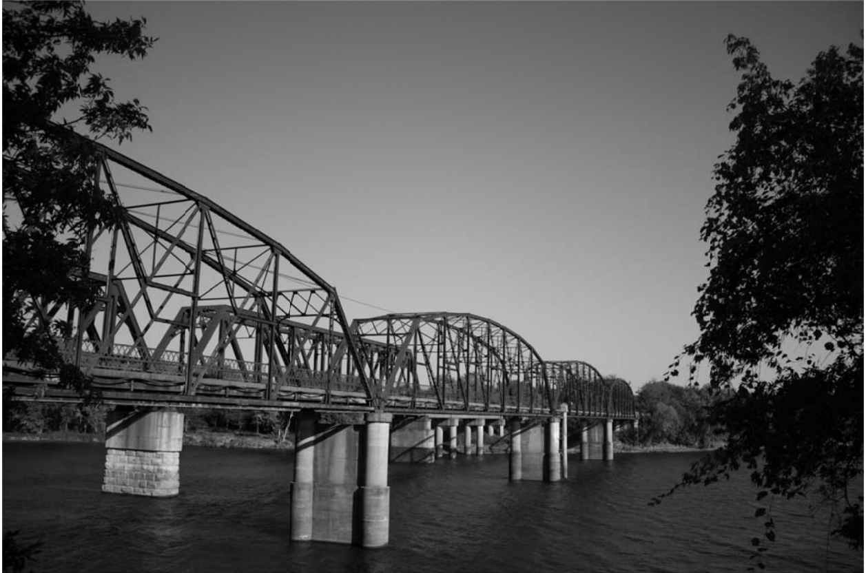
5. BRIDGE SIDE VIEW AND PIERS, LOOKING SOUTHEAST
