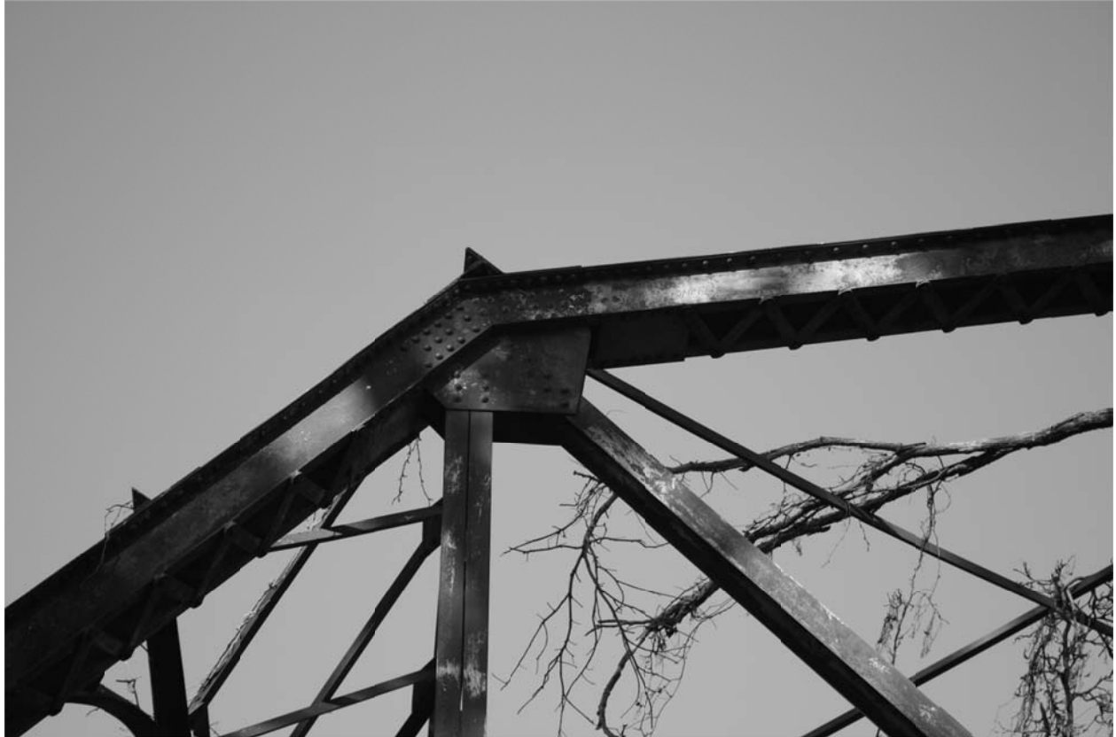
11. DETAIL VIEW OF GUSSET PLATE AT TRUSS, LOOKING NORTH
