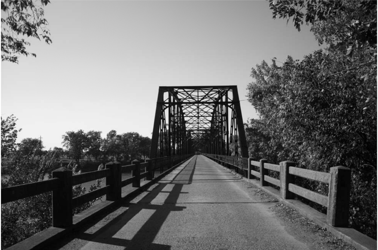
2. BRIDGE APPROACH, DECK AND TRUSS VIEW, LOOKING NORTHWEST
