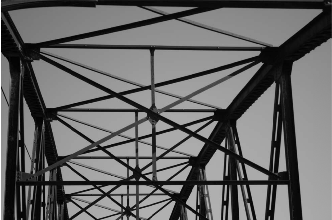
13. DETAIL VIEW OF OVERHEAD THROUGH TRUSS, LOOKING NORTHWEST
