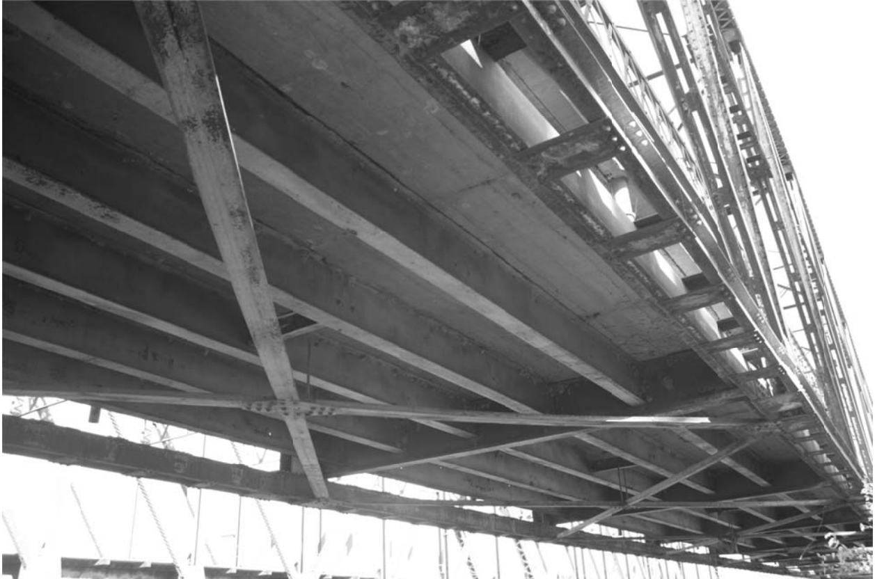
12. DETAIL VIEW OF UNDERSIDE, LOOKING NORTHEAST
