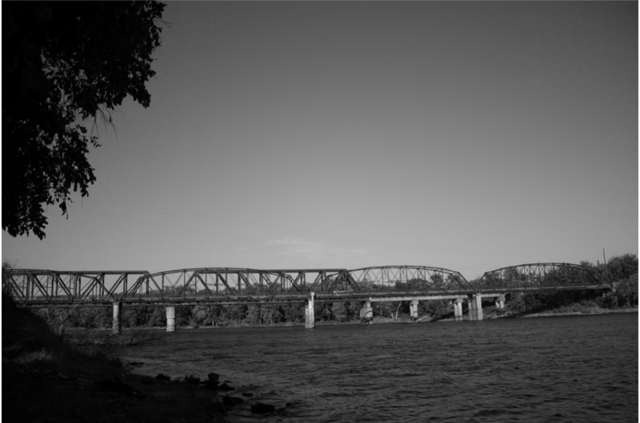
4. BRIDGE SIDE VIEW, LOOKING SOUTHEAST
