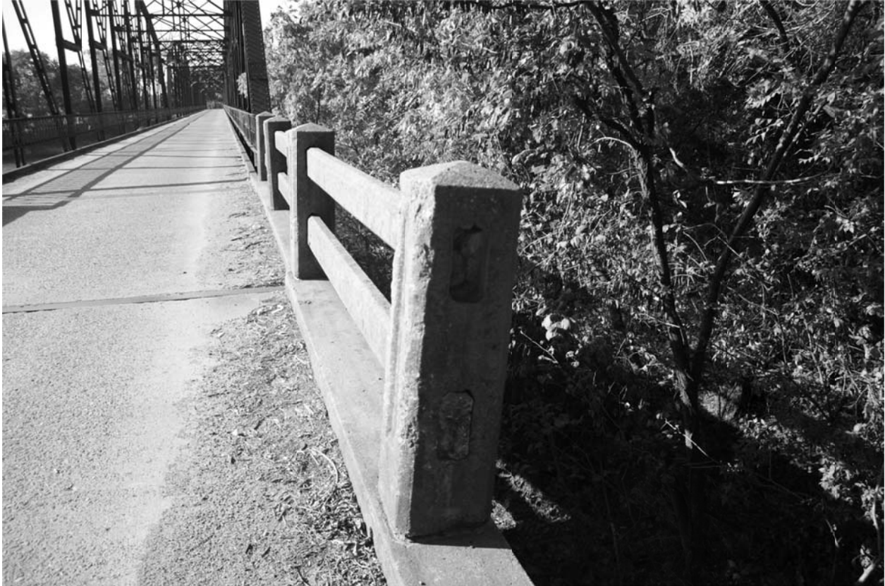
16. DETAIL VIEW OF CONCRETE POST AT SOUTH APPROACH, LOOKING NORTHWEST
