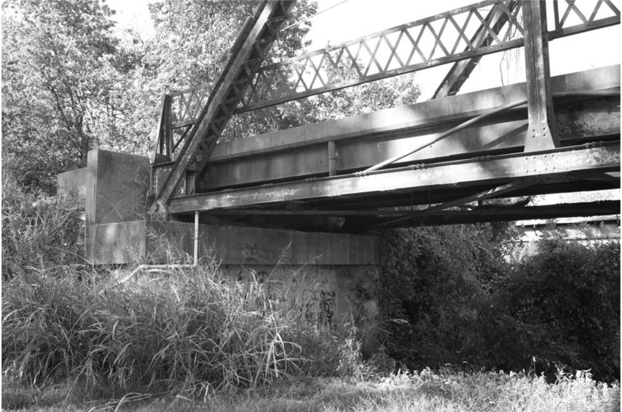
7. ABUTMENT, LOOKING NORTHWEST
