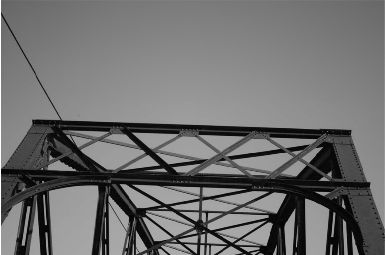
19. OVERHEAD DETAIL VIEW OF THROUGH TRUSS, LOOKING SOUTHEAST
