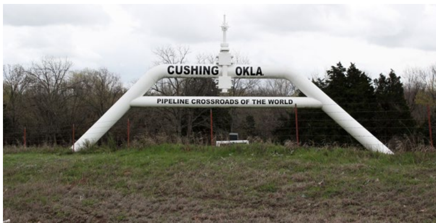
Figure 4-1. Pipeline Landmark in Cushing, OK
