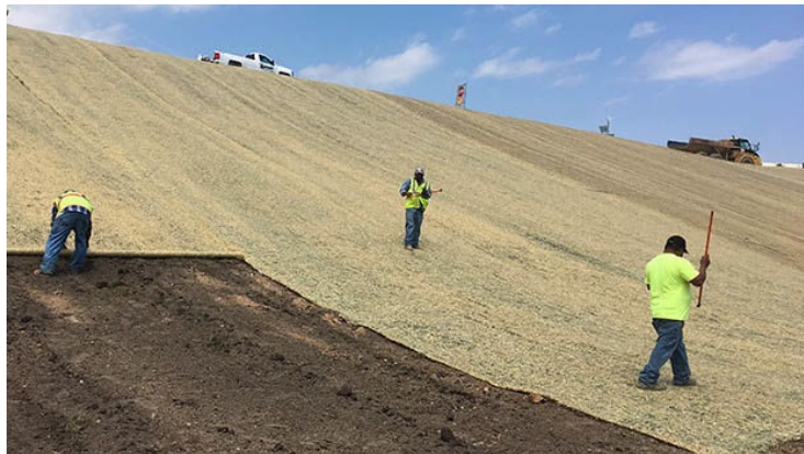
[Installation of Erosion Control Blanket on a slope]
