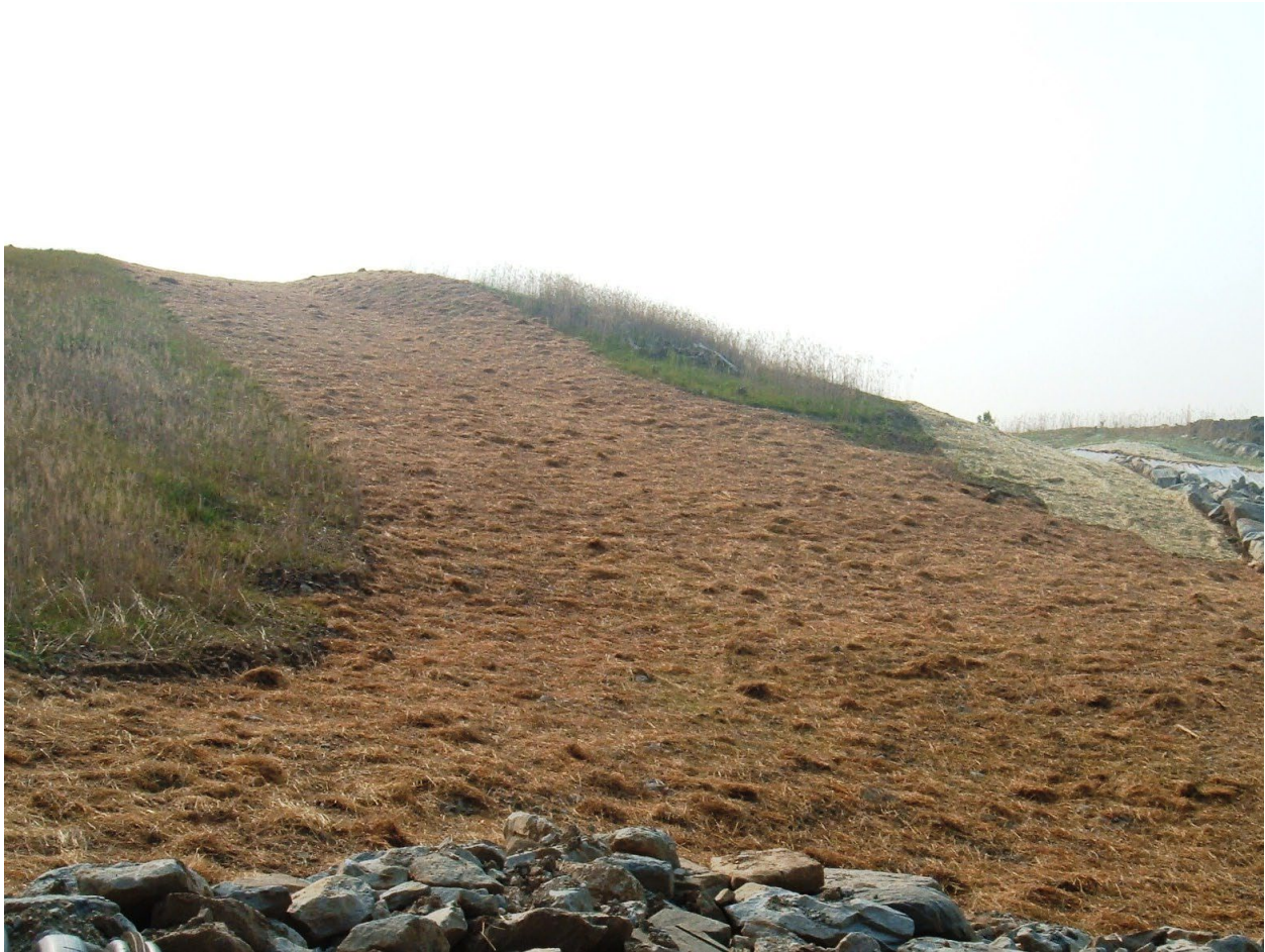
[Vegetative Mulch applied to a slope]
