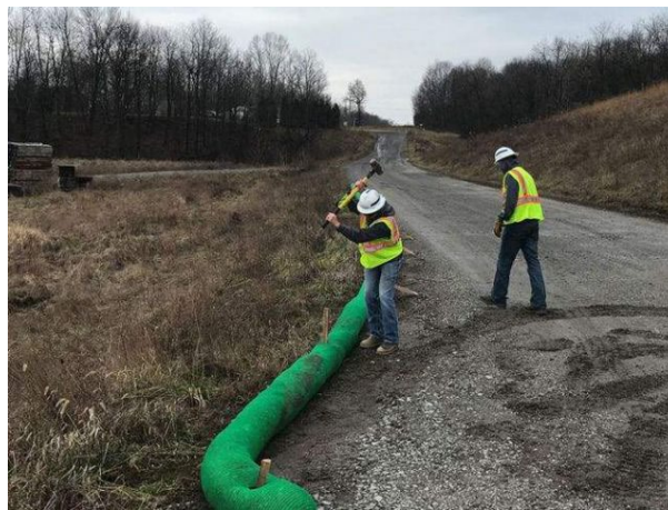
[Filtrexx Compost Filter Socks being fixed to the ground using stakes]
