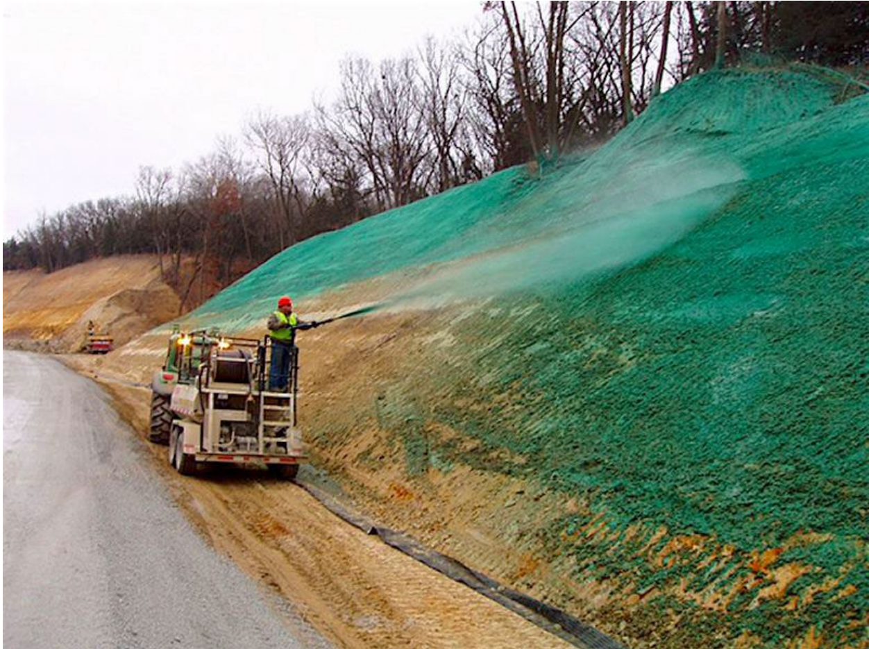
[Hydromulch being applied to a slope]
