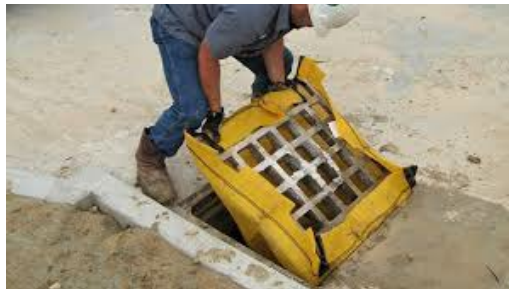
[Inlet Protection being installed on a storm drain]
