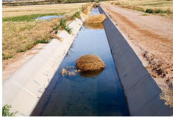
[Concrete drainage ditch]
