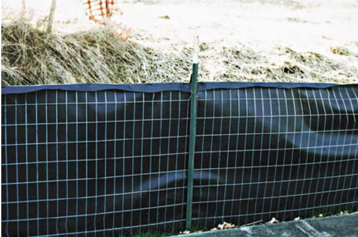
[Reinforced Silt Fence, outer view]
