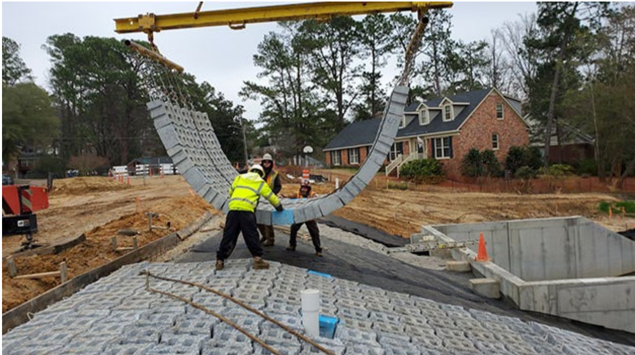
[Articulated Concrete Block Mat Installation]
