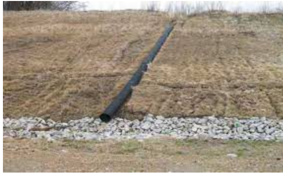
[Temporary Slope Drain]
