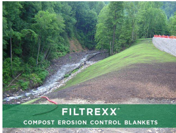
[Filtrexx Compost Erosion Control Blanket applied to a slope]
