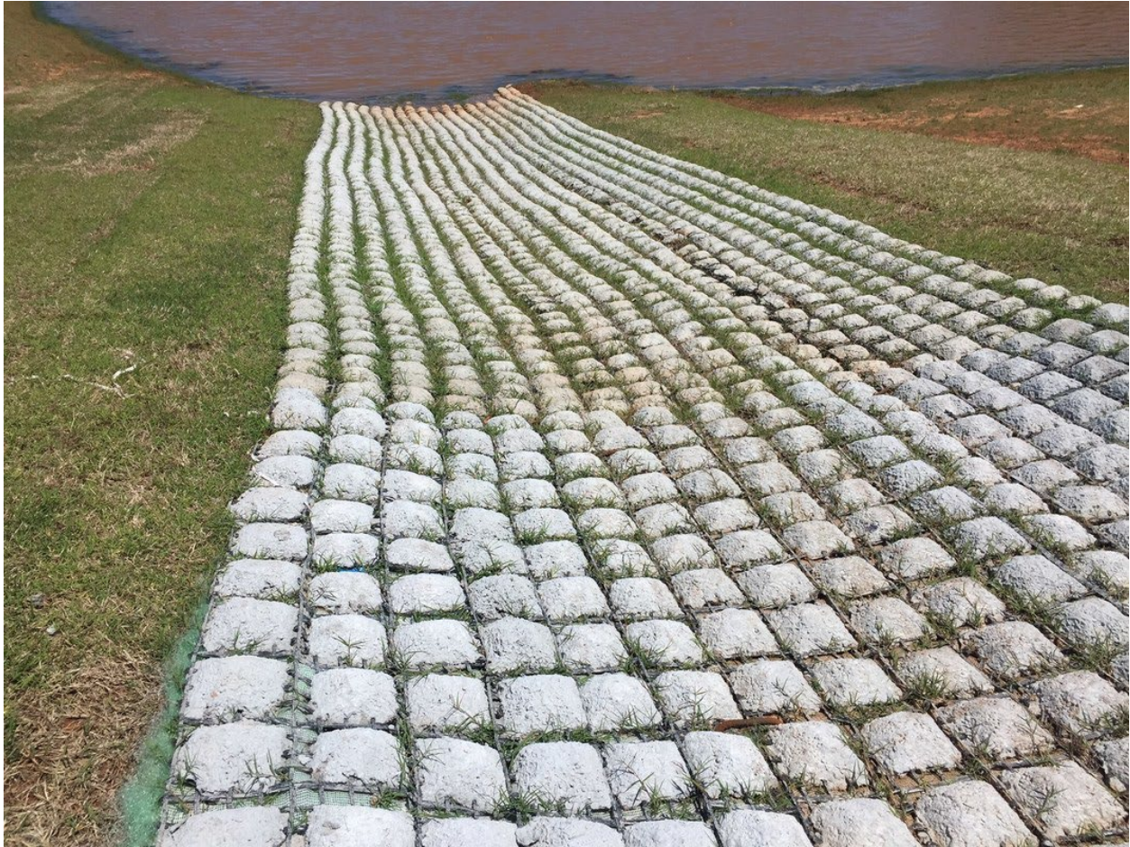
[Flexamat installed within a channel]
