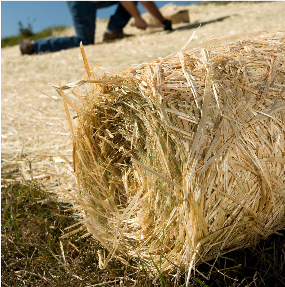
[Straw Blanket in the process of installation]
