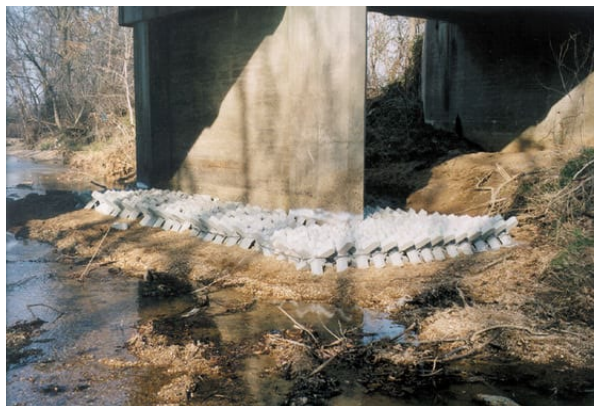
[A-Jacks Concrete Armoring Units used for Bridge Scour]
