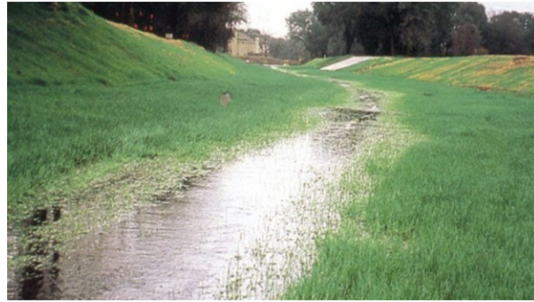
[Turf Reinforcement Mat used in an area of heavy flow]
