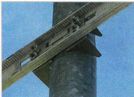
Saddle brackets are mounted on the flat side of the the C-Channel segment and face a standard pole
