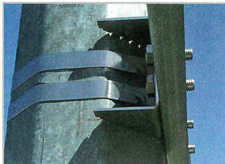
Notched saddle brackets are mounted to the flat side of the C-Channel and banding secures the assembly to an octagon pole
