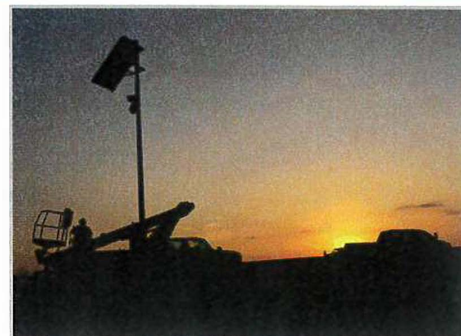
A crew finishes installing an SPM Tapered Pole Series kit
