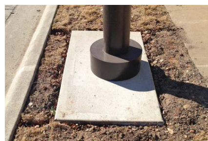
Acceptable Footer Detail
