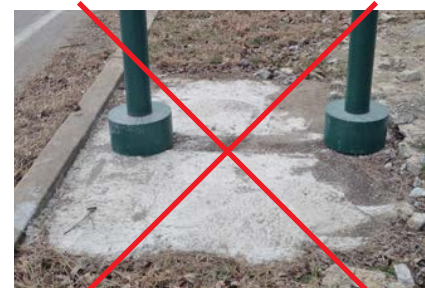
NOT Acceptable Footer Detail
