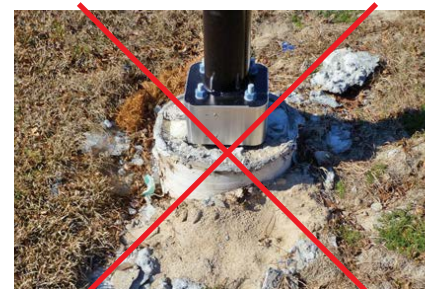
NOT Acceptable Footer Detail
