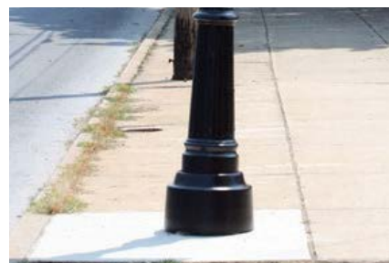
Acceptable Footer Detail
