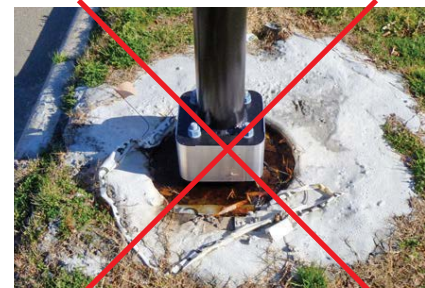
NOT Acceptable Footer Detail
