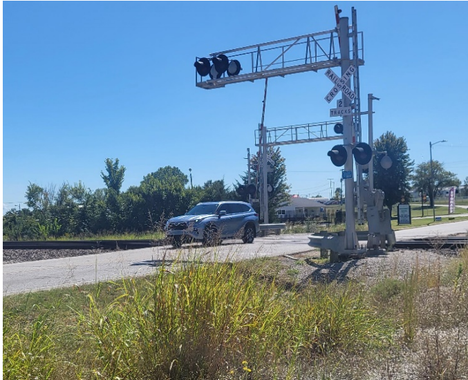
Figure 1 Railroad Crossing 673651V, Basin Rd., Mannford, OK.
