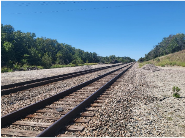
Figure 6 Side Track and BNSF Main Line, Mannford.
