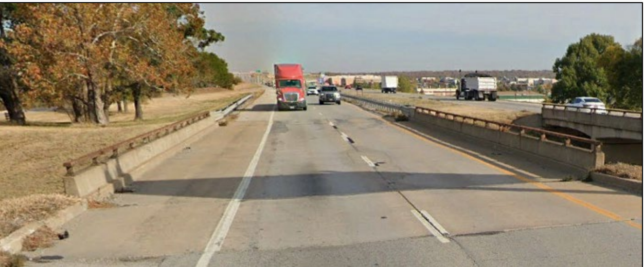
Figure 9: Existing US-75 Bridges over W. 81st Street
