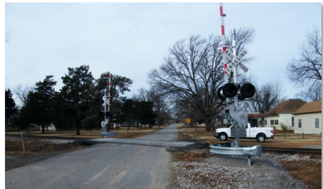
At-Grade Rail Crossing
