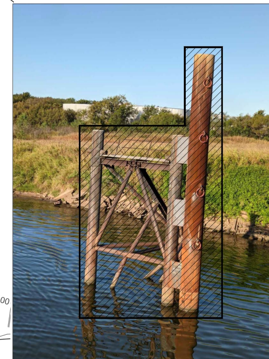
TYPICAL DOLPHIN DEMOLITION
