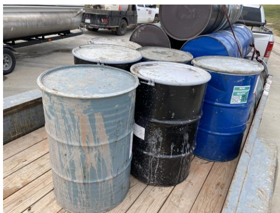
Photo #18: Four 55-gallon drums of soil cuttings from the soil boring installation. Eight empty/unlabeled drums are also located on the trailer.
