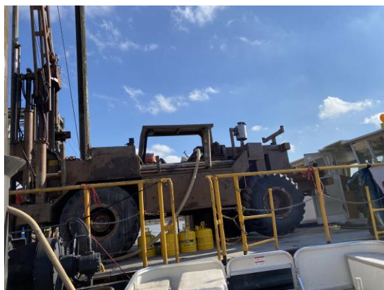
Photo #3: Representative photograph of drill rig set-up on the barge.
