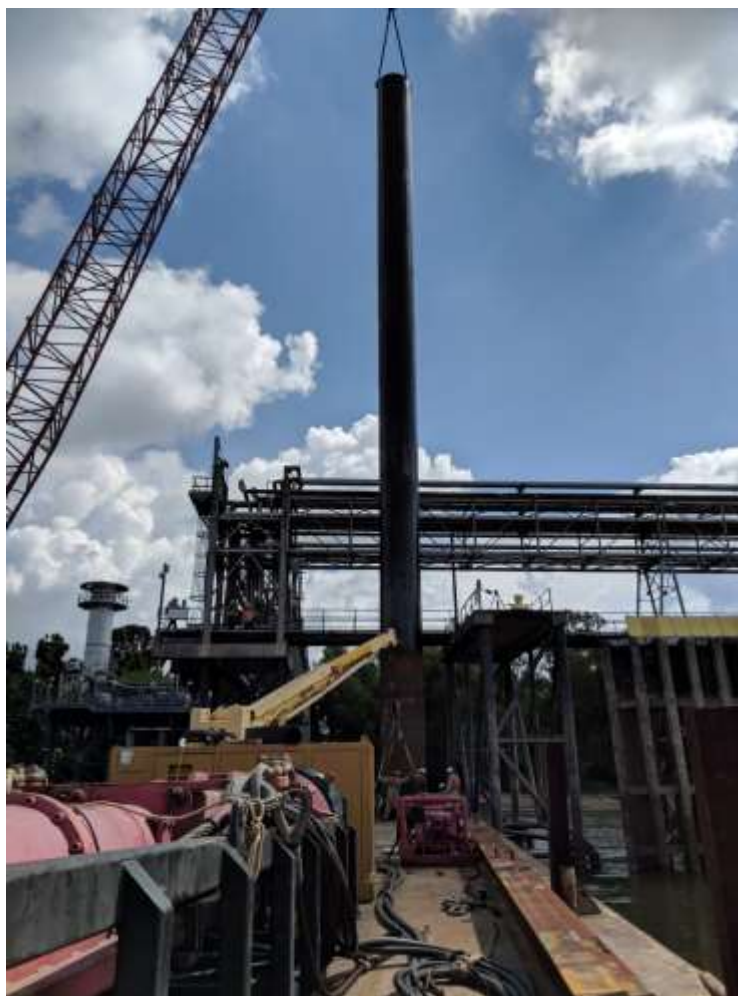
FIGURE 22 - MONOPILE INSTALLATION
