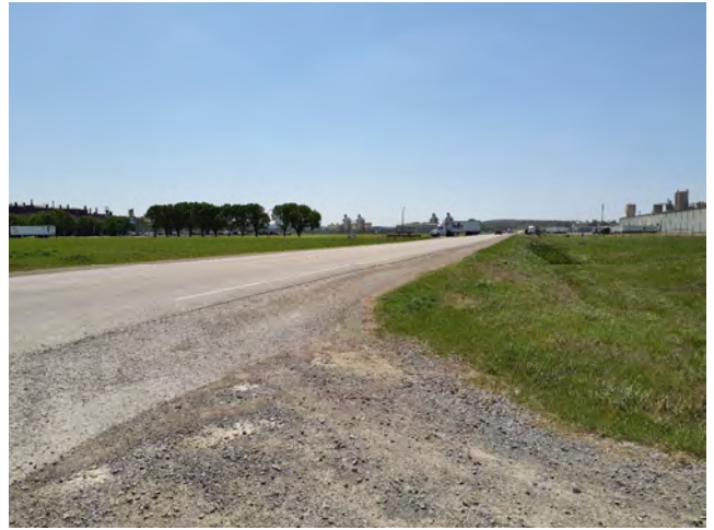
14. P4 looking south
