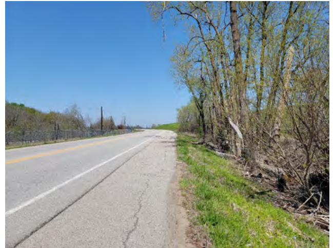
4. P2 looking north
