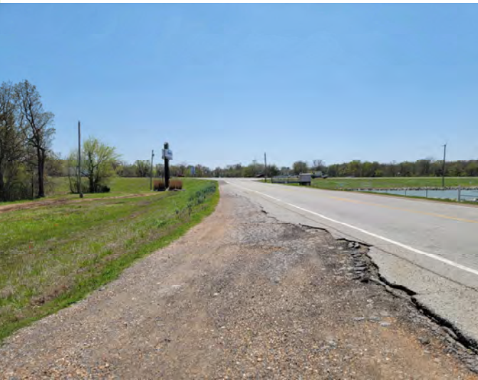
3. P1 looking south.
