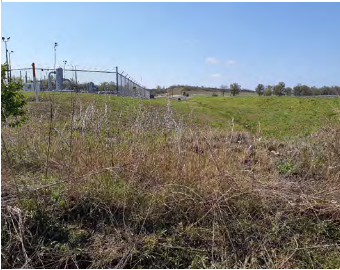
9. P3 looking south
