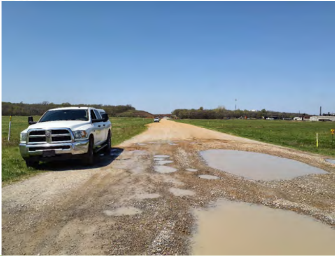
13. P4 looking west
