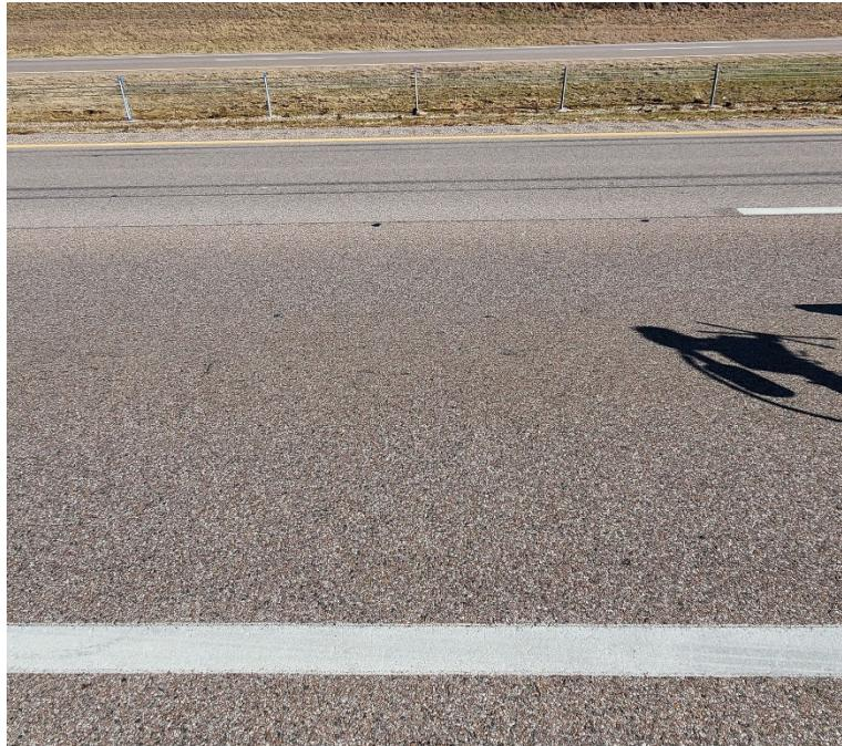
**Photo #37** Minor severity transverse cracking near C-37.
