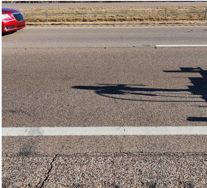
**Photo #34** Minor severity transverse cracking near C-34.
