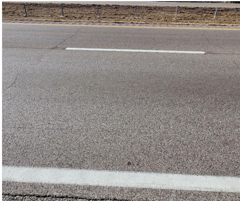
**Photo #10** Minor severity transverse cracking near C-10.
