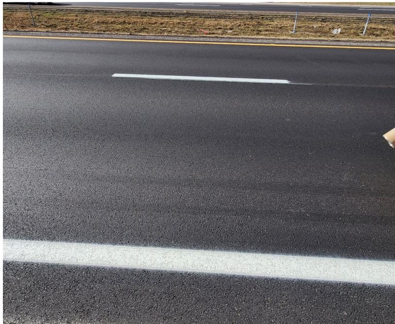
**Photo #20** Recent asphalt overlay near C-20.
