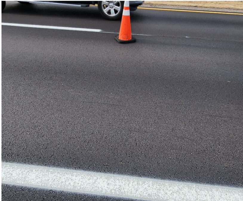
**Photo #16** Recent asphalt overlay near C-16.
