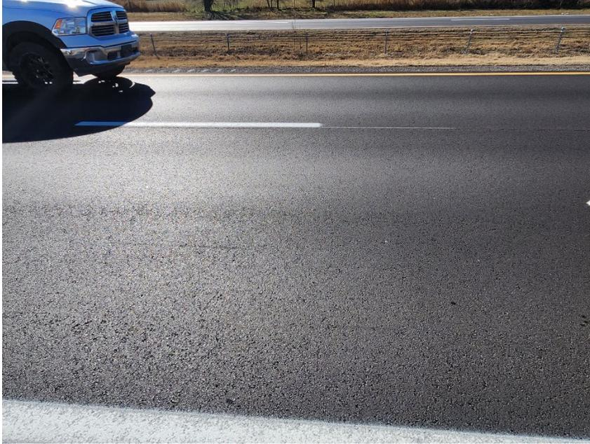
**Photo #15** Recent asphalt overlay near C-15.
