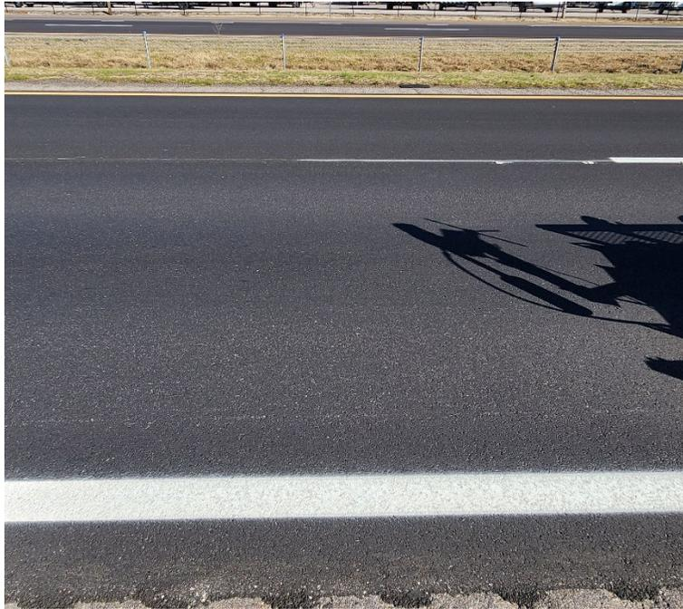
**Photo #25** Recent asphalt overlay near C-25.
