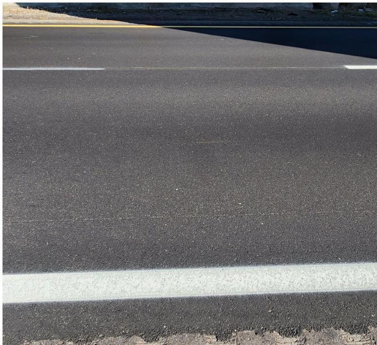
**Photo #26** Recent asphalt overlay near C-26.
