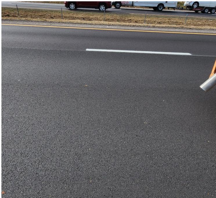
**Photo #22** Recent asphalt overlay near C-22.
