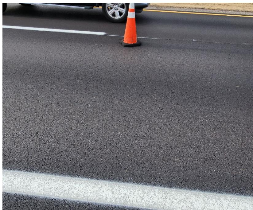
**Photo #16** Recent asphalt overlay near C-16.
