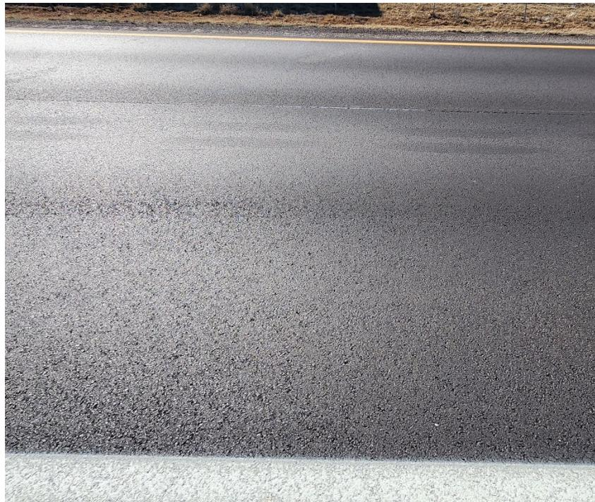
**Photo #14** Recent asphalt overlay near C-14.
