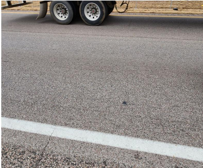
**Photo #1** Minor severity transverse cracking near C-1.
