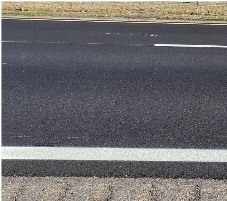
**Photo #24** Recent asphalt overlay near C-24.
