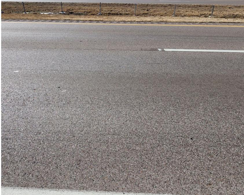
**Photo #13** No cracking observed near C-13.
