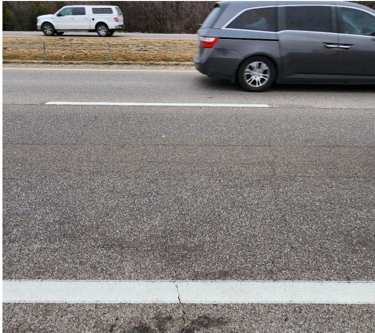
**Photo #43** Minor severity transverse cracking near C-43.
