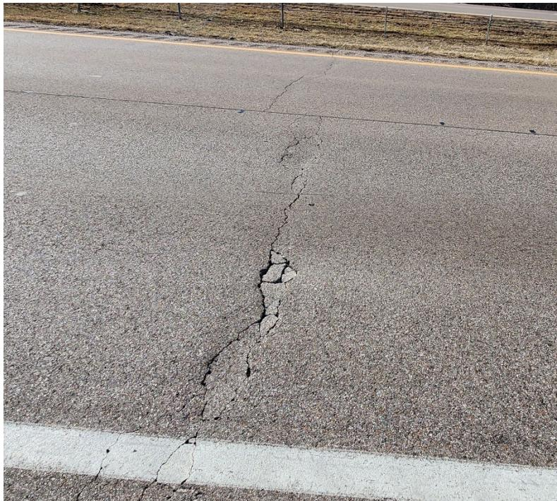
**Photo #11** Moderate severity transverse cracking near C-11.
