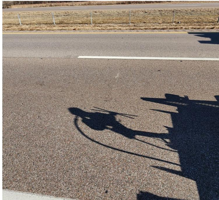
**Photo #36** Minor severity transverse cracking near C-36.
