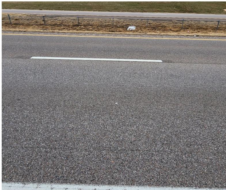
**Photo #4** Minor severity transverse cracking near C-4.
