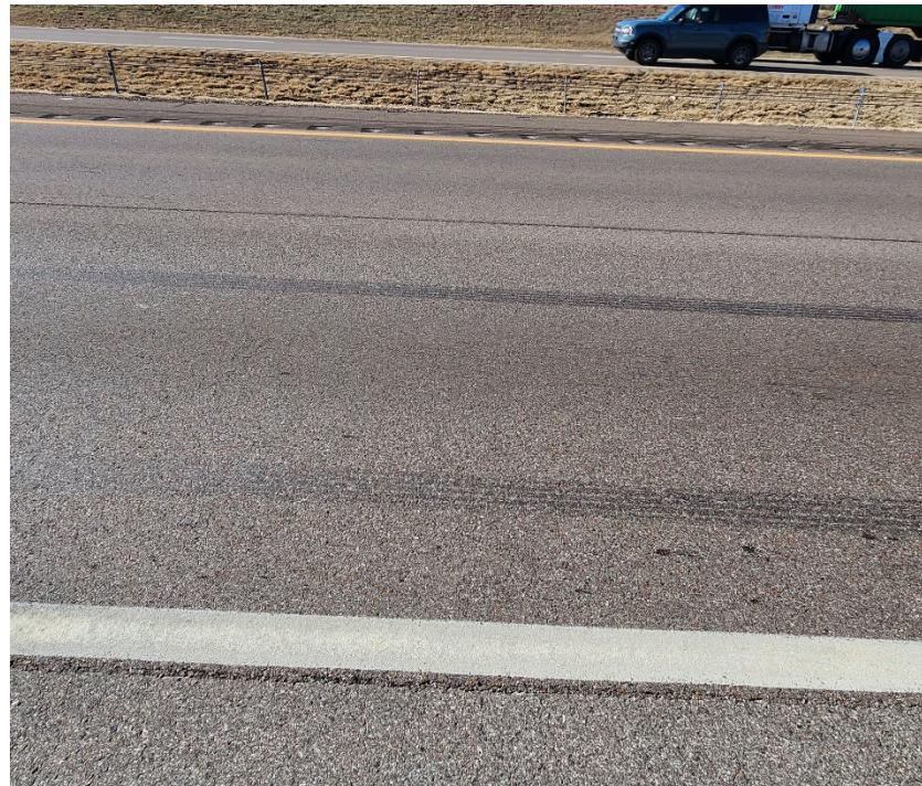
**Photo #8** No cracking observed near C-8.
