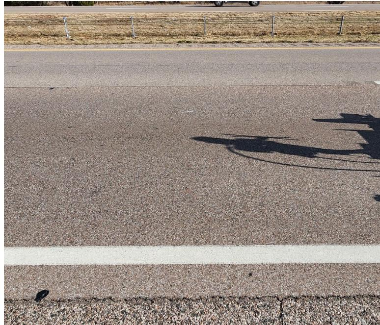
**Photo #35** Minor severity transverse cracking near C-35.
