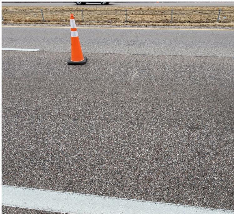
**Photo #46** Minor severity transverse cracking near C-46.
