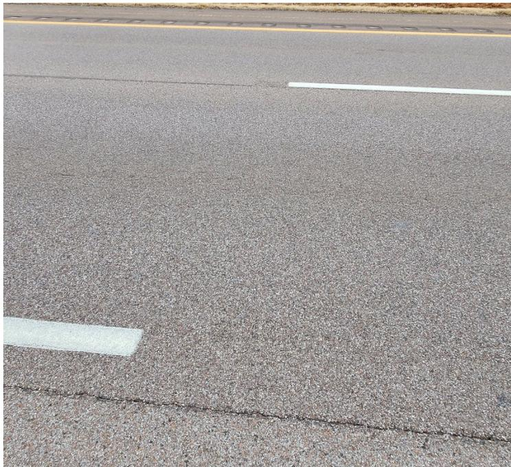
**Photo #42** No cracking observed near C-42.
