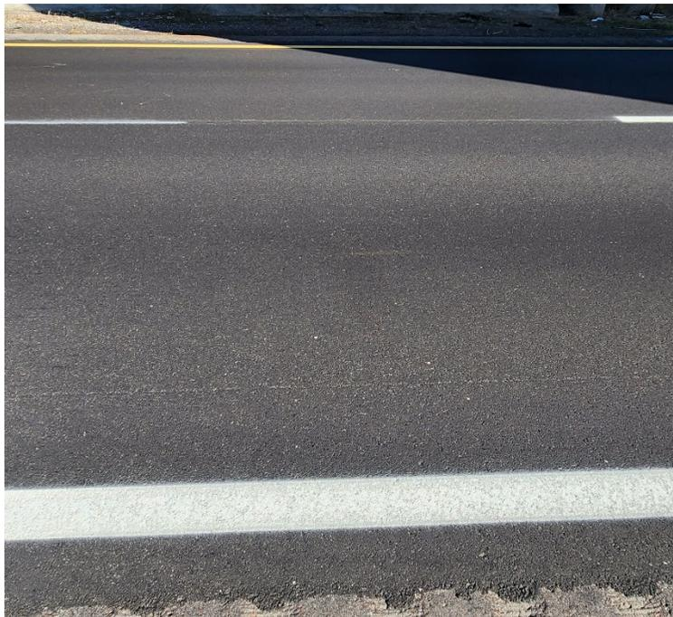
**Photo #26** Recent asphalt overlay near C-26.
