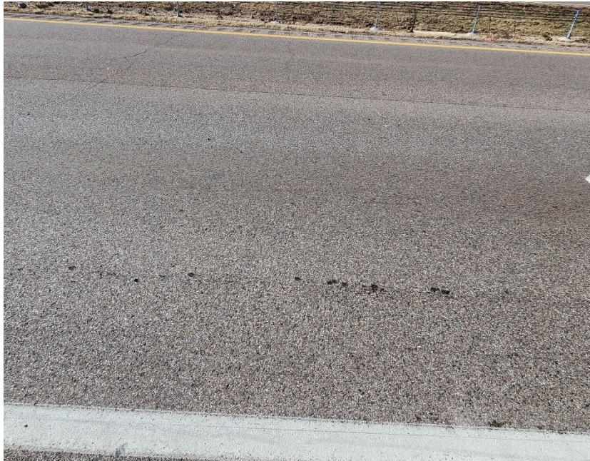
**Photo #9** Minor severity transverse cracking near C-9.
