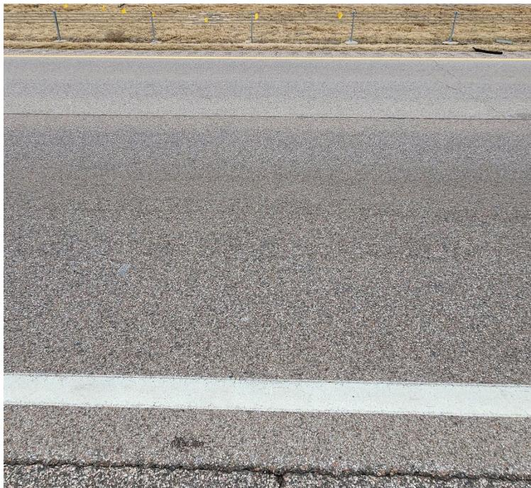
**Photo #44** Minor severity transverse cracking near C-44.
