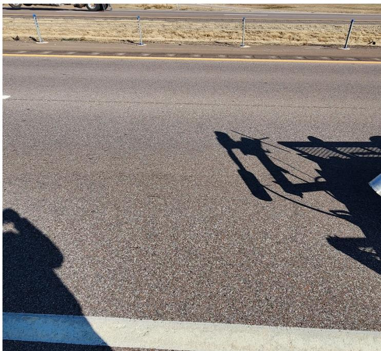
**Photo #40** No cracking observed near C-40.
