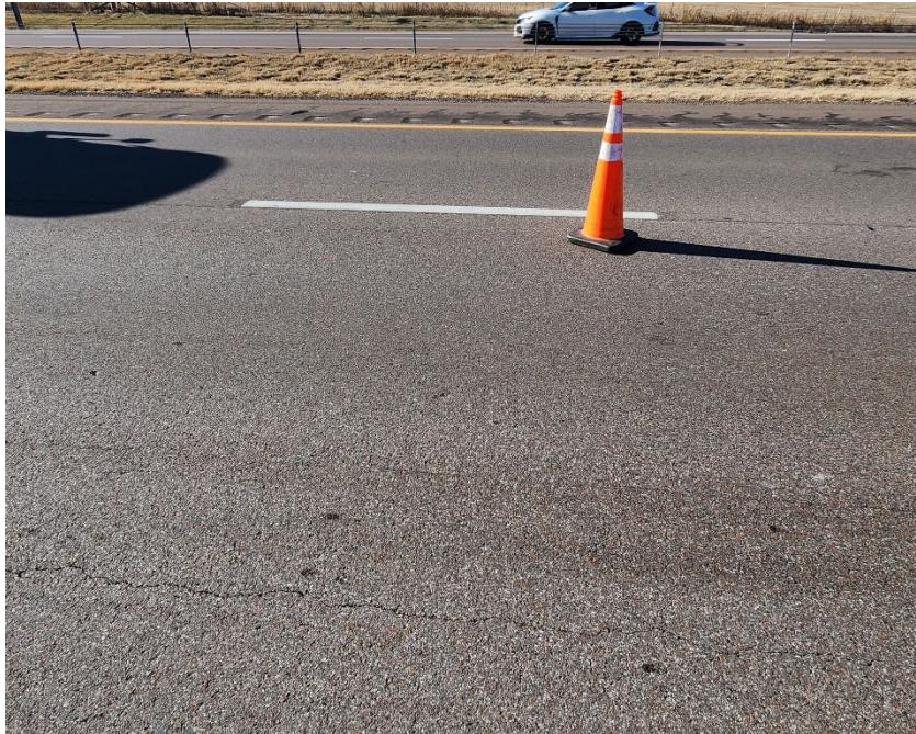
**Photo #7** Minor severity longitudinal cracking near C-7.
