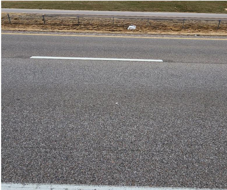
**Photo #4** Minor severity transverse cracking near C-4.
