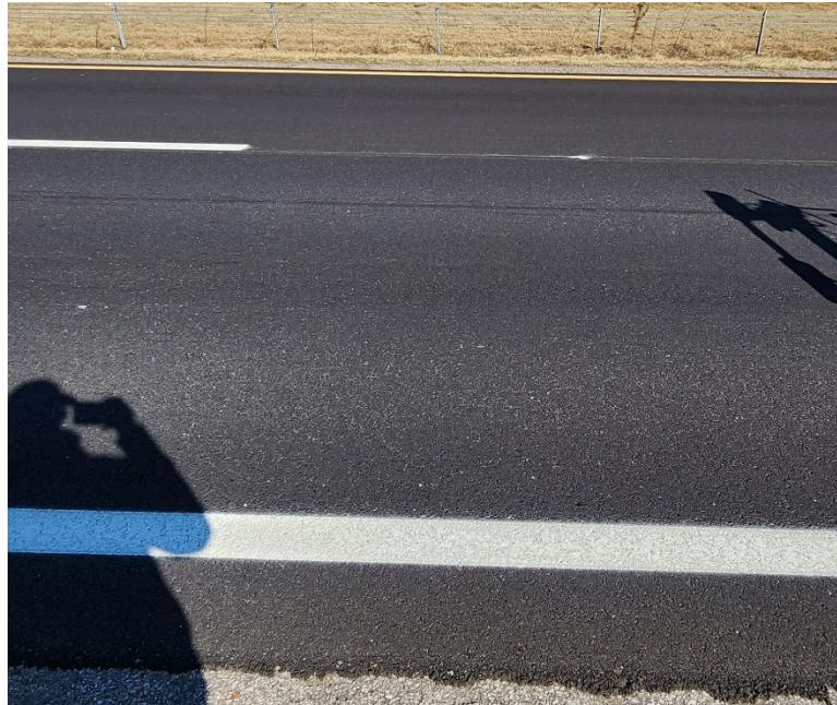
**Photo #29** Recent asphalt overlay near C-29.
