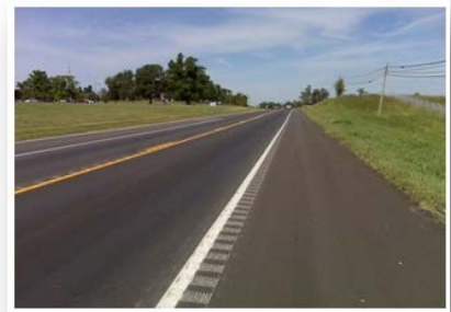
Centerline and edge line rumble strips
