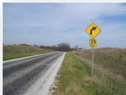
Curve warning sign
