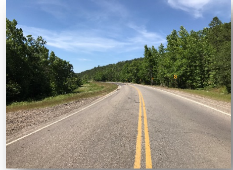
No Passing Zone pavement marking on US-259 north of Stevens Rd
