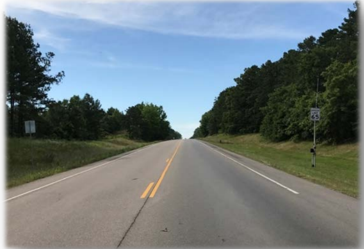
US-259 near Carson Creek Road (NB)
