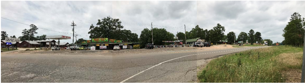
Wide, open driveways across from SH-259A (S)/US-259 intersection
