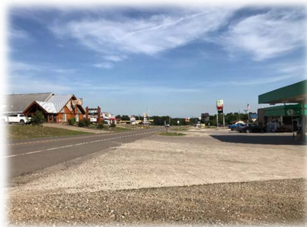
Location of E-Z Mart Gas Station (W70) Medium Priority access modification
