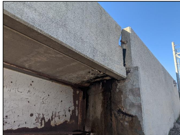
Figure 4: Deck Sliding
