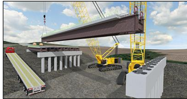
Figure 12: Example of PBES Installation
