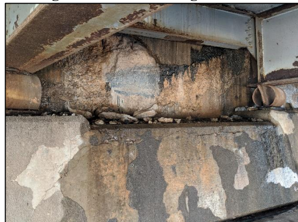
Figure 6: Deteriorating Abutment
