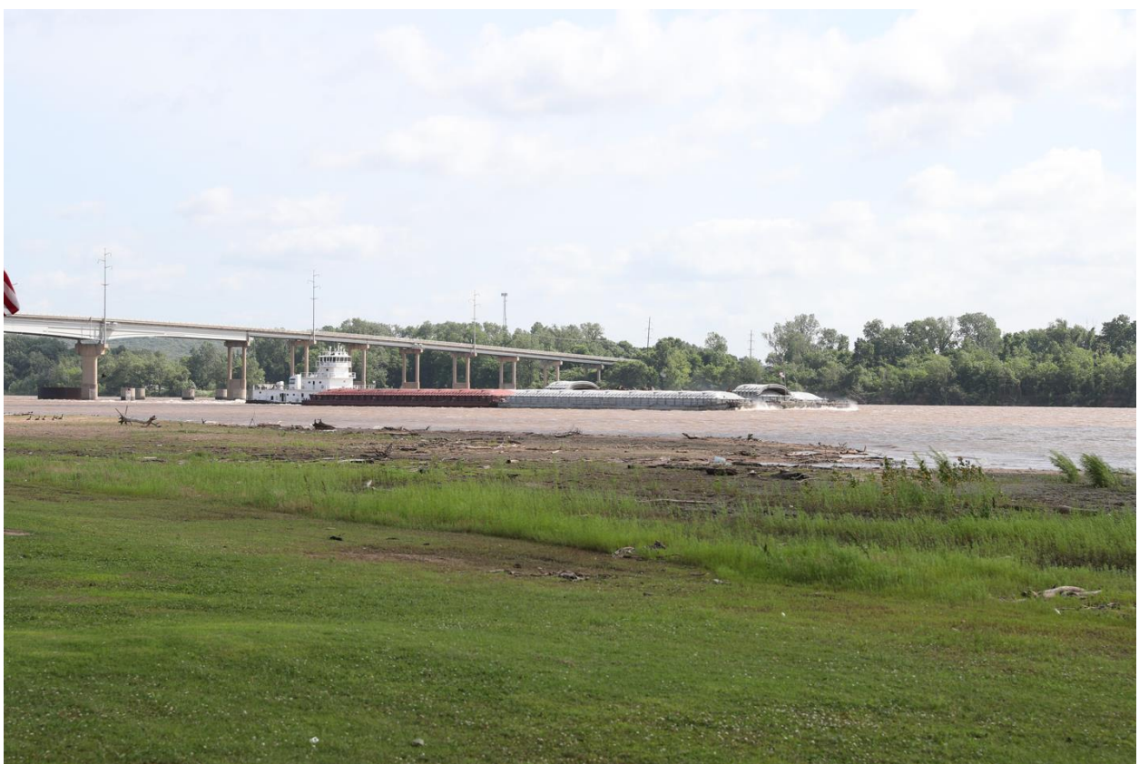
I-40 Bridge Replacement over the Arkansas River at Webbers Falls Site Photos
