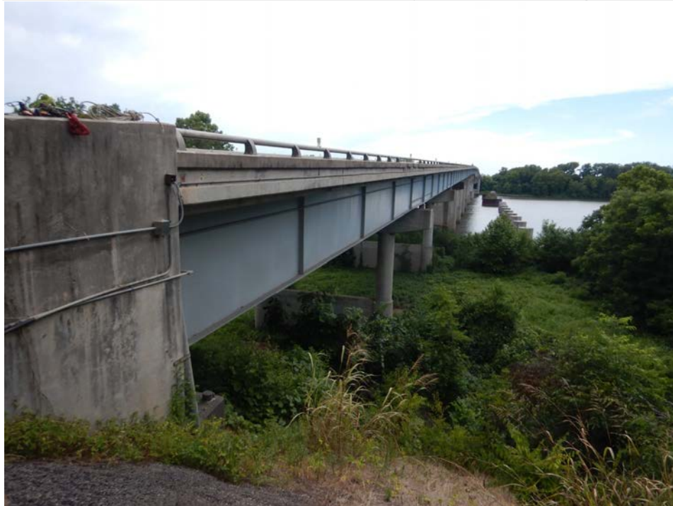
Photograph 2 - Looking southwest at the bridge elevation.
