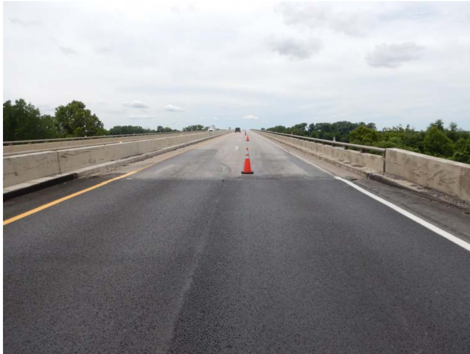
Photograph 1 - Looking west at the bridge end view.
