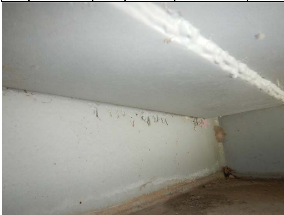
Photograph 54 - Looking southwest at lower lateral bracing gusset plate at girder 1 at floor beam 3 in span 6. Note: gouges exist in the web of the girder.
