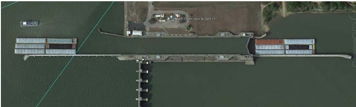
Figure 5.2-5: Hopper Barge Tow at Robert S Kerr Lock and Dam 15
