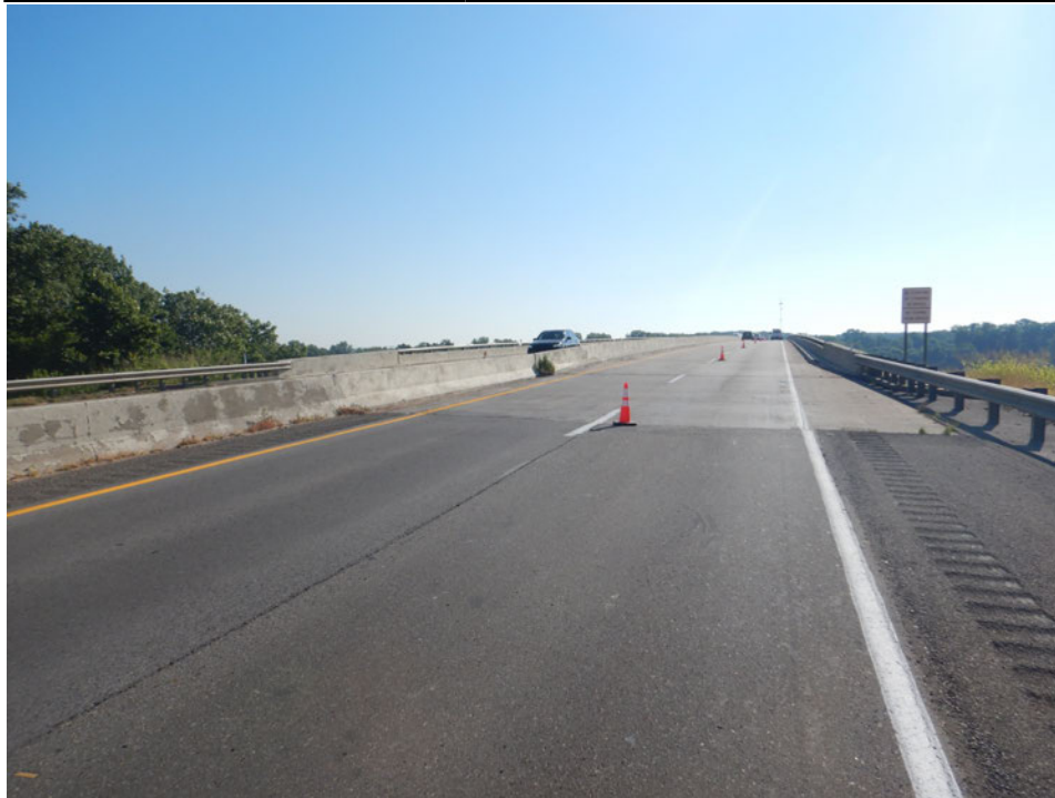
Photograph 1 - Looking east at the bridge end view.
