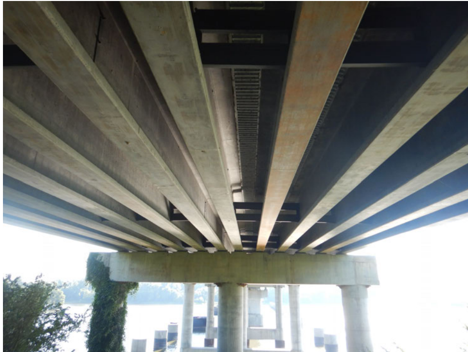
Photograph 21 - Looking east at the underside of span 1. Note: no significant deficiencies.
