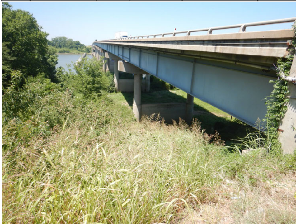
Photograph 2 - Looking west at the bridge elevation.
