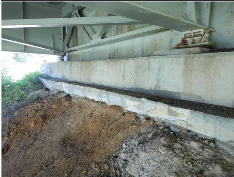
Photograph 52 - Looking northeast at the east abutment. Note: no significant deficiencies.
