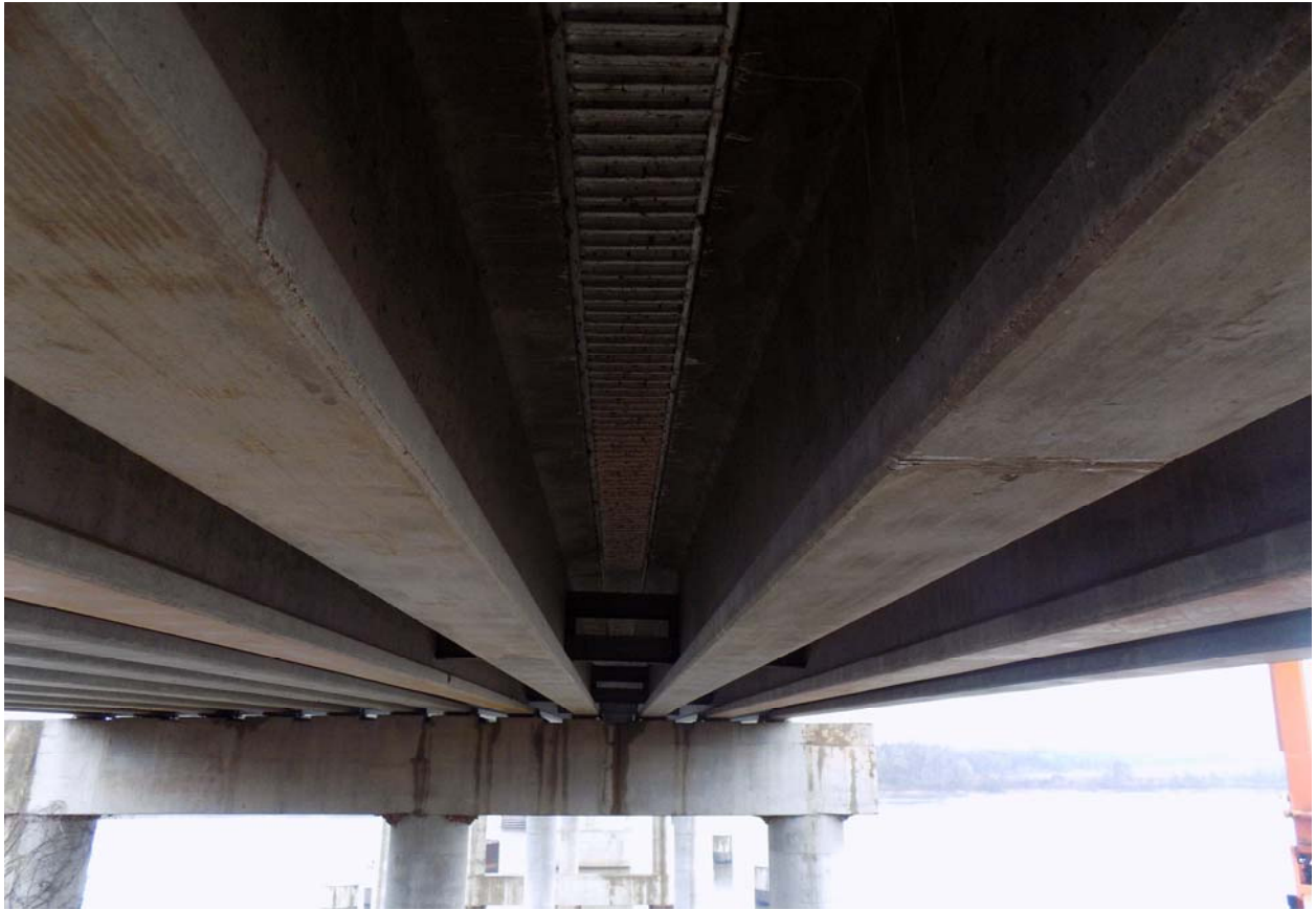
P.C Beams (Typical)
