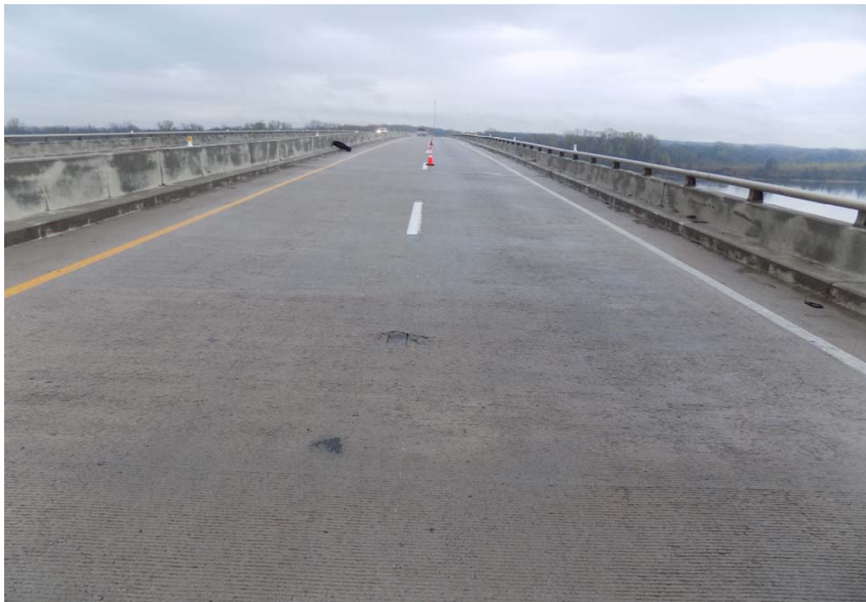
Eastbound Deck Slab, Median Barrier and Parapet
