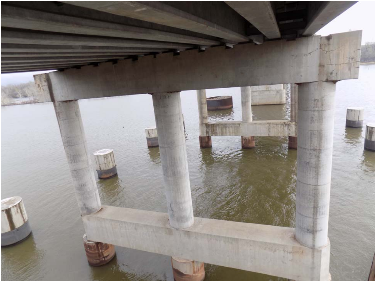
West Side of Pier No. 2
