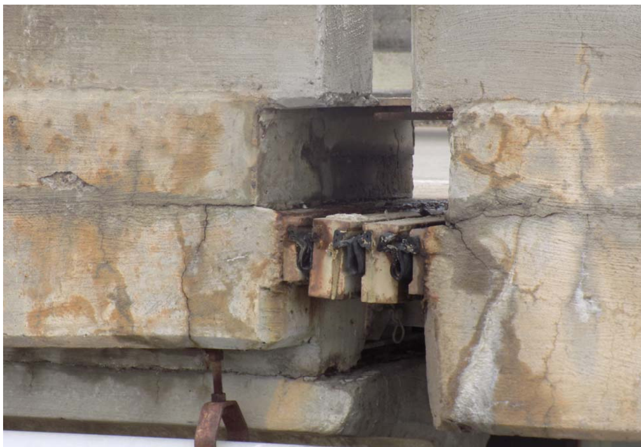
Deck Slab Fascia at Modular Expansion Joint
