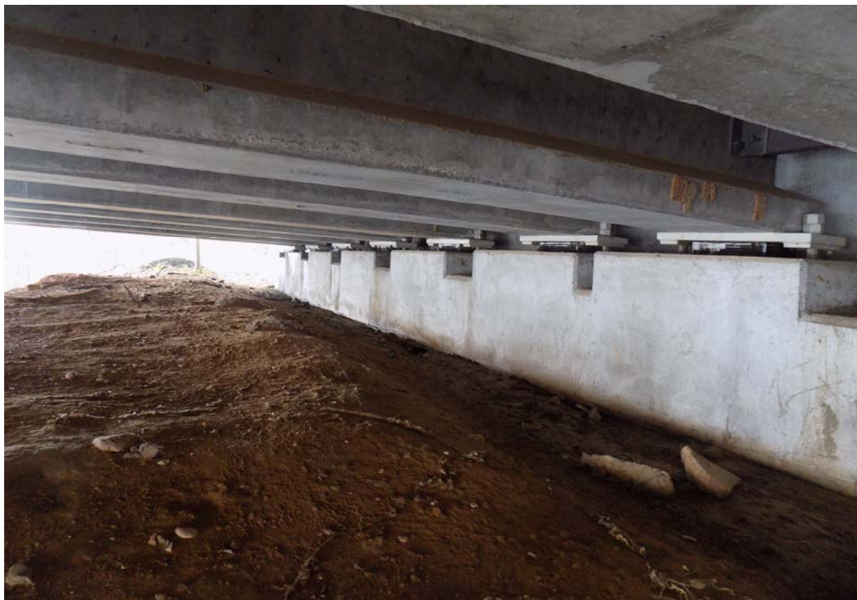
Bridge Seat of Abutment No. 1
