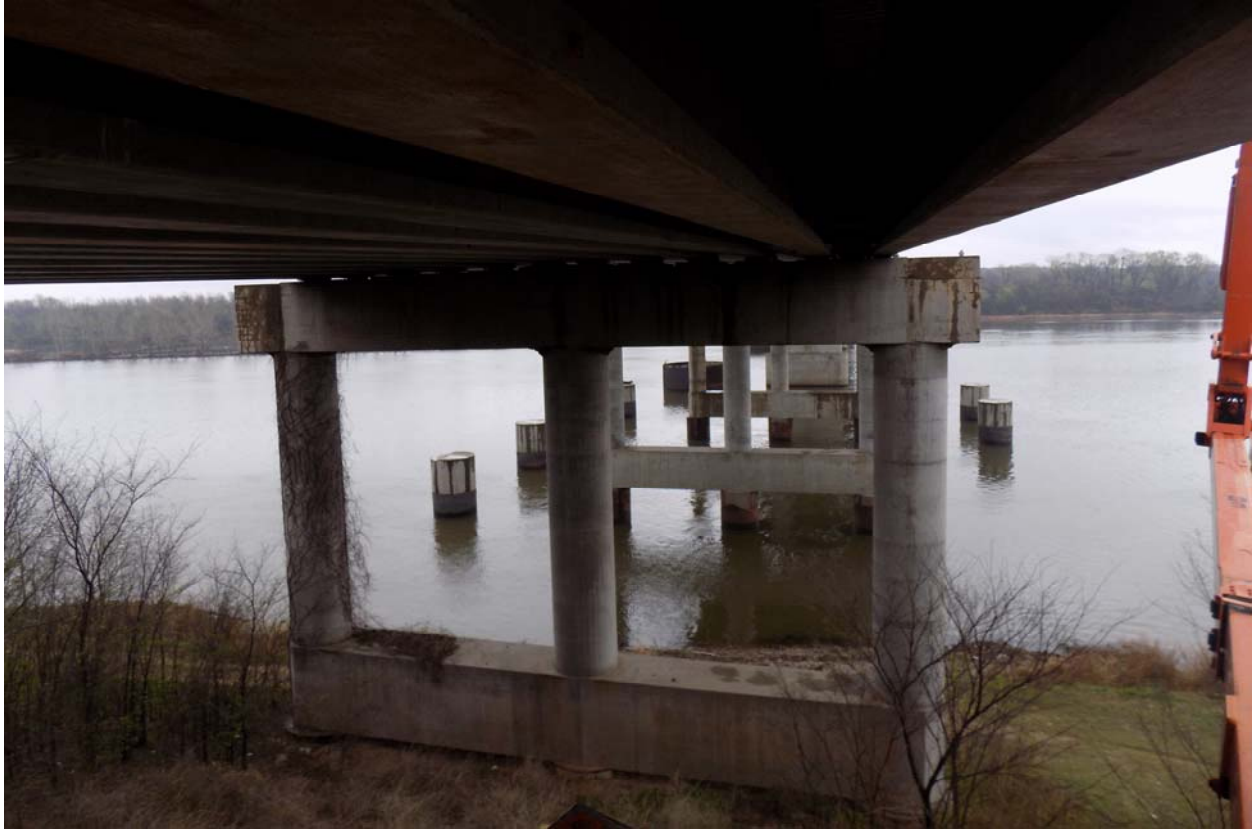
West Side of Pier No. 1
