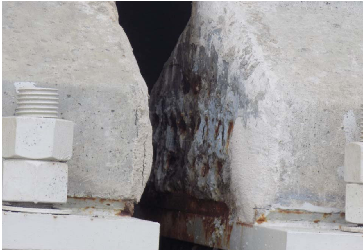
North Exterior P.C. Beam End at Pier No. 2
