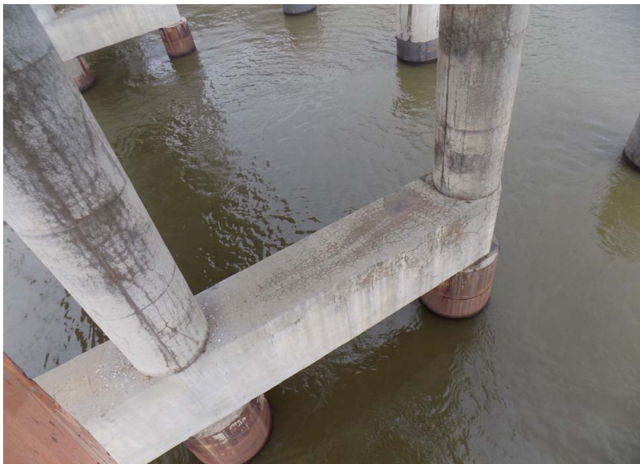
Web Wall at Pier No. 3
