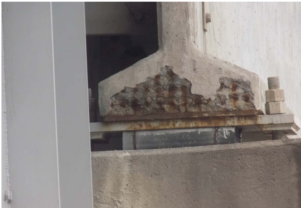
North Exterior P.C. Beam End at Pier No. 3
