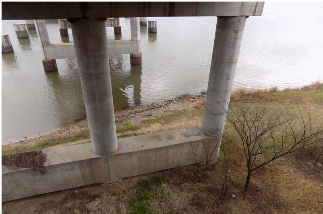
Web Wall at Pier No. 1
