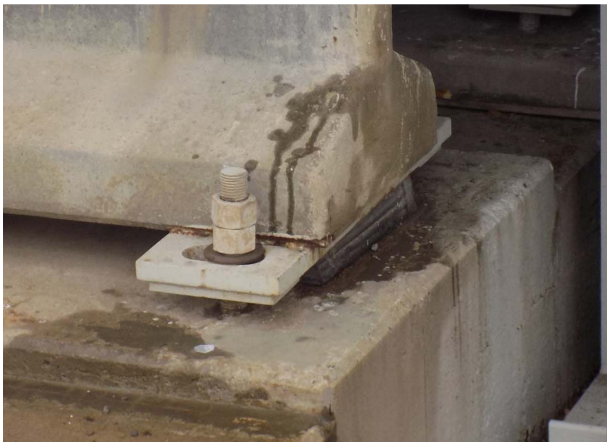
Painted Weathering Steel Bearing Assembly at Exterior P.C. Beam
