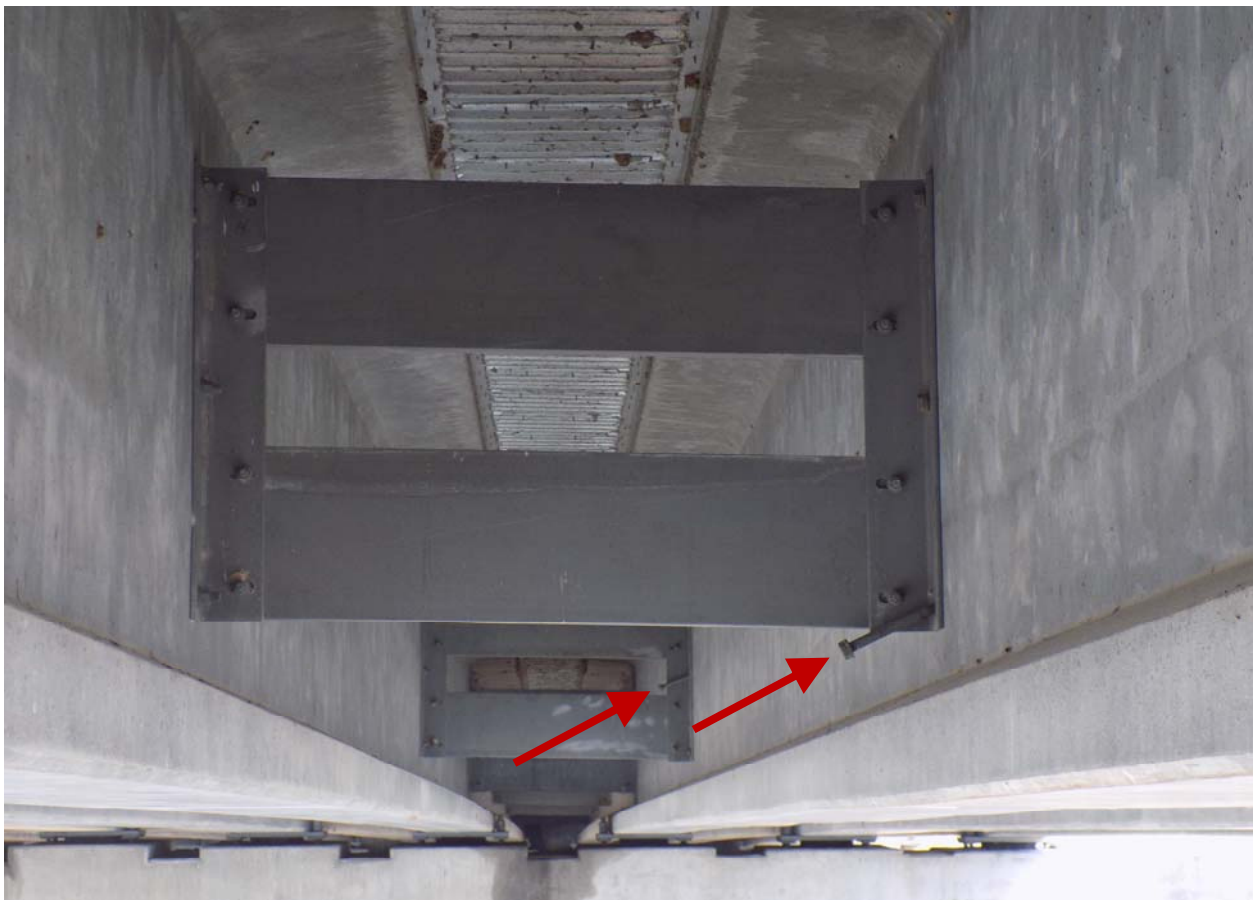
Structural Steel Diaphragms and Angle Gussets (Typical)
