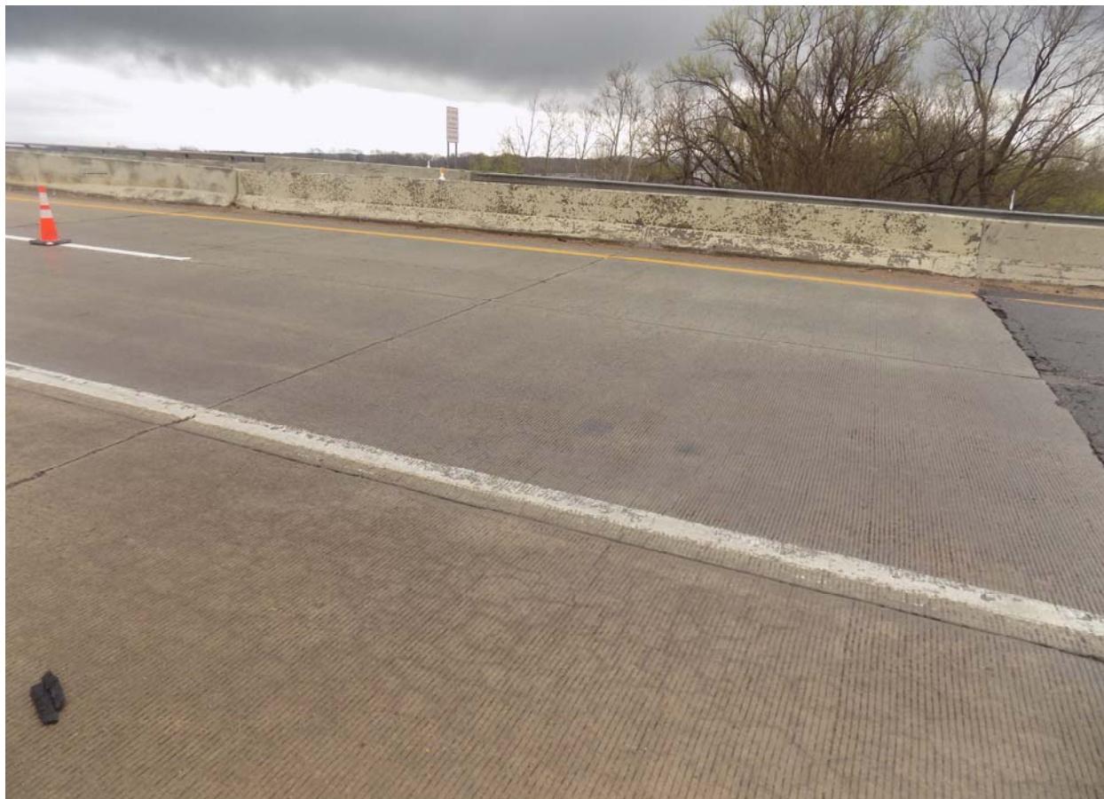
West Approach Slab on Westbound Side of Bridge
