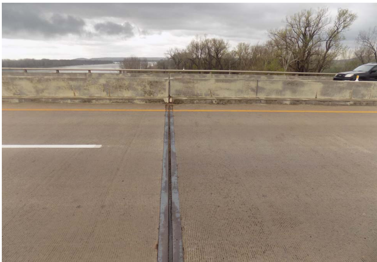
Sealed Expansion Joint in Deck Slab
