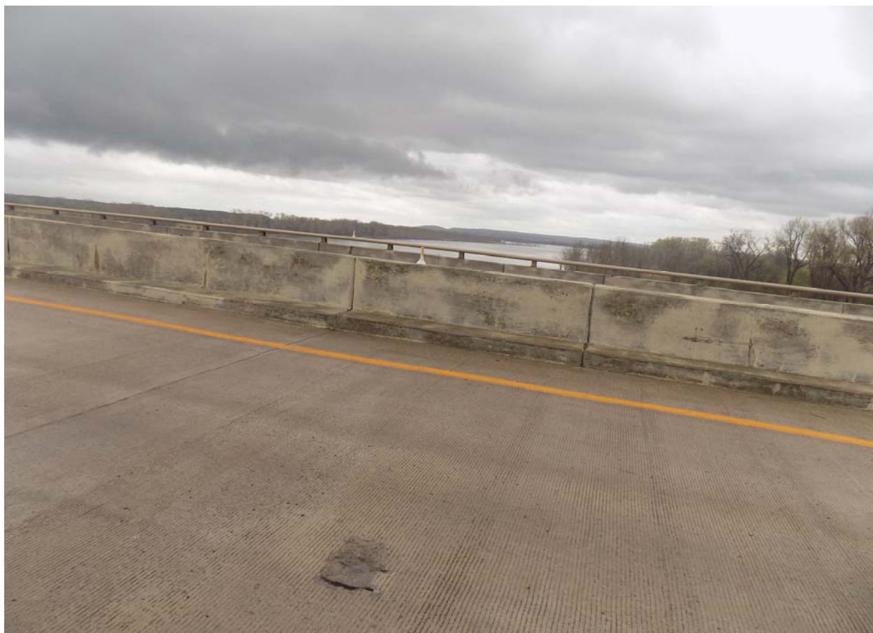
Westbound Deck Slab and Median Barrier
