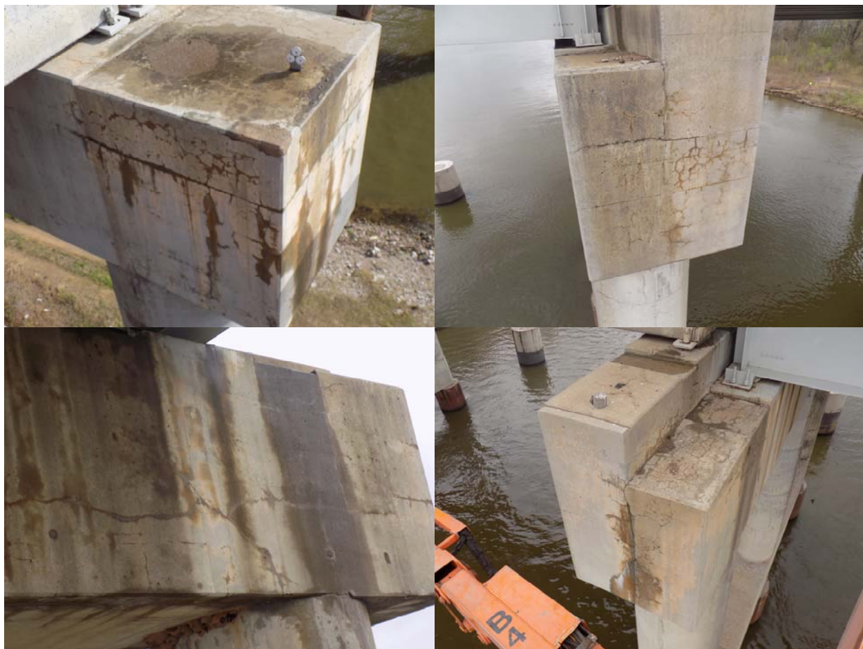
Pier Cap Overhangs
