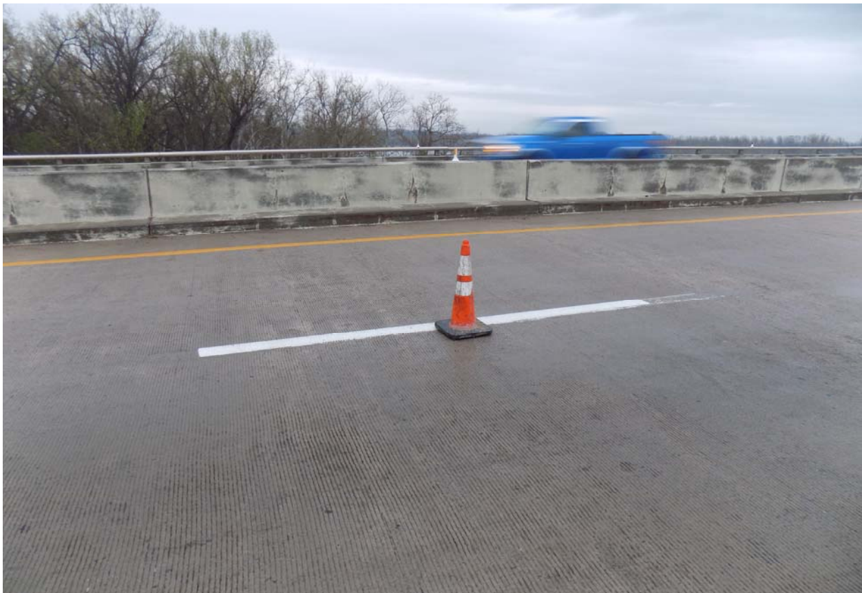
Eastbound Deck Slab and Median Barrier
