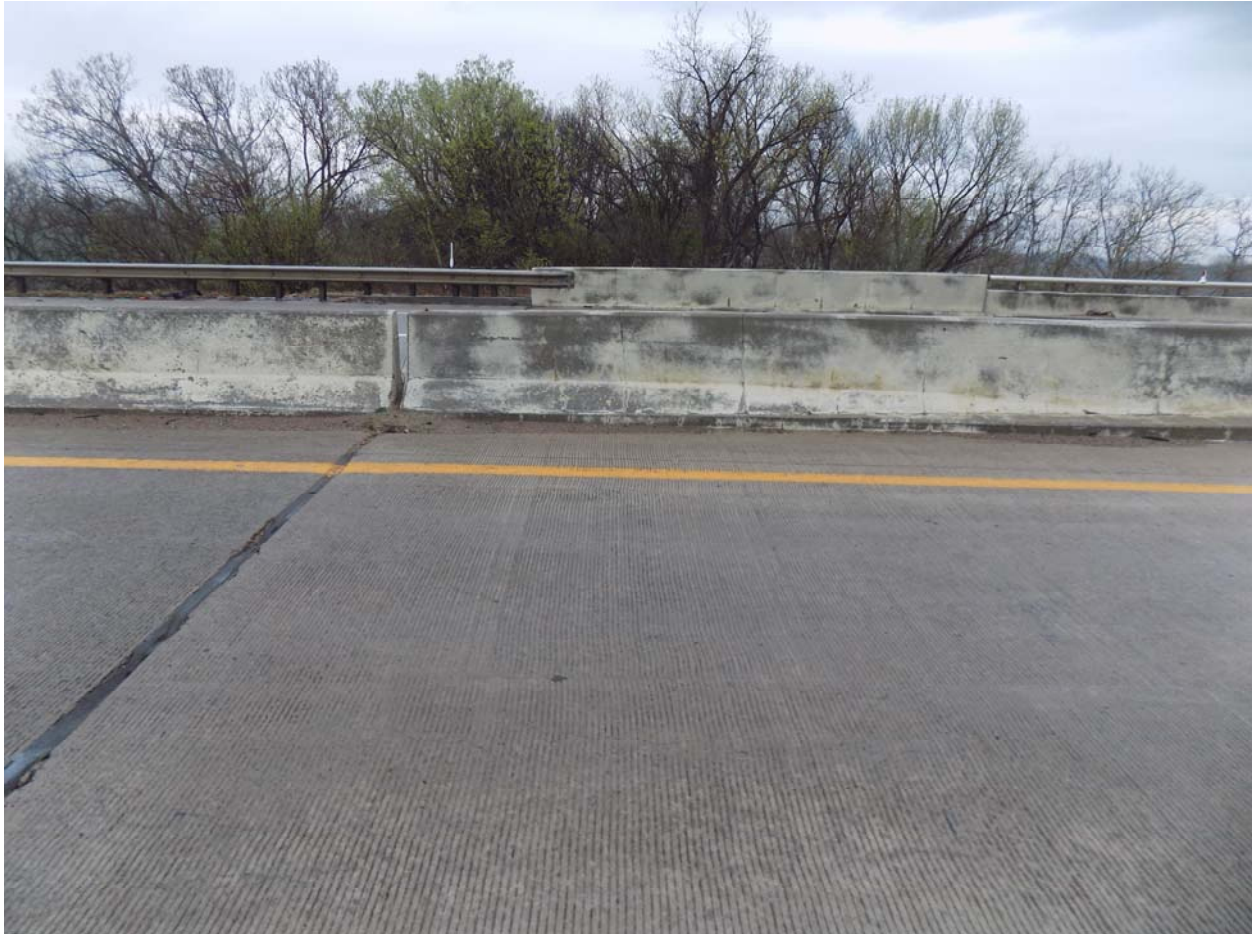
West Approach Slab on Eastbound Side of Bridge
