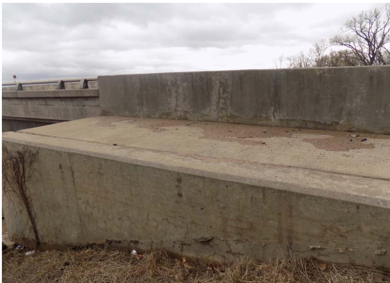
North Wing of Abutment No. 1
