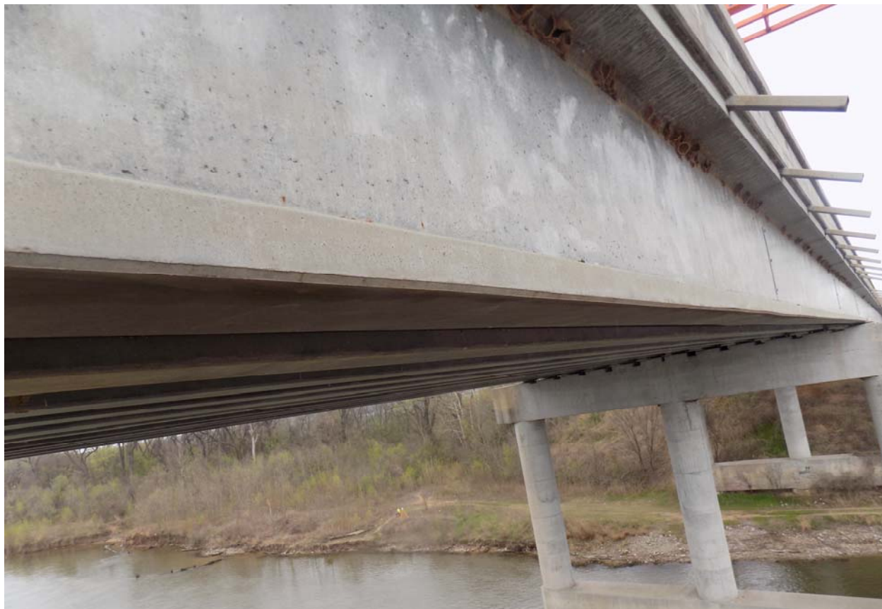
Soffit of Eastbound Deck Slab
