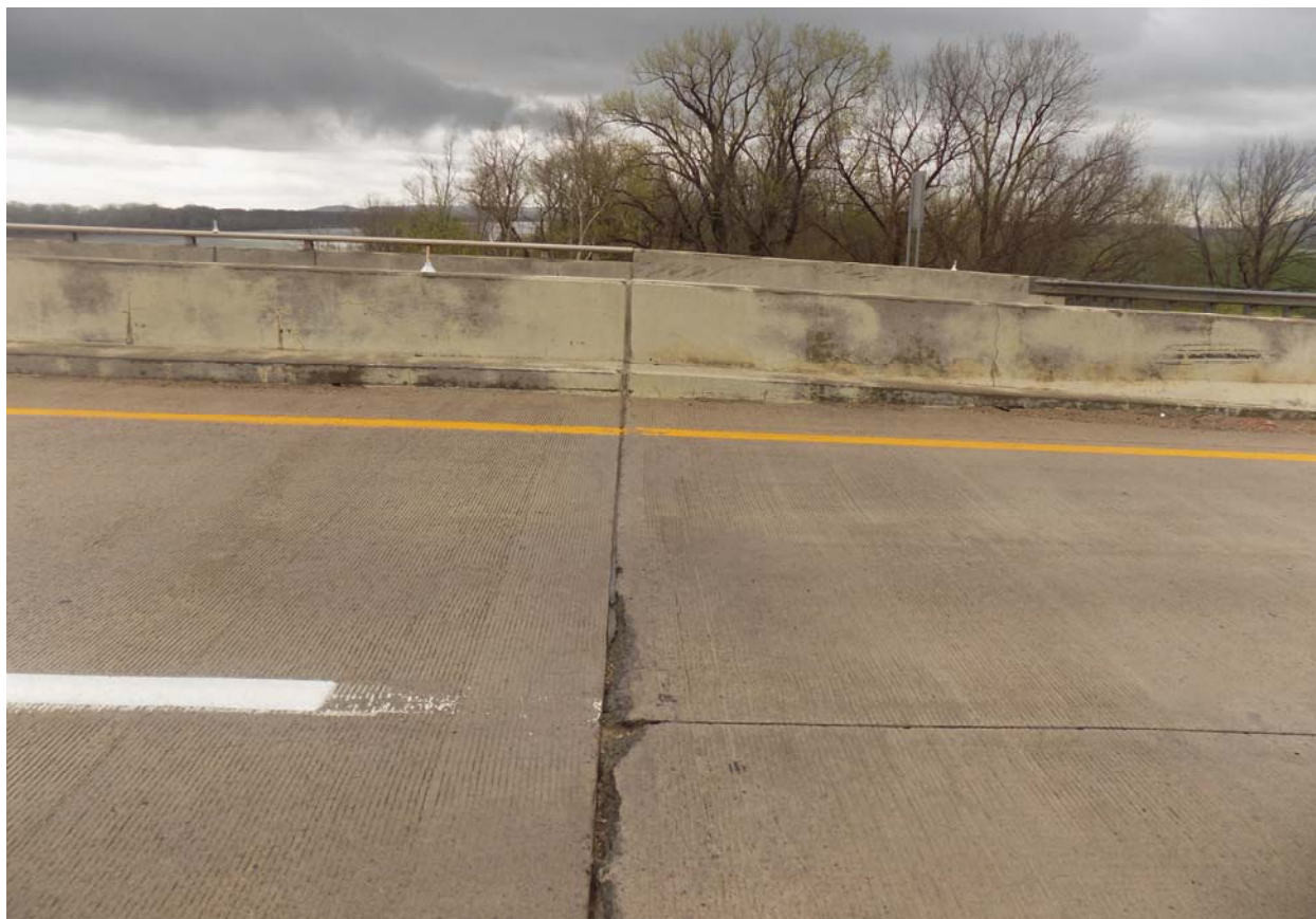
Construction Joint between Deck Slab Approach Slab
