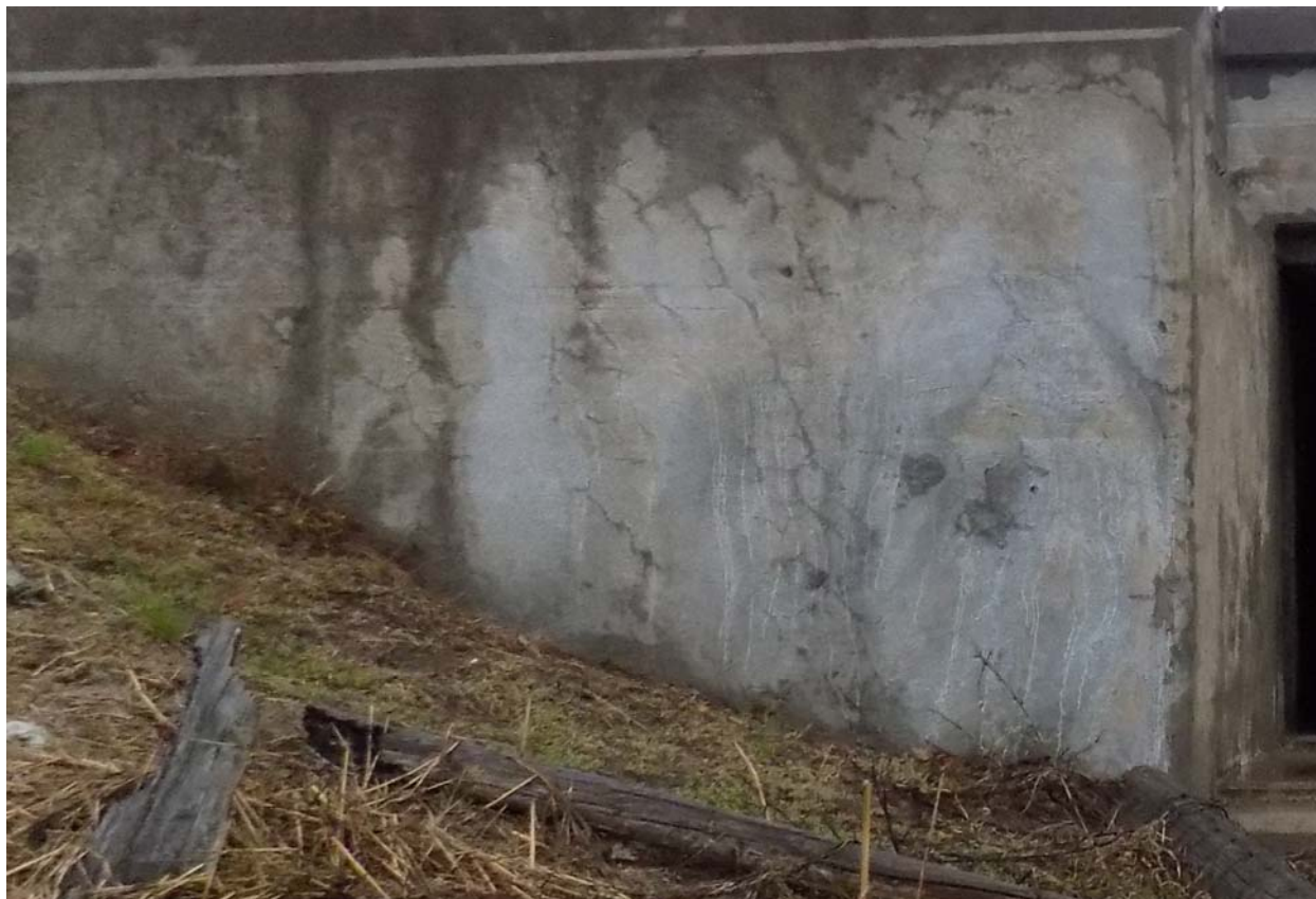
South Wing of Abutment No. 1
