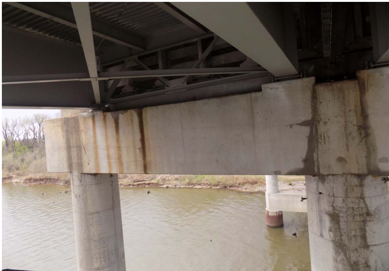
East Side of Pier No. 3
