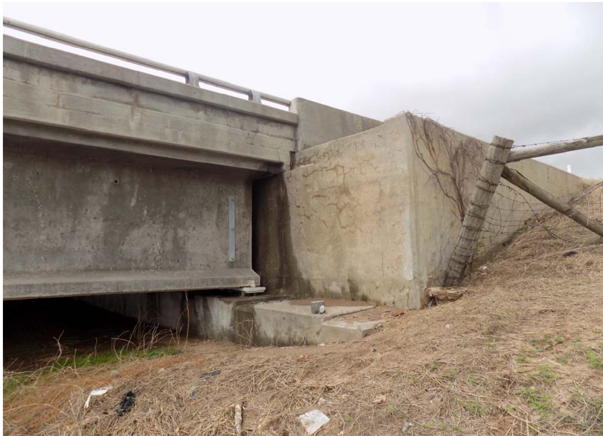
North End of Abutment No. 1
