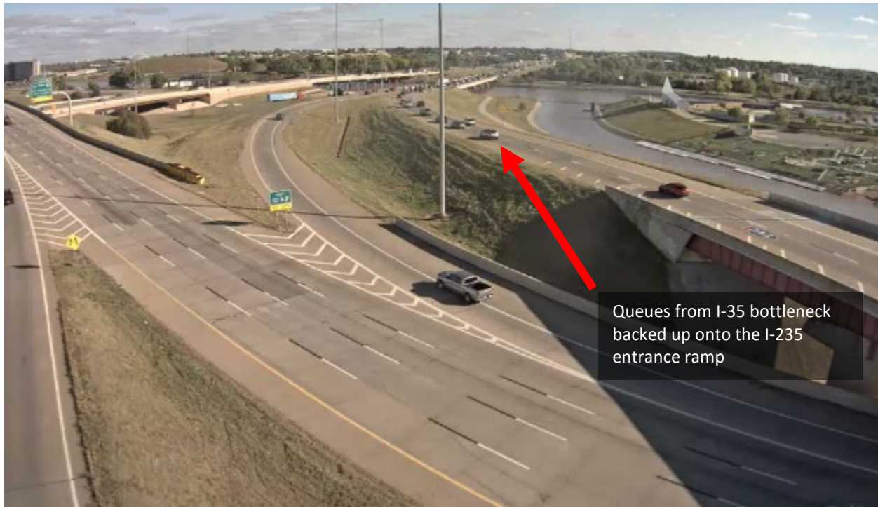
Figure 9. Queues from I-35 spilling over to I-40 entrance ramps and I-235, November 5, 2024, at 3:17pm
