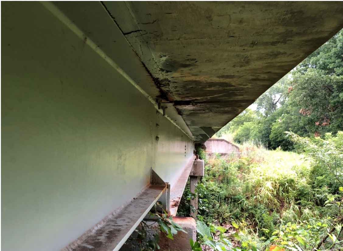
Fig. 4: Underside of Soffit and Scuppers (Typical)
