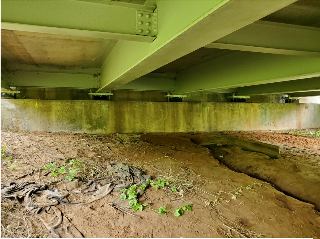
Fig. 10b: Front Face of Abutment Seat (Abutment 1, Facing West)
